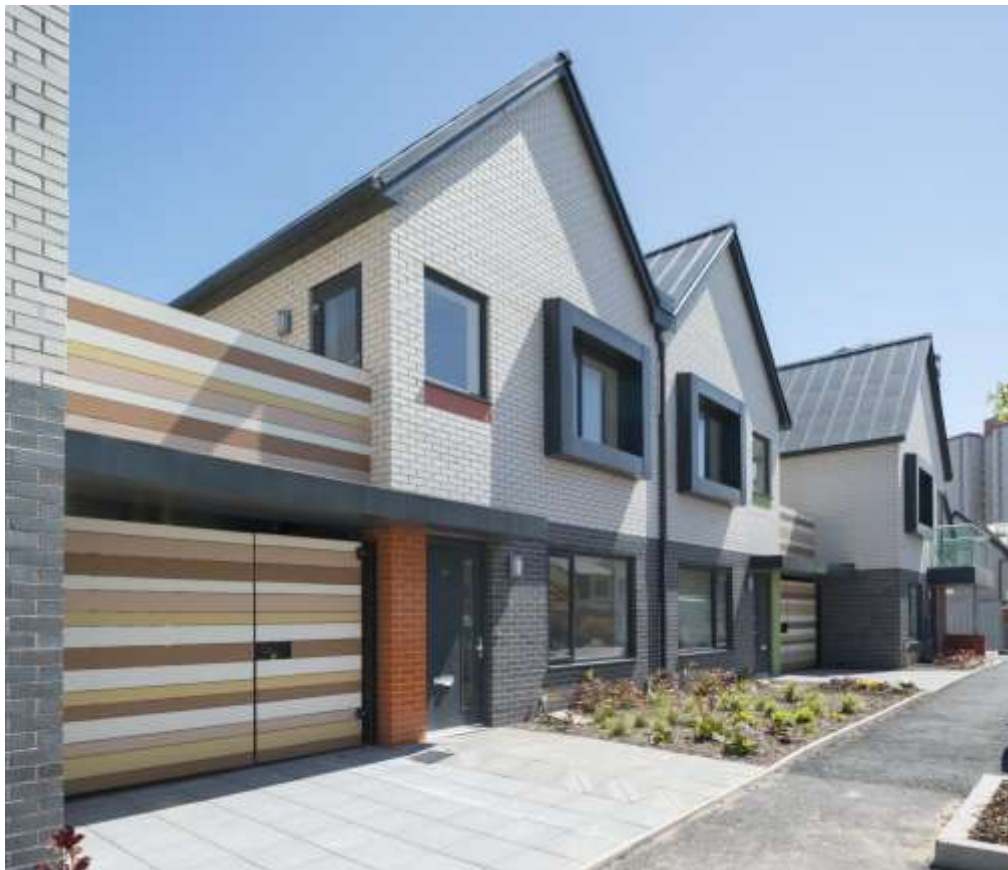
Above: Affordable housing at Queens Park, Blackpool
