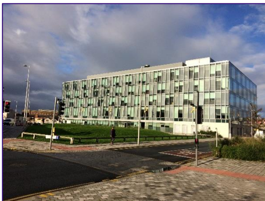
Photograph 7: Blackpool Borough Council Offices, George Street
