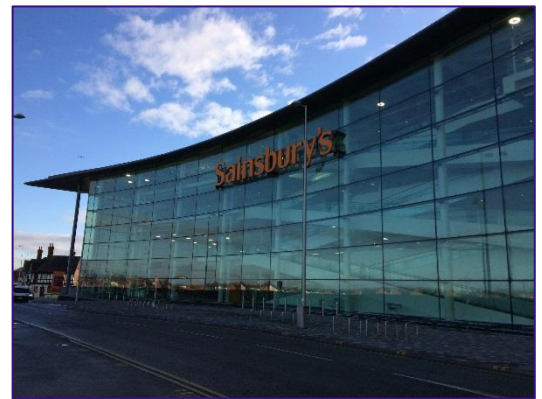
Photograph 6: Sainsbury's Supermarket, Talbot Road
