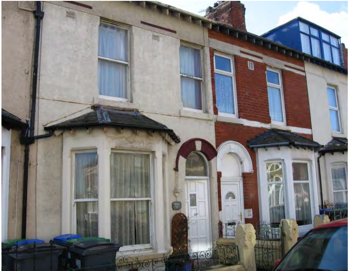
Fig.19: The contrast between rendered brick frontages and an original fair-faced brick frontage on Lowrey Terrace
