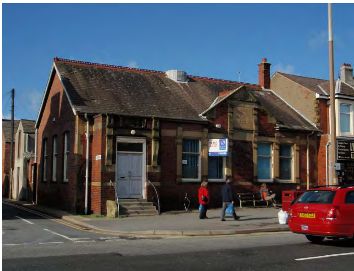
Fig.52: The former library on Lytham Road has Local List potential
