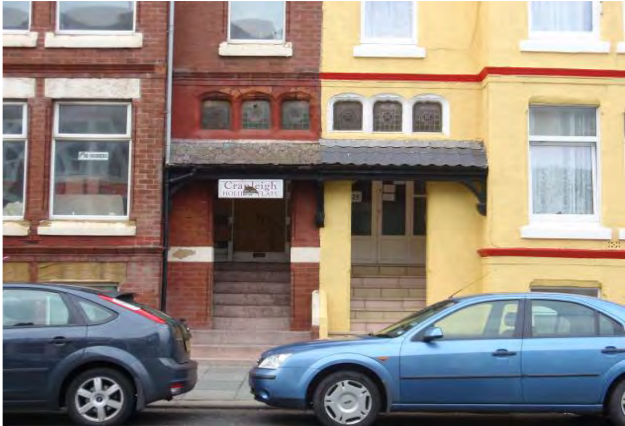
Fig.20: Nos 25 & 27 Tyldesley Road; historic sashes survive to the right with uPVC to the left.
