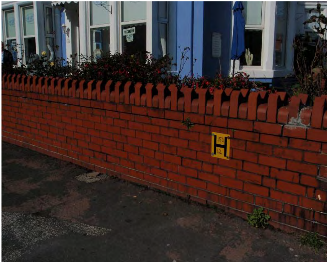
Fig.23: Early 20 th century brick boundary walls on Alexandra Road with decorative brick coping
