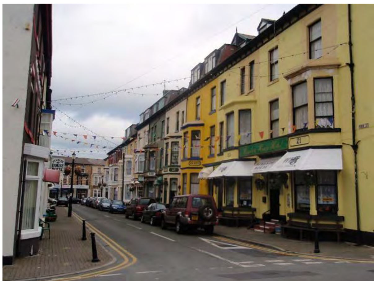
Fig. 49: York Street looking west
