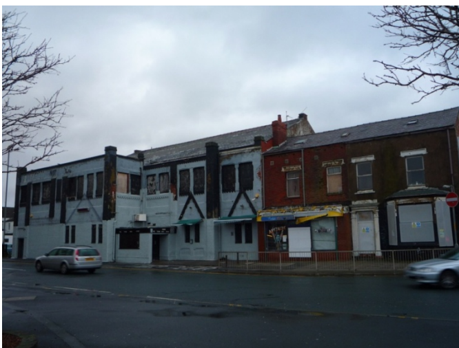
Figure 62: Derelict Rock Club on Cookson Street
