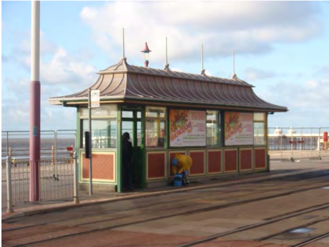
Fig. 41: Tram shelter near the Tower
