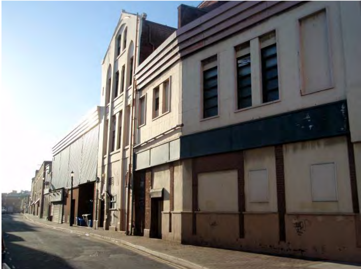
Fig. 57: Looking south along the east side of Foxhall Road from Chapel Street
