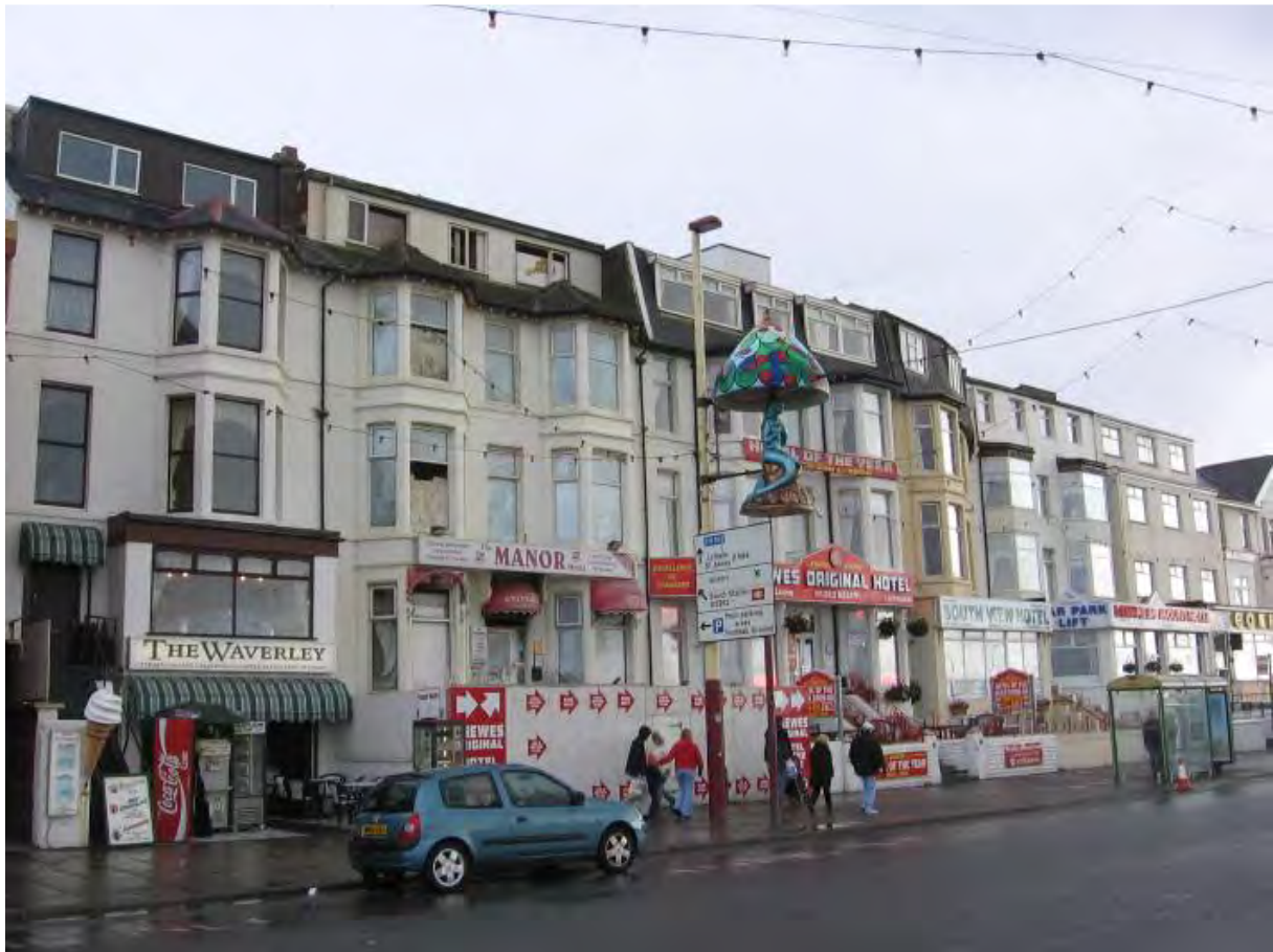
Fig. 45: Boarding houses on the Promenade
