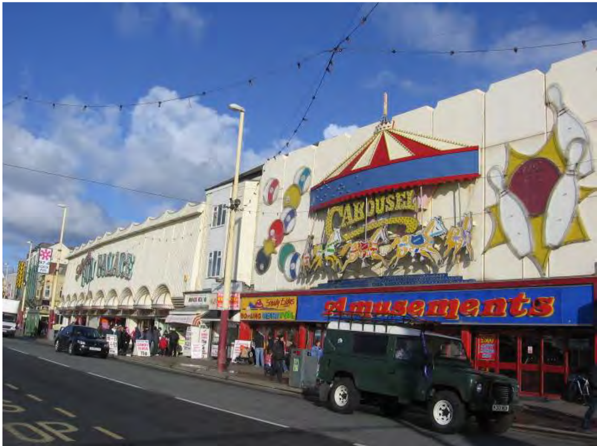
Fig. 47: Entertainment buildings south of the Tower
