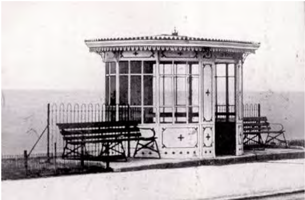
Fig. 40: Tram shelter at South Beach, early 20 th -century (Image from www.rossallbeach.co.uk )
