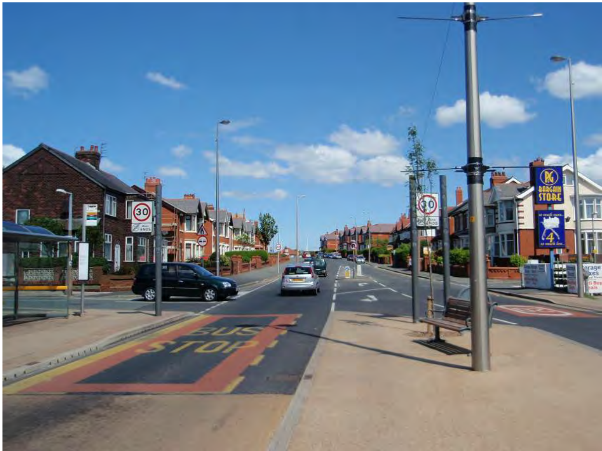
Fig. 114: Looking north up Westcliffe Drive from outside the Institute
