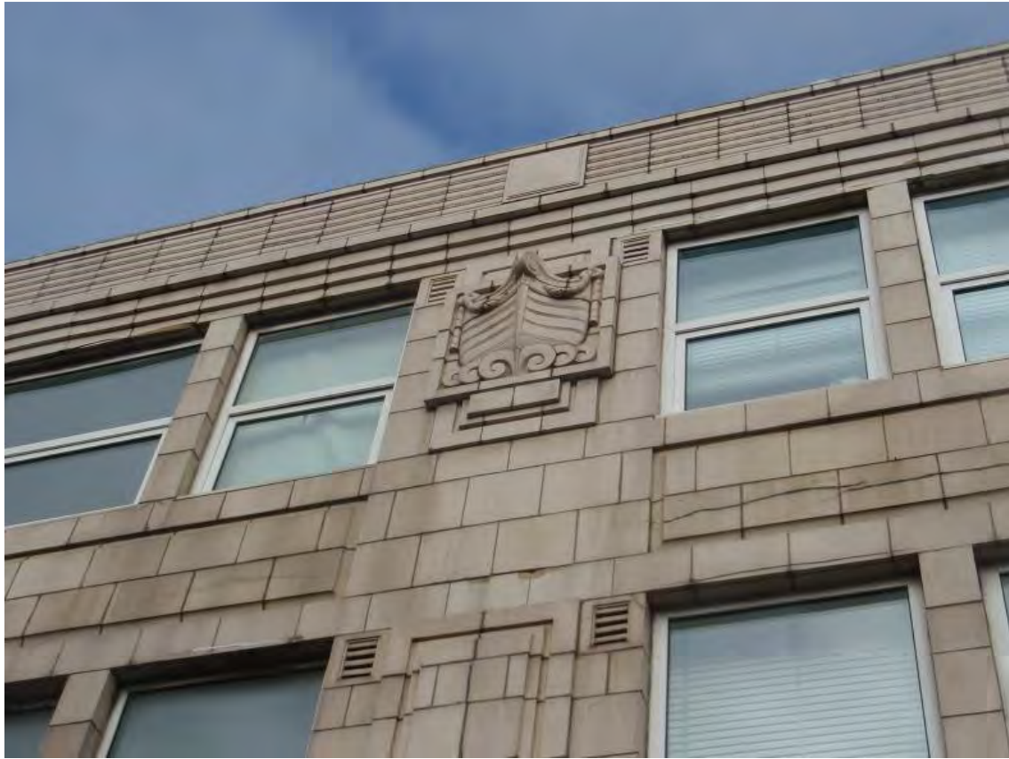
Fig. 26: Terracotta faience decoration on Church Street
