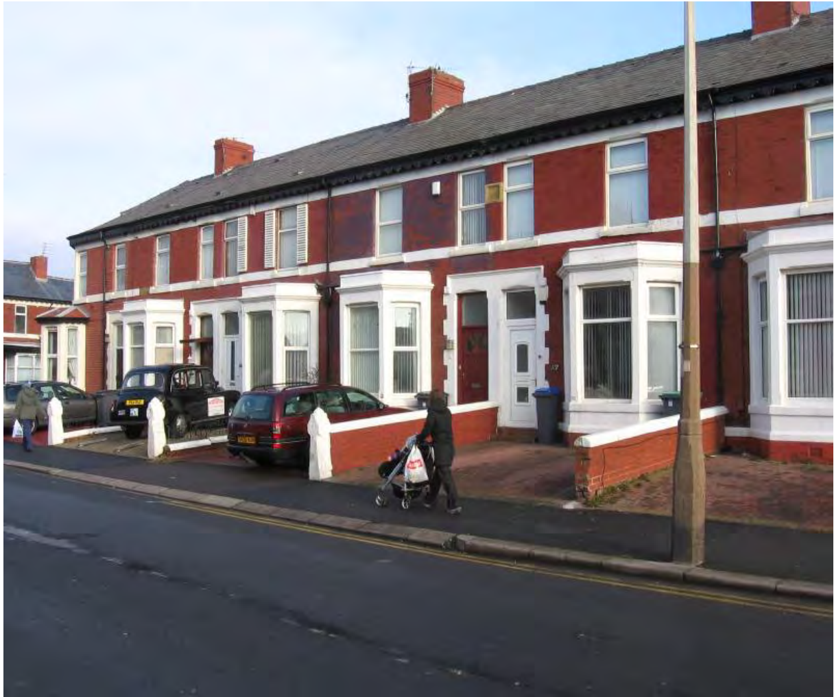
Fig.43: Frontage car parking towards the south end of Egerton Road
