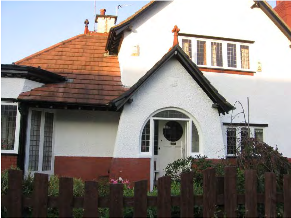
Fig. 56: No. 2a Mere Avenue: detail showing treatment of porch, rooflines and windows.
