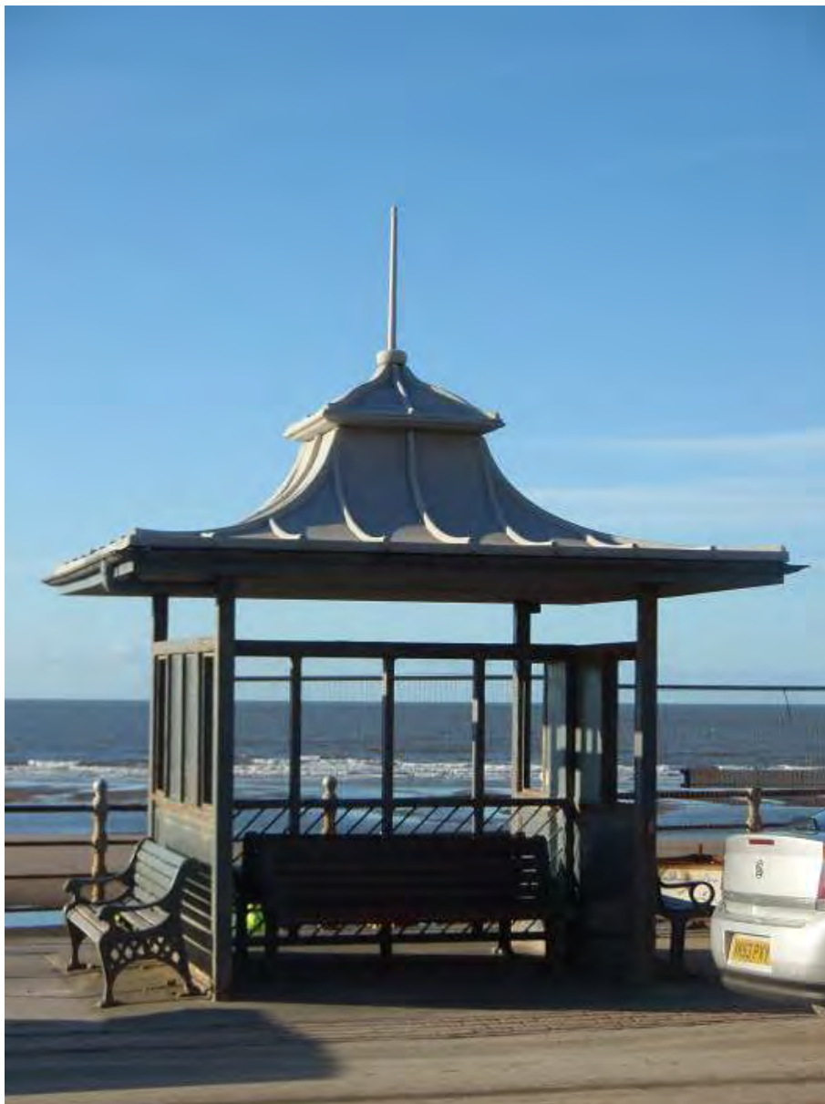
Fig. 43: Replica Promenade shelter
