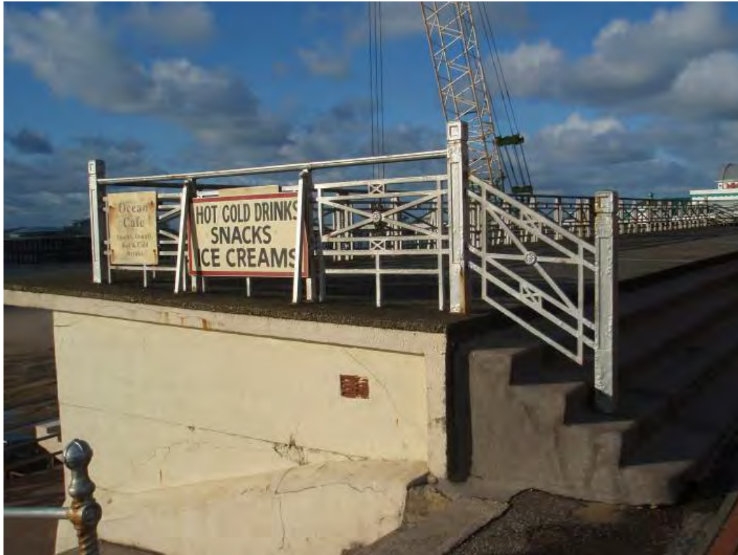
Fig. 32: 1920s steel balustrading near North Pier
