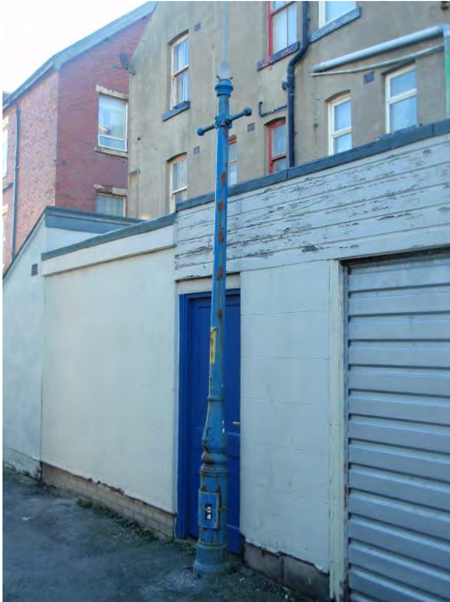
Fig. 32: Redundant gas standard on a back street
