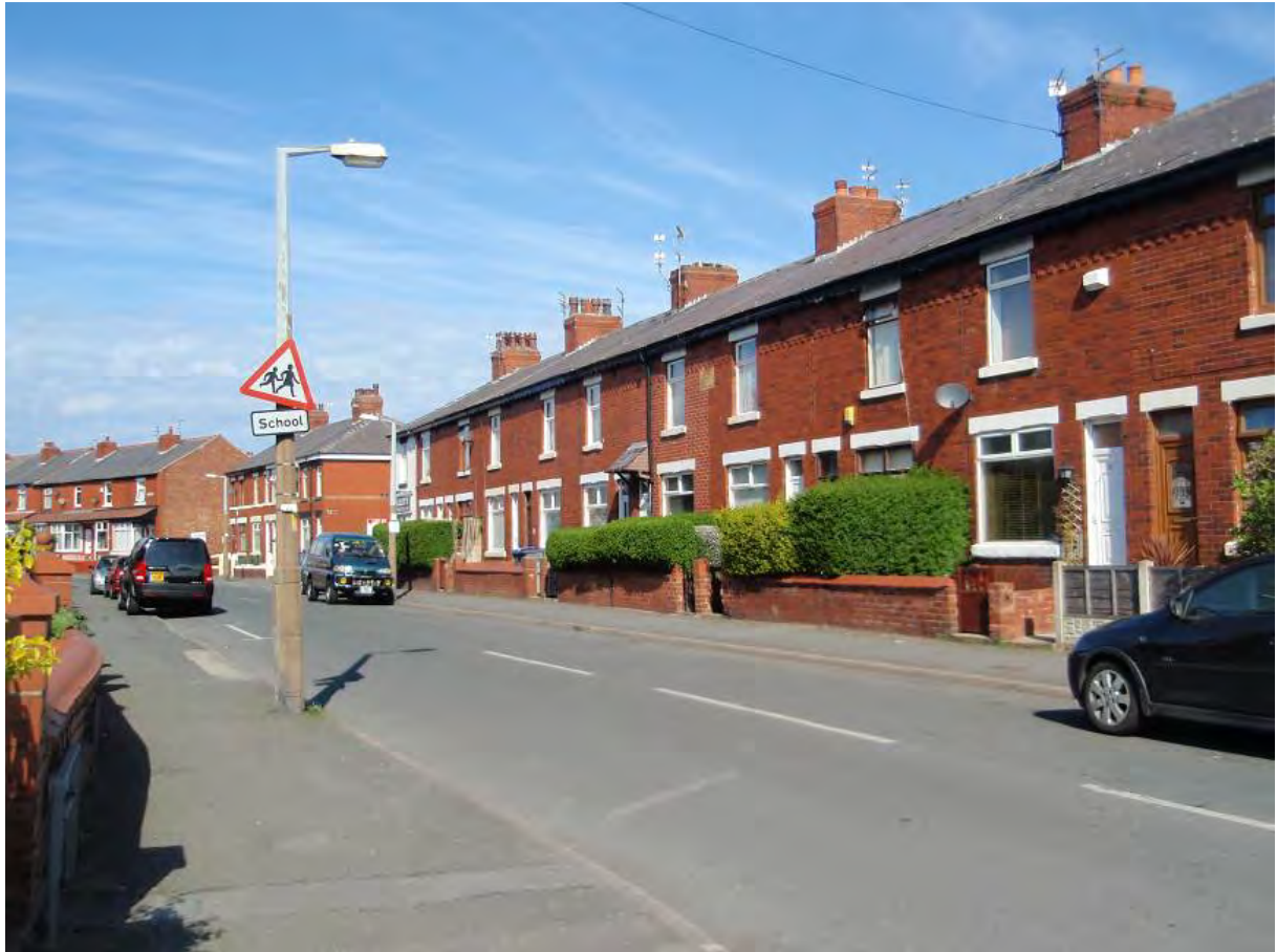
Fig. 101: Nos 77 101 Onslow Road, on the north side
