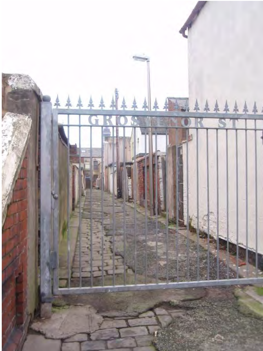
Fig. 32: Modern steel security gate off Grosvenor Street
