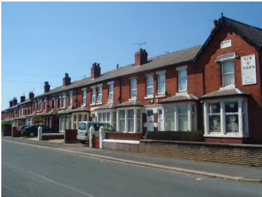
Fig. 129: Nos 42-74 Layton Road from the south
