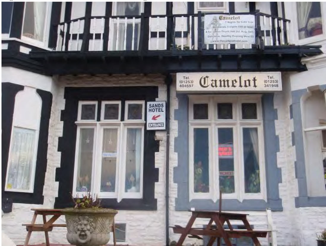
Fig. 21: Ground floor windows to No.487 Promenade
