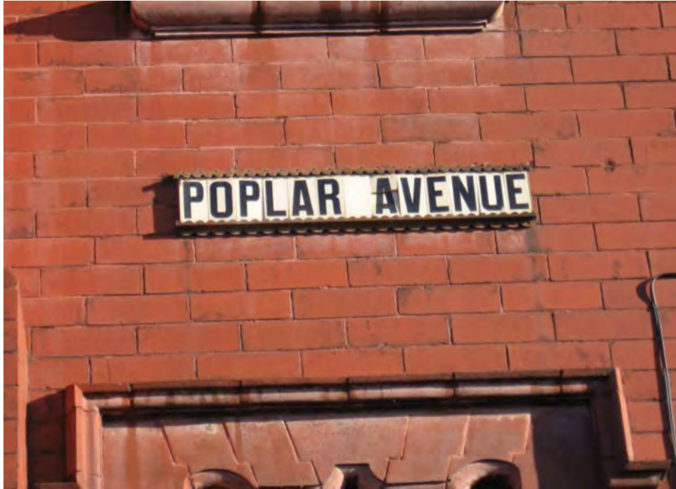
Fig. 41: Early 20 th -century street name signage, tiled letters in cast-iron frame
