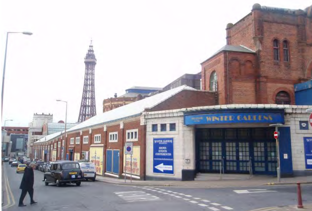
Fig. 89: The south elevation of the Winter Gardens, from the east
