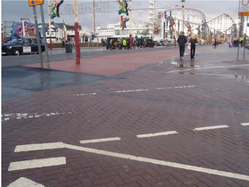
Fig. 29: Surfacing to the Promenade near South Pier
