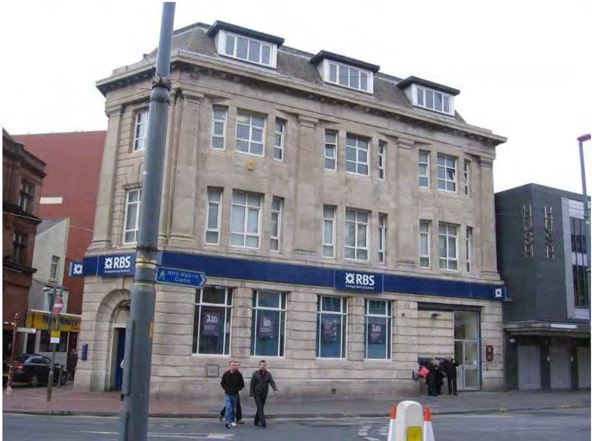
Fig. 72: The RBS building on Talbot Road
