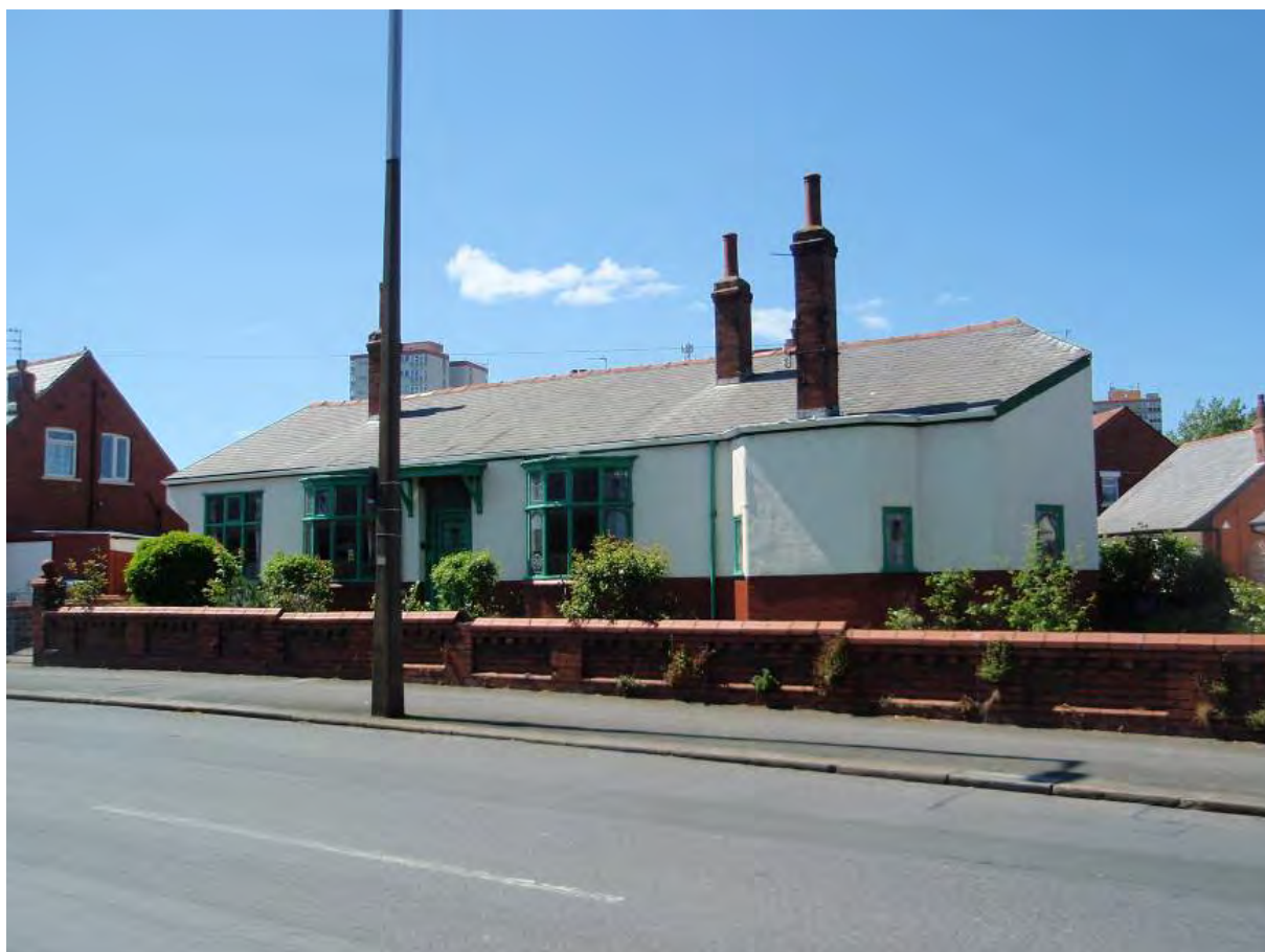
Fig. 112: No. 2 Layton Road
