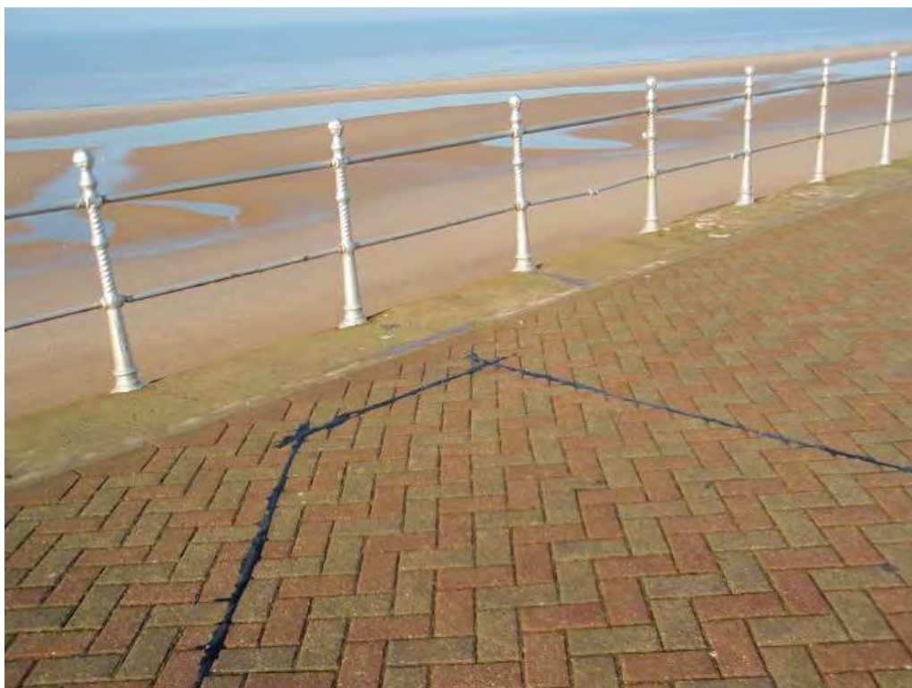
Fig. 24: Balustrades to lower walkway
