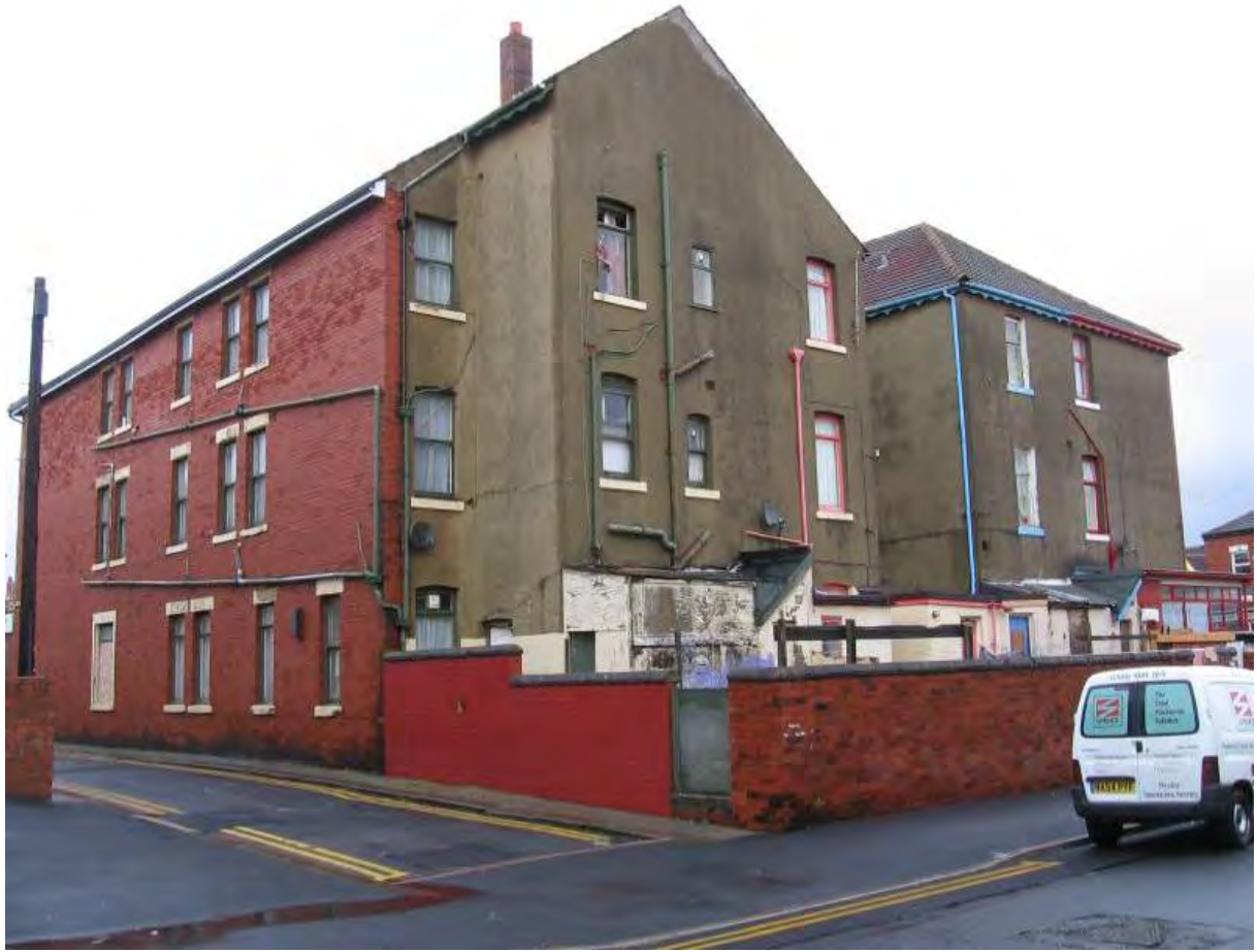
Fig.36: Typical large outriggers on lodging houses fronting Pleasant Street, seen from Mount Street
