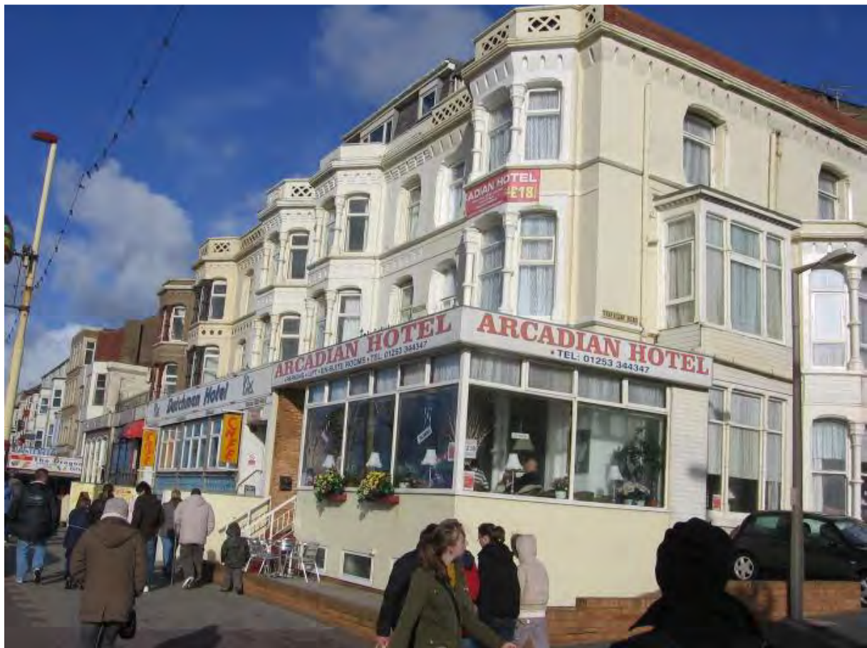
Fig. 48: Ground floor extensions and almost complete upper storeys to Eaves Terrace
