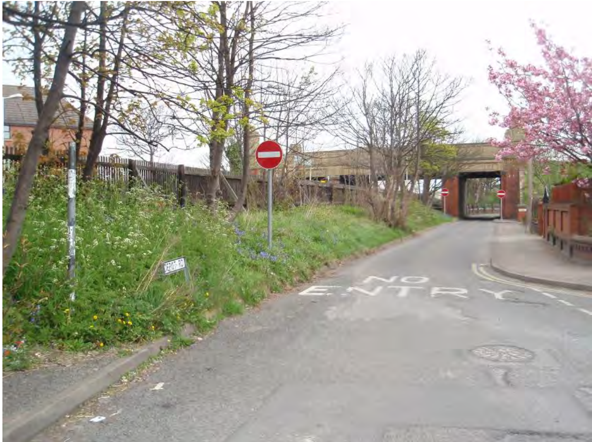
Fig. 76: Looking along Depot Road to Crossley's Bridge
