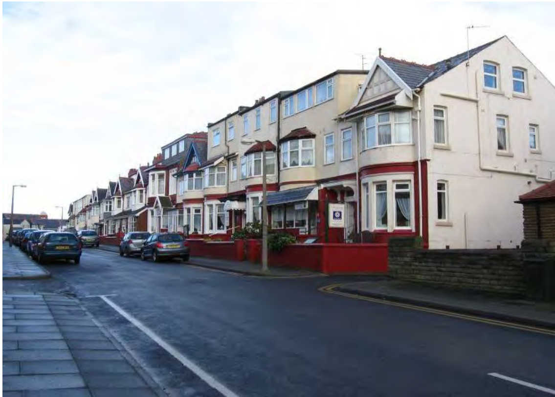
Fig.87: Large early 20 th century houses on Gynn Avenue, now much altered
