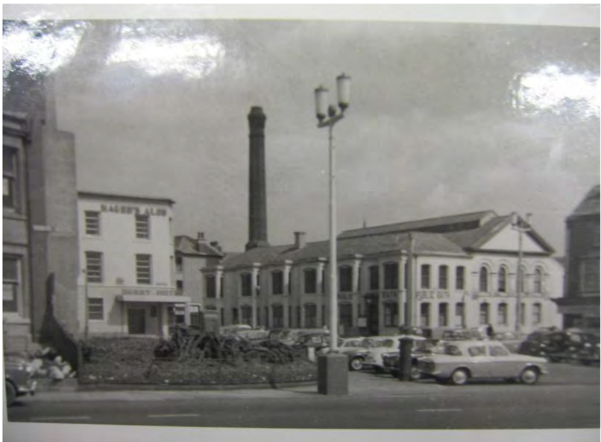
Fig.8: The baths on Cocker Street before demolition in 1974 (Blackpool Library)
