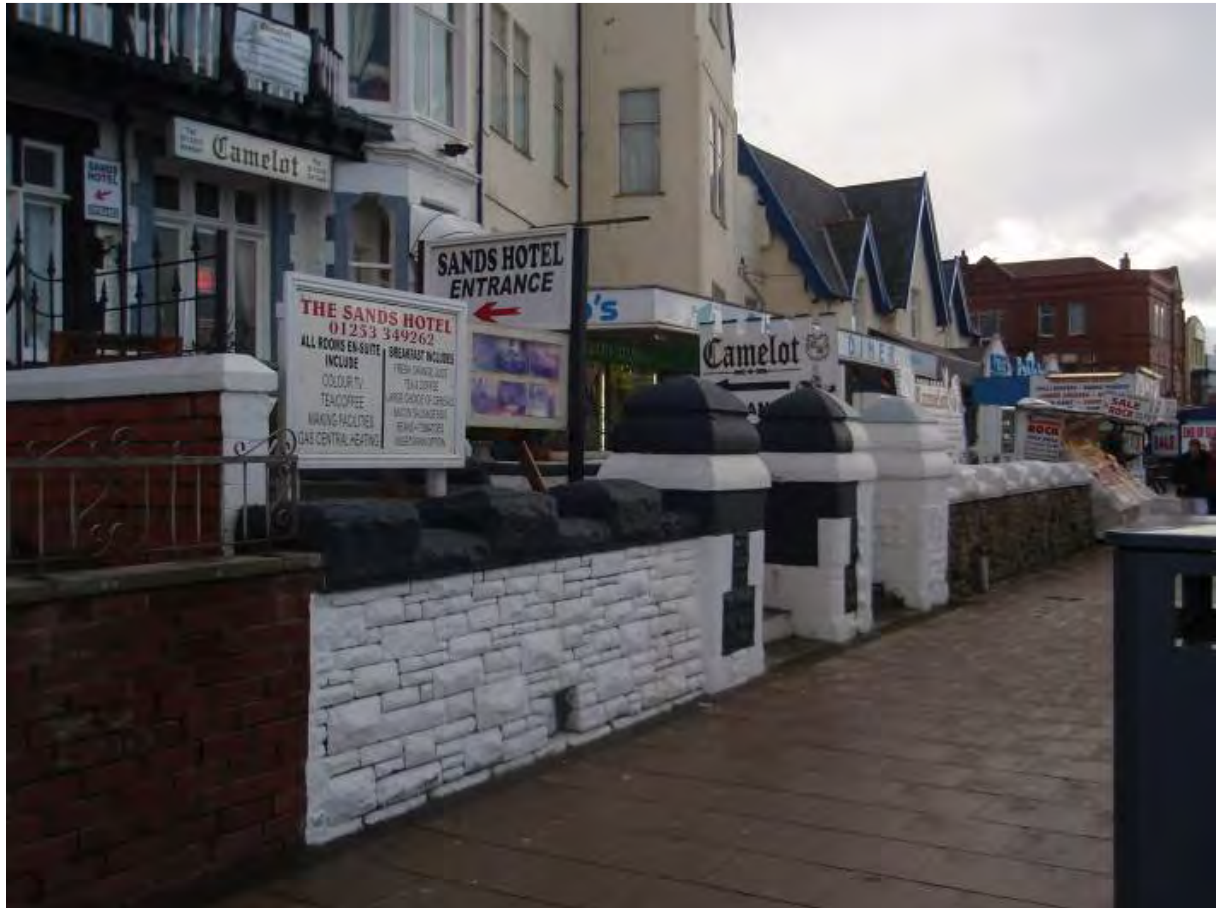
Fig. 28: Original stone boundary wall to back of footway outside the Camelot Hotel
