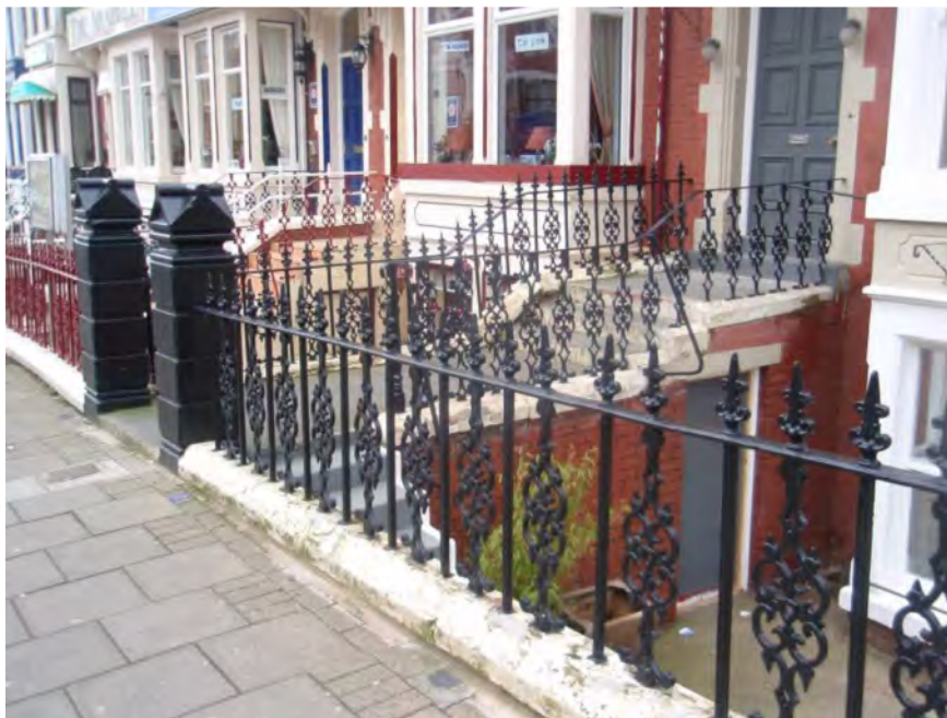
Fig. 31: Cast-iron railings on Albert Road
