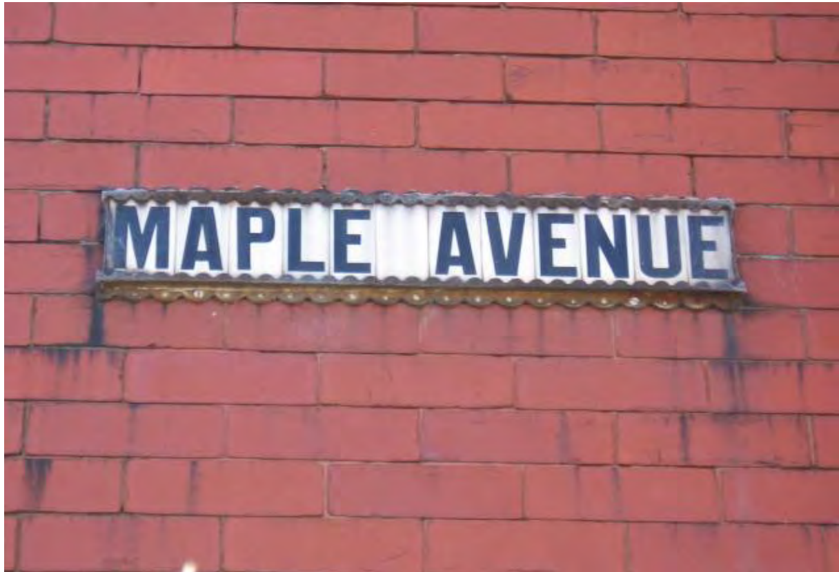
Fig. 102: Typical cast iron and tiled street sign
