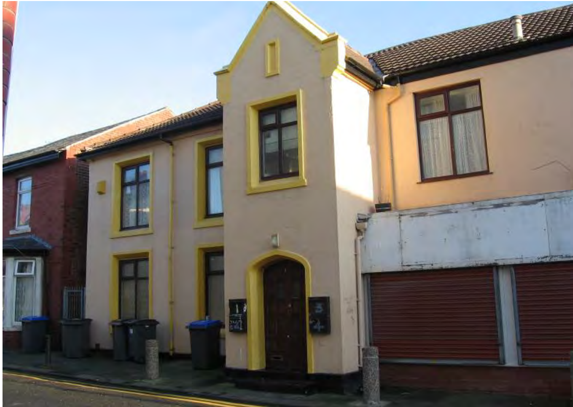
Fig.77: Lynn Grove house, formerly The Cliffe, built c.1860
