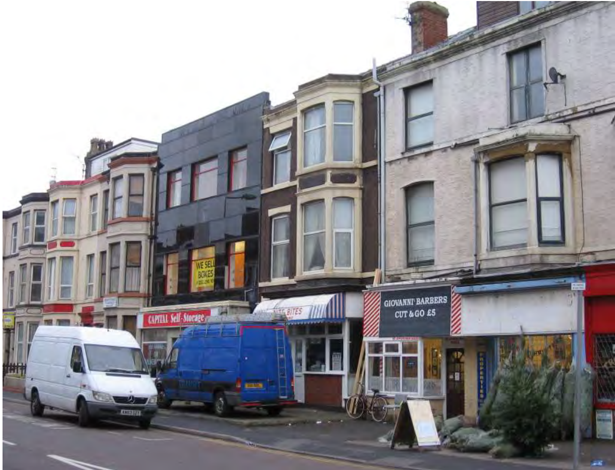
Fig.48: Altered lodging houses on the west side, built in the 1870s.
