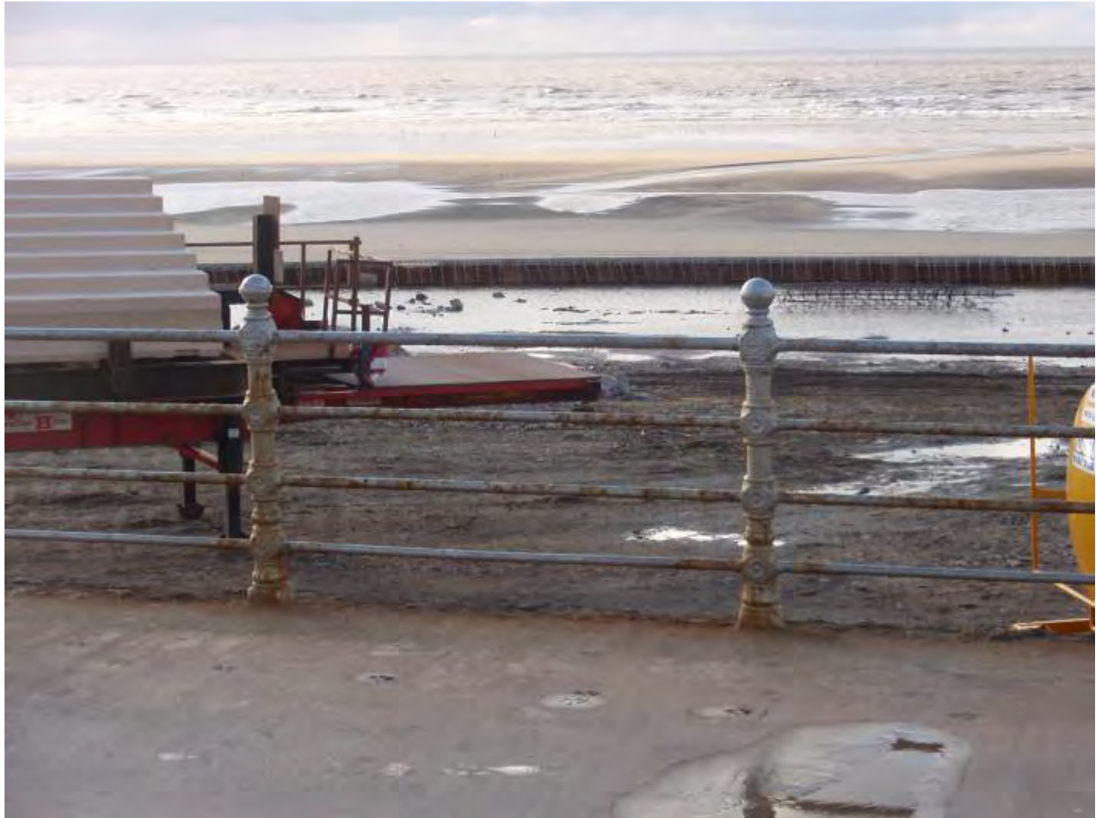
Fig. 31: Late Victorian or Edwardian cast-iron railings on the Promenade
