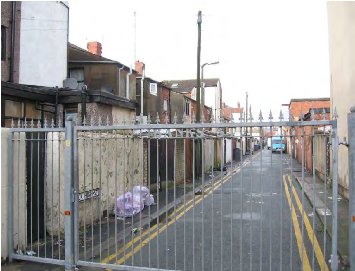
Fig.13: Narrow rear lane and densely developed back yards on Back High Street
