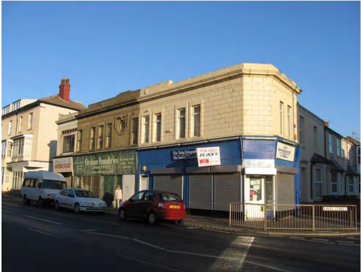
Fig. 39: Nos 169-175 Dickson Road, a 1920s commercial buildings faced in faience in classical style
