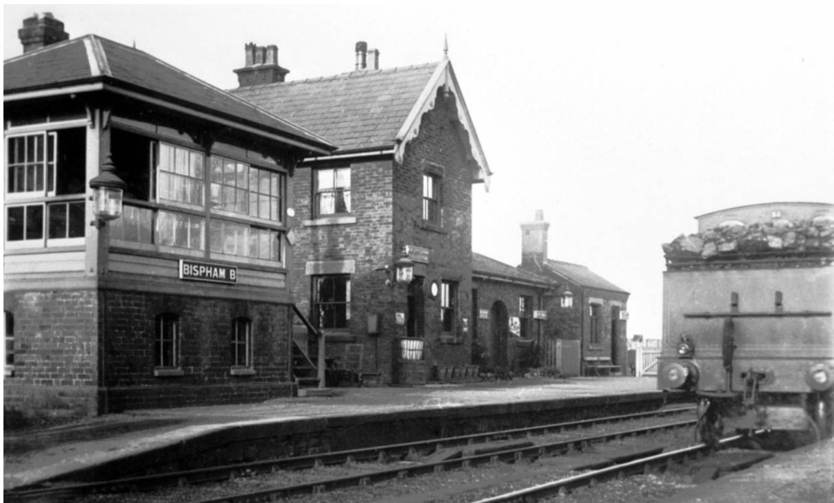
Fig. 6: Bispham (now Layton) Station in the early 20 th -century; the station house and adjacent single-storey buildings are still extant (courtesy Ted Lightbown).
