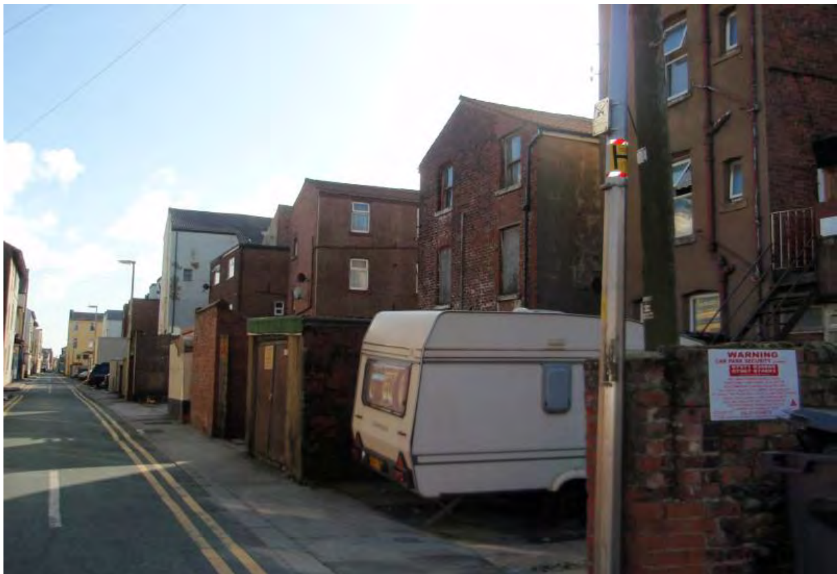
Fig.28: Typical large outriggers to the rear of lodging houses on Bolton Street North
