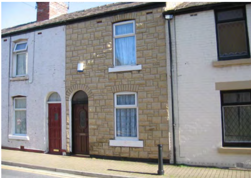
Fig.39: Concrete 'stone' cladding and painted brickwork on Caroline Street
