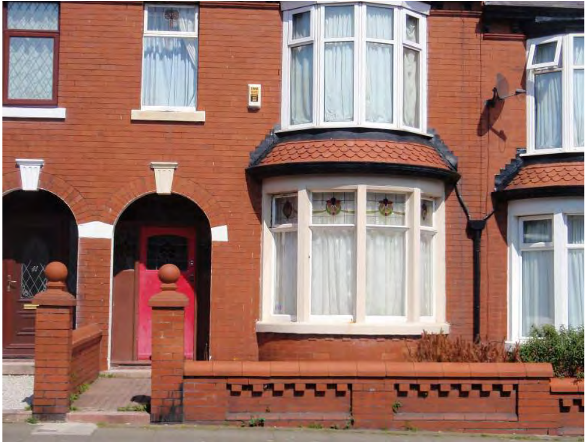
Fig. 35: Original glazing to doors and windows on Grange Road
