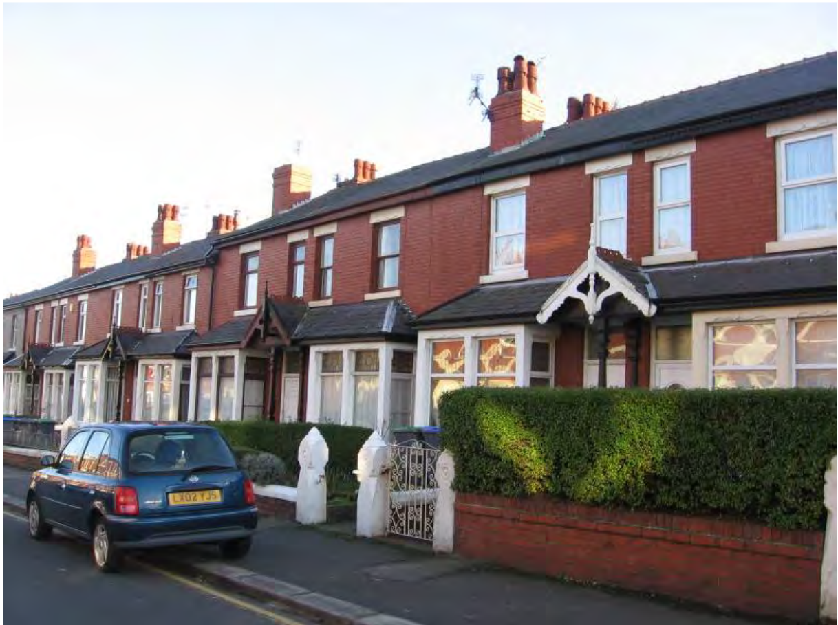
Fig. 82: Typical terrace, Leeds Road
