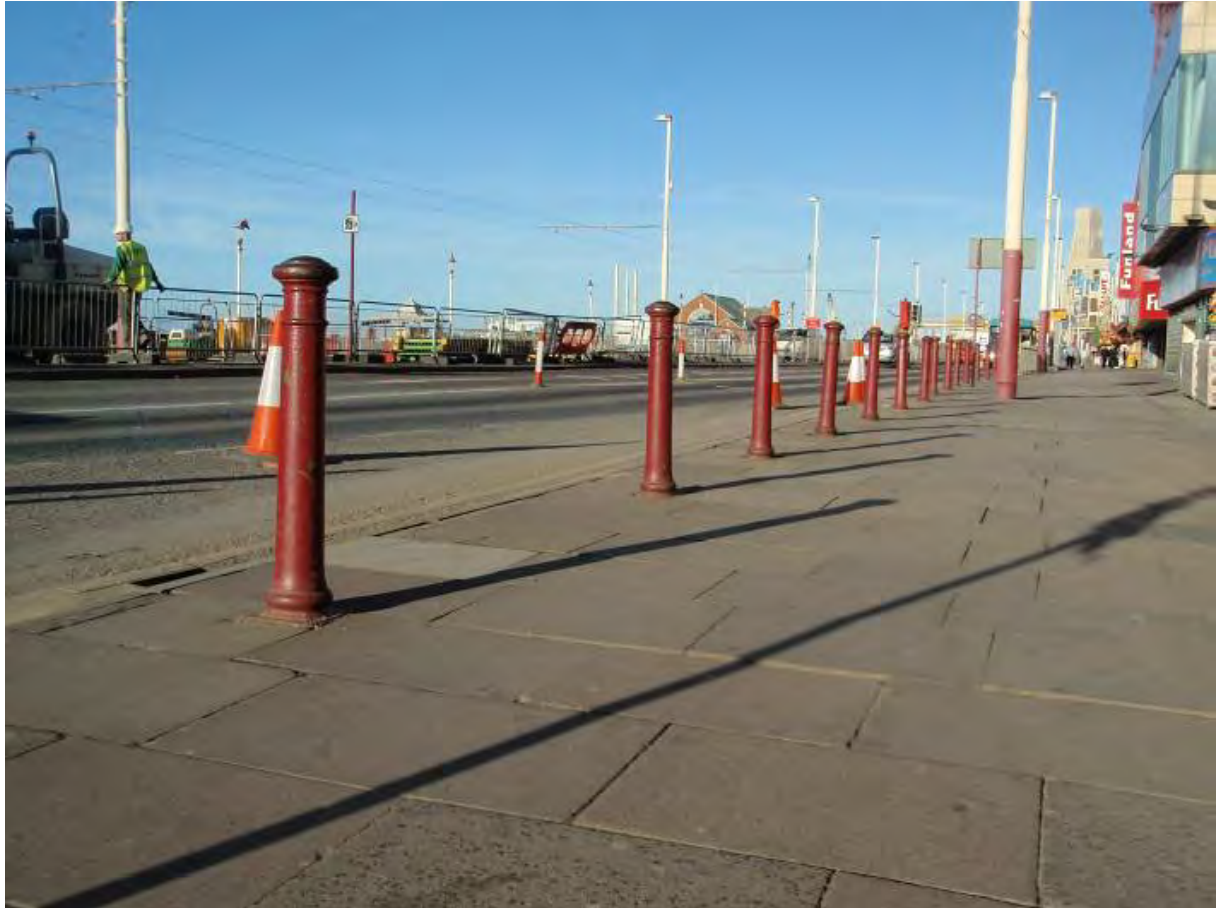
Fig. 34: Cast-iron bollards on the east side of the Promenade
