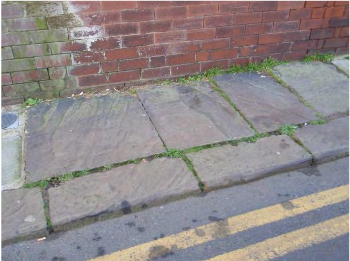
Fig. 29: Natural stone slabs and kerbs to Banks Street
