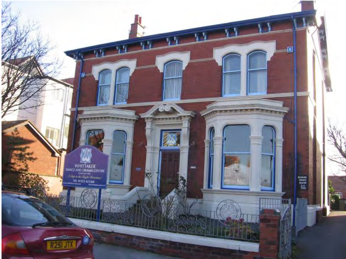
Fig. 36: Elaborate stone doorway and bays, No. 135 Hornby Road
