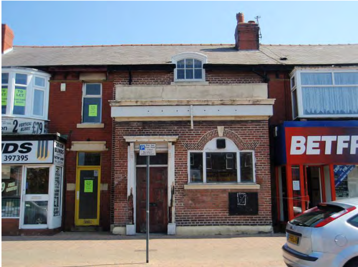
Fig. 115: No 21 Westcliffe Drive
