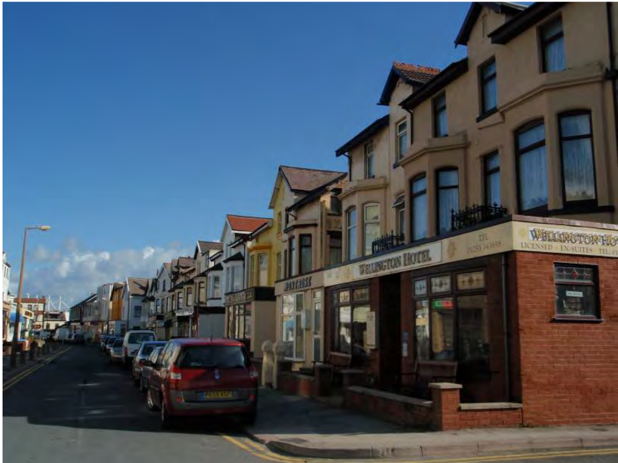
Fig.29: Strong rhythm of two-storey bays and gabled dormers on Wellington Road, disrupted by front additions.
