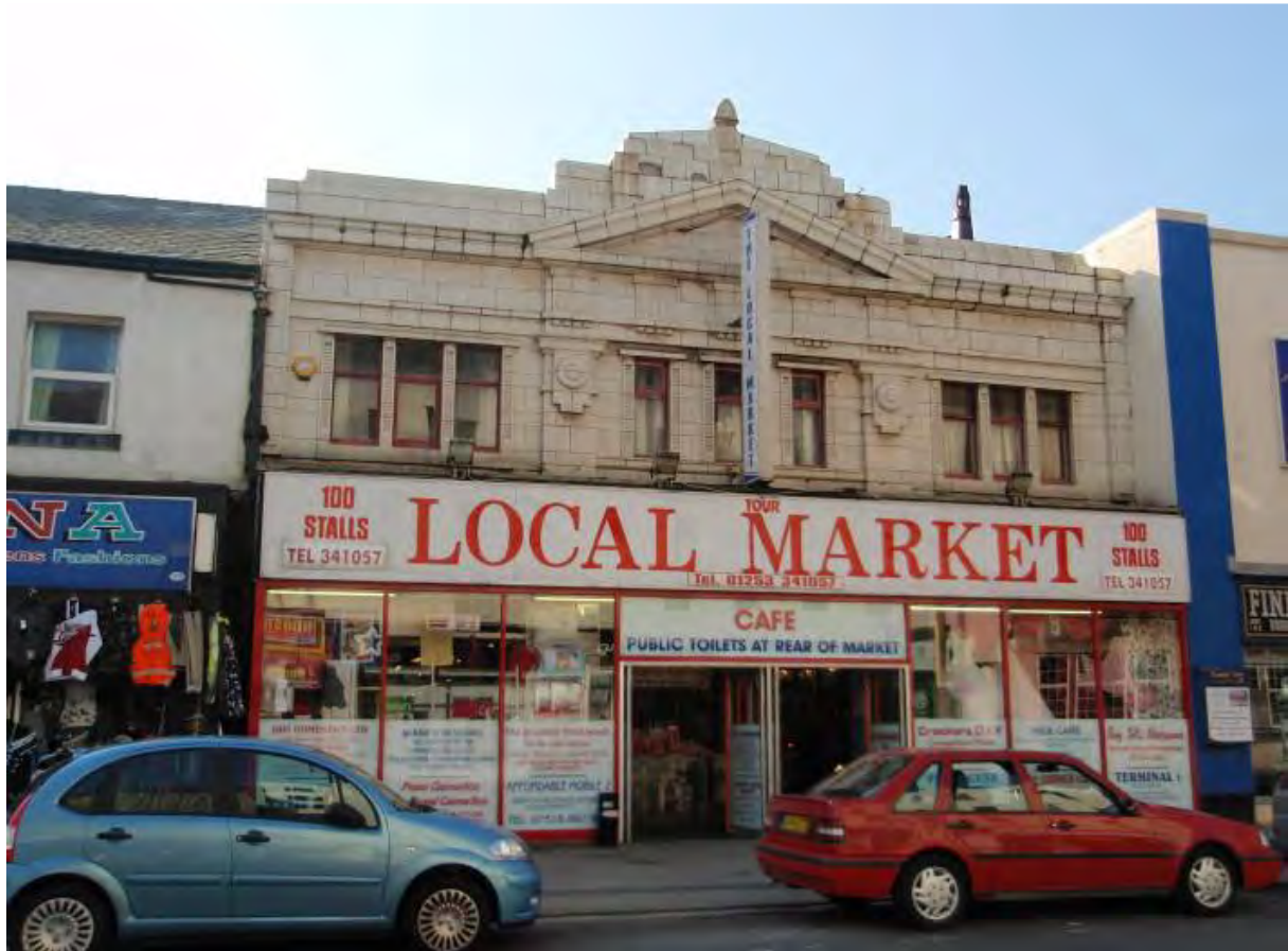
Fig. 22: No. 35 Waterloo Road
