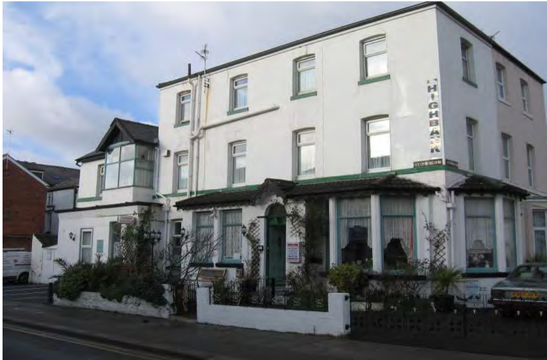
Fig.65: No.46 Banks Street, probably built in c.1870
