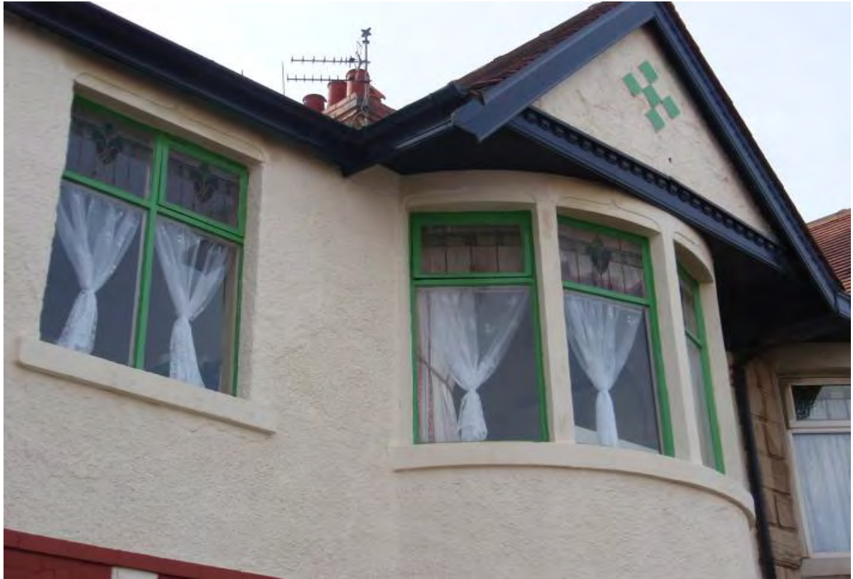
Fig. 26: Original windows on an inter-war house at 45 Dean Street
