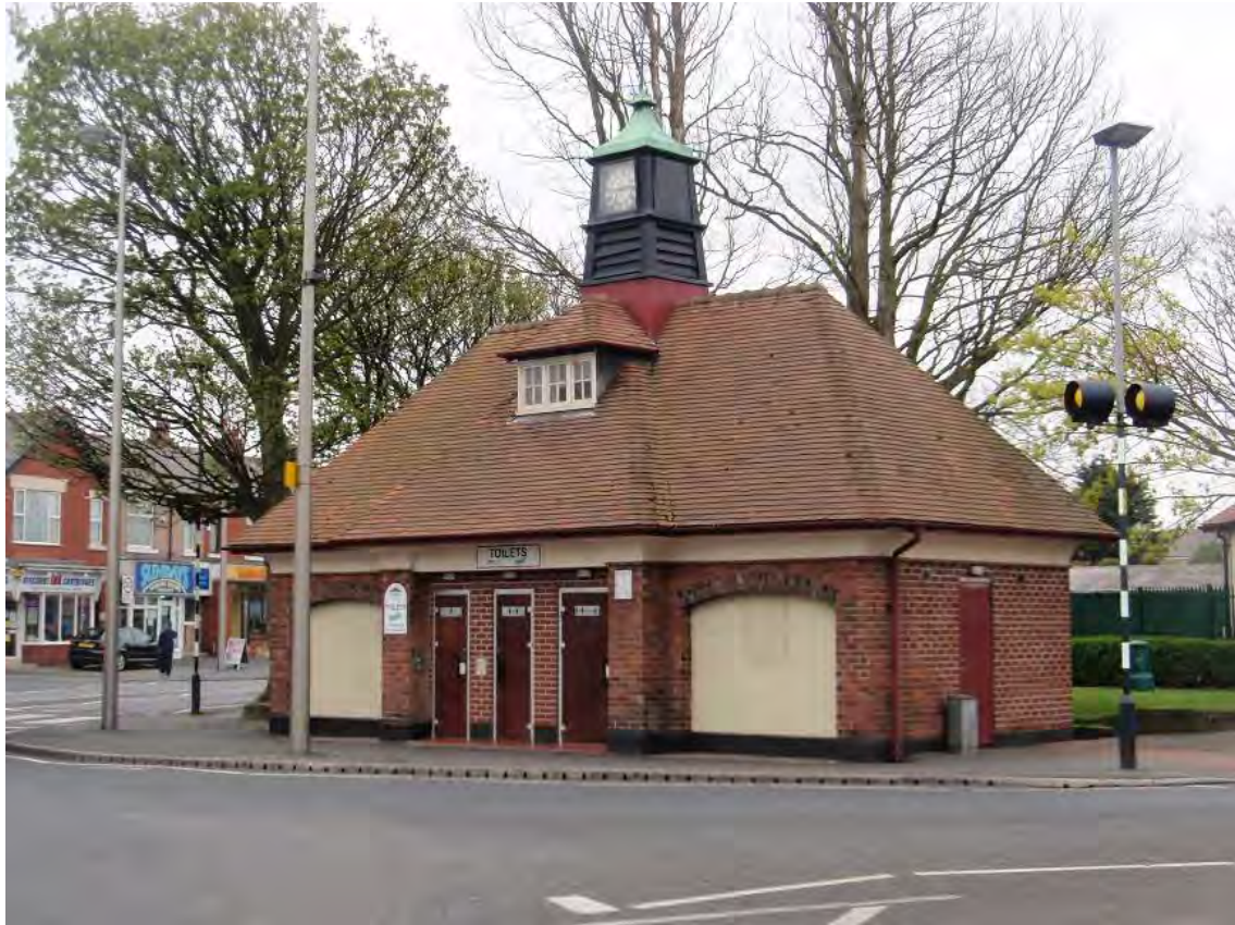
Fig. 66: The former tram shelter in Layton Square
