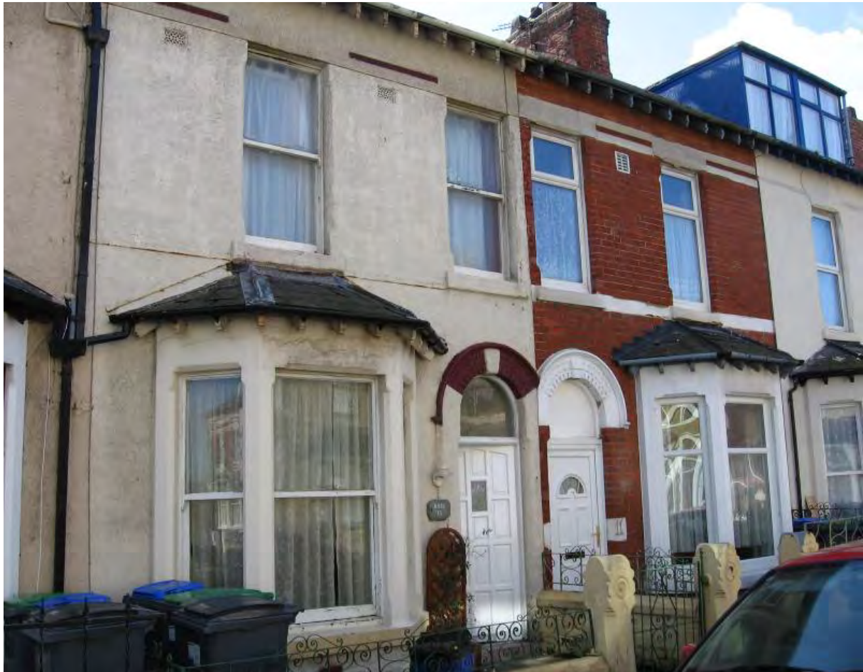
Fig.19: The contrast between rendered brick frontages and an original fair-faced brick frontage on Lowrey Terrace
