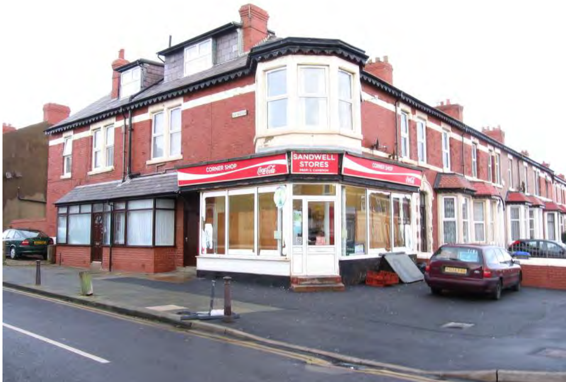
Fig.88: Corner shop on Boothroyden and Carshalton Road junction
