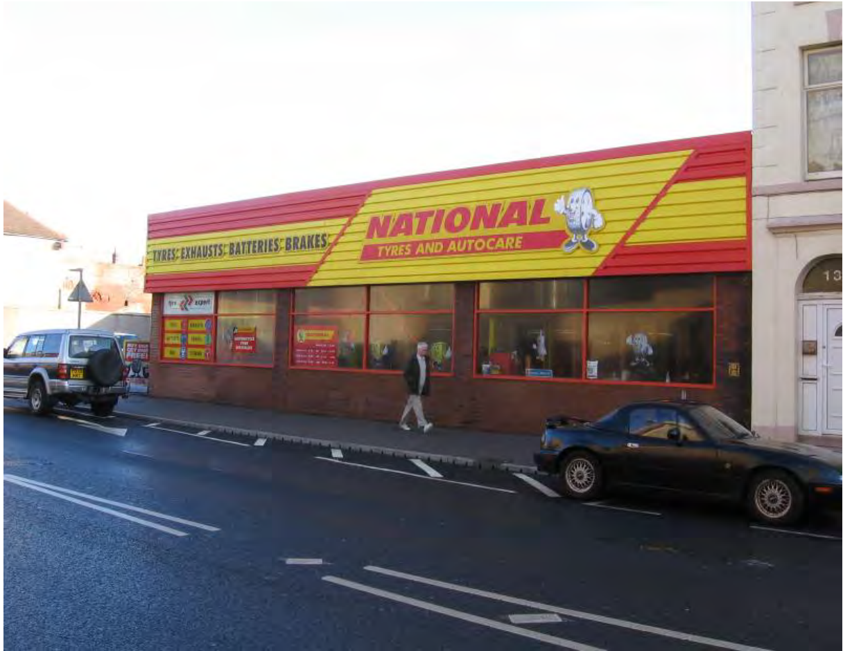
Fig. 49: Intrusive garage repair shop, on the site of a late 19 th century skating rink
