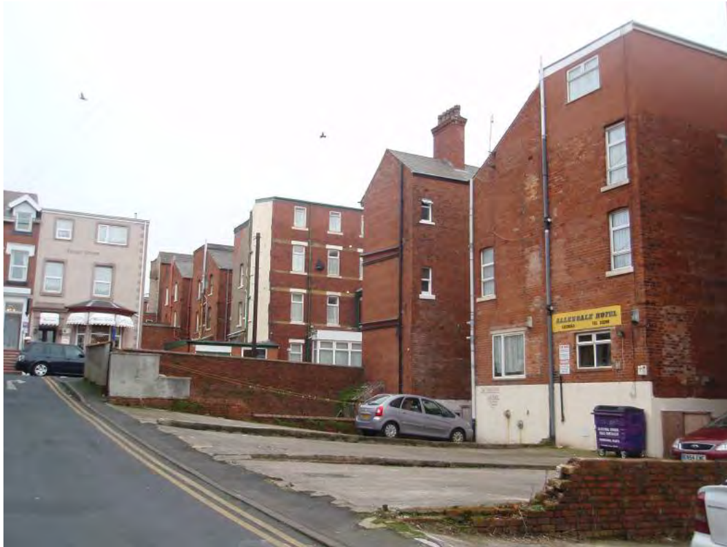
Fig. 112: South side of service lane to Albert Road
