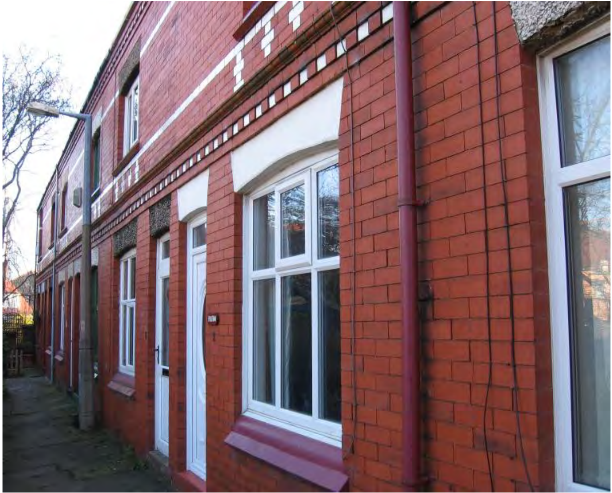
Fig. 116: Belle Vue Place faces north onto a stone paved path
