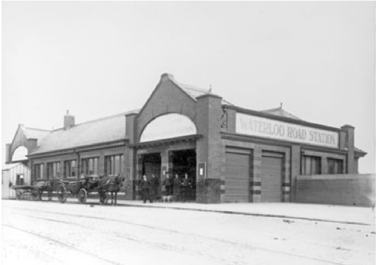
Fig. 9: Waterloo Road Station c.1900 (Blackpool Library)
