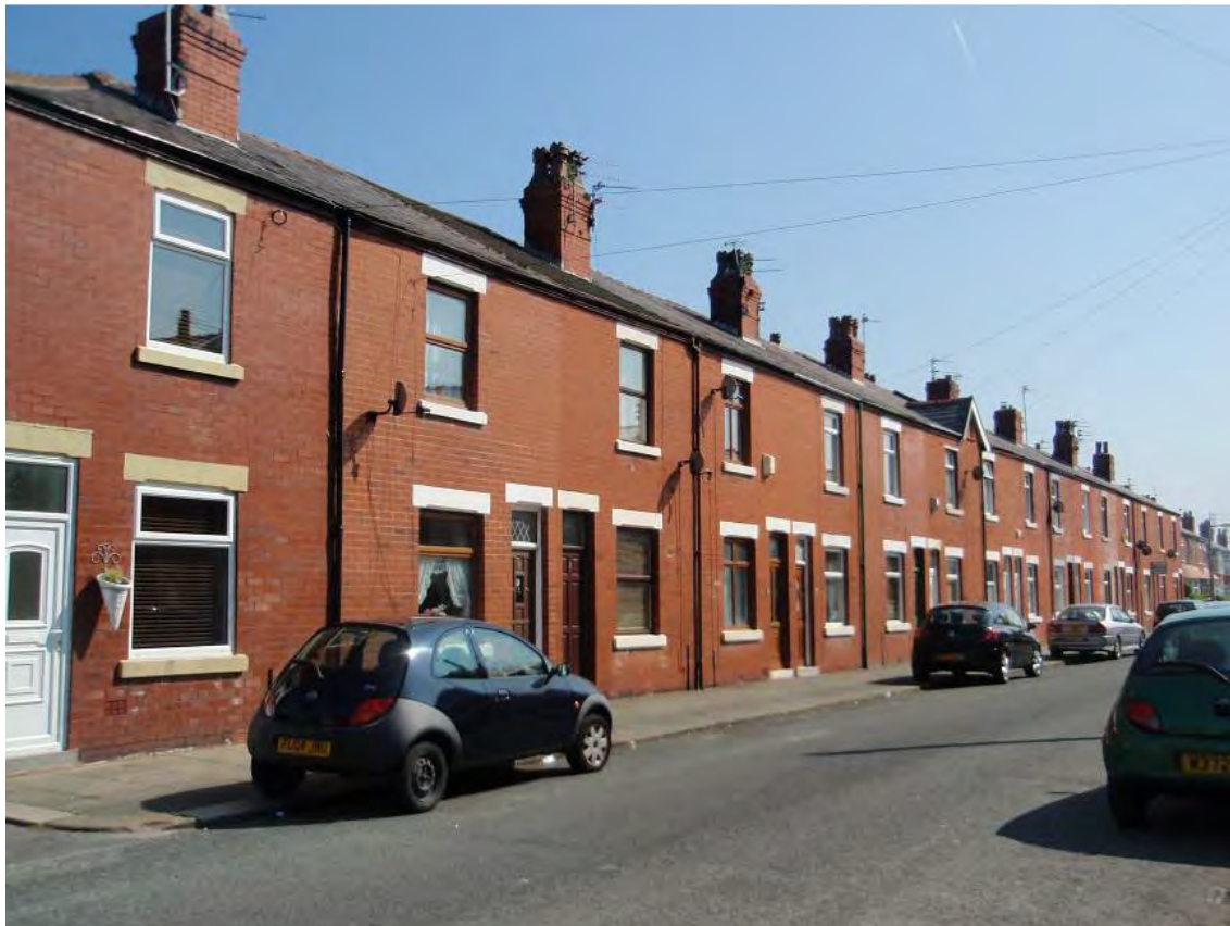
Fig. 61: Typical two-up two-down cottages on Rathlyn Avenue
