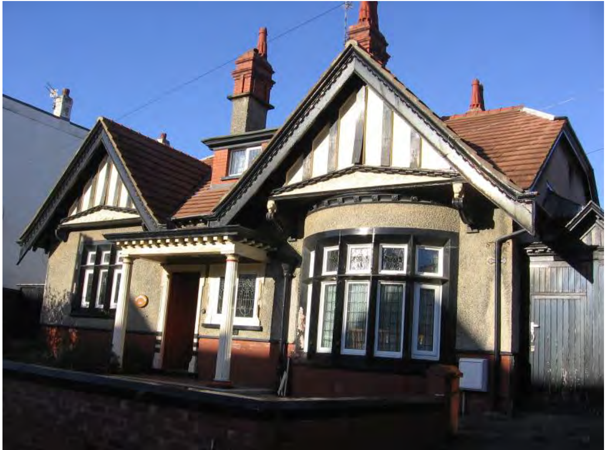
Fig. 79: Northwood, No. 165 Read's Avenue.
