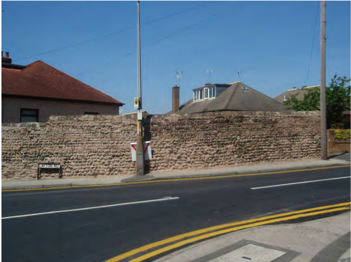
Fig. 55: Extant cobble wall at the south-west end of Layton Road
