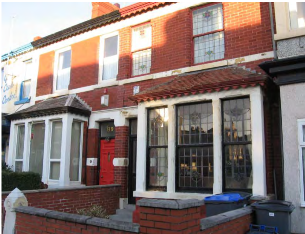
Fig.26: Early 20 th century leaded sash windows at the north end of High Street
