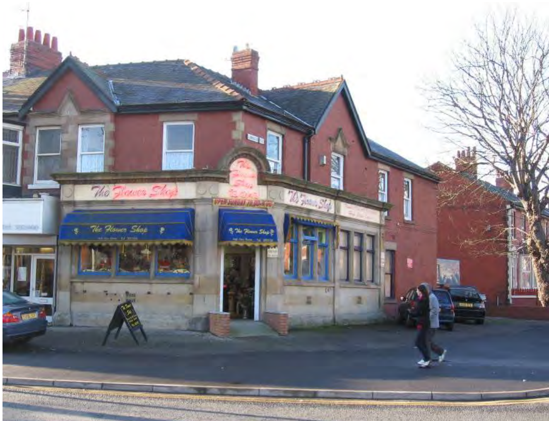
Fig. 39: Former bank at junction of Leamington Road and Whitegate Drive
