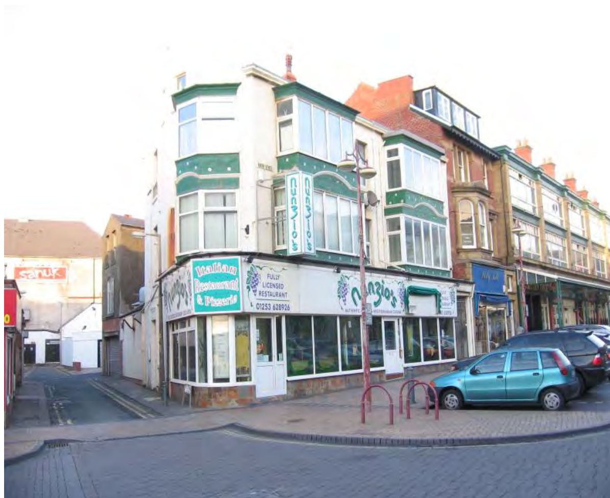
Fig.56: The north side of Queen Street with No 6, a former house sandwiched between early 20 th century shops
