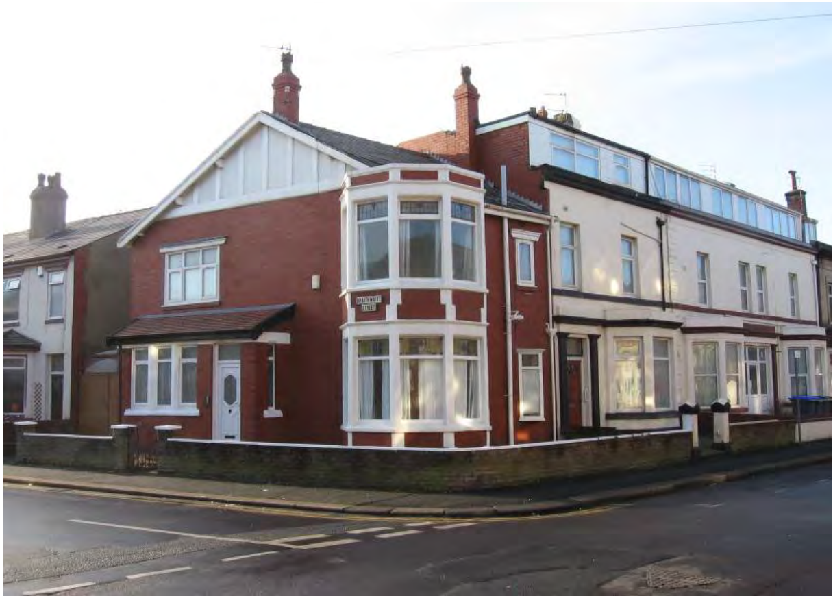
Fig.83: Bute Avenue corner house, built in the early 1900s
