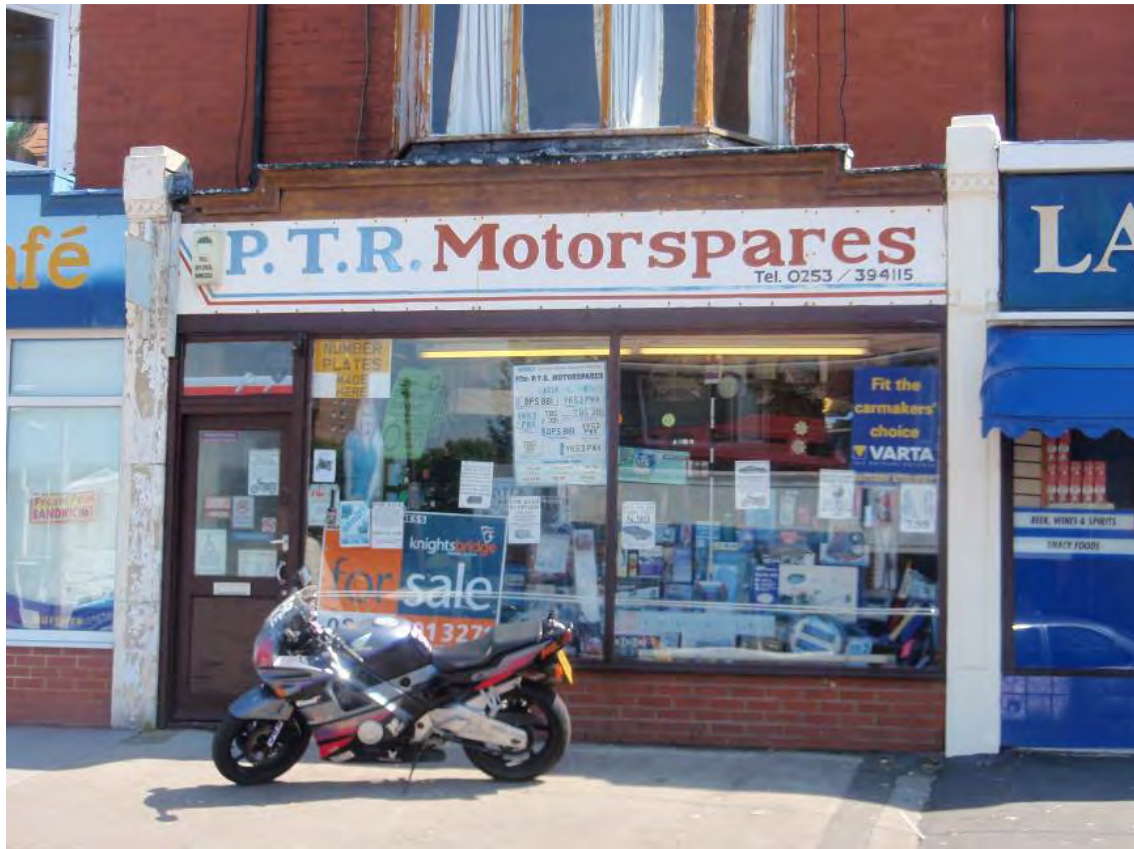
Fig.42: Retained pilasters and cornice to shopfront at No. 163 Layton Road
