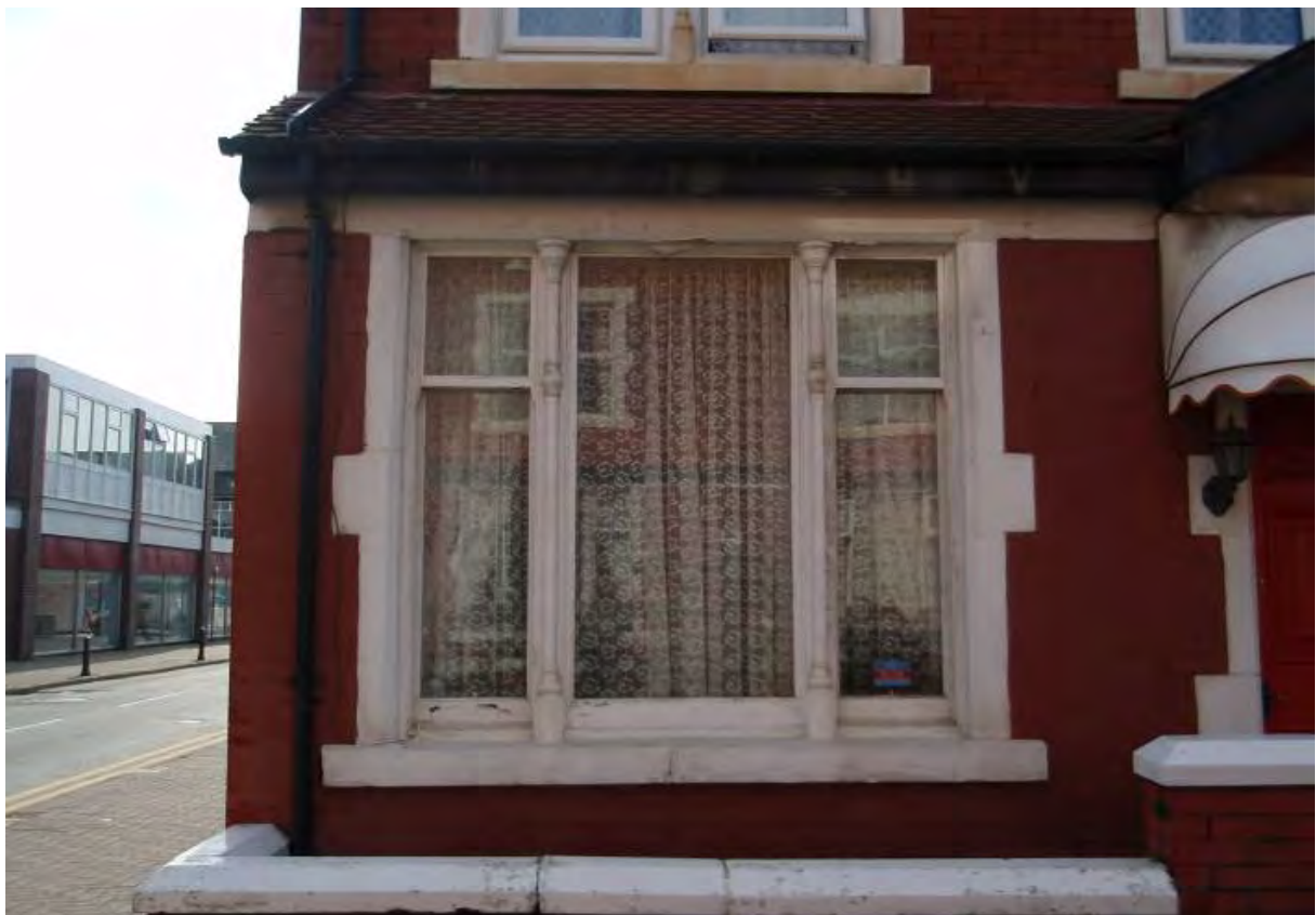
Fig. 25: Tripartite window on St Bede's Avenue.
