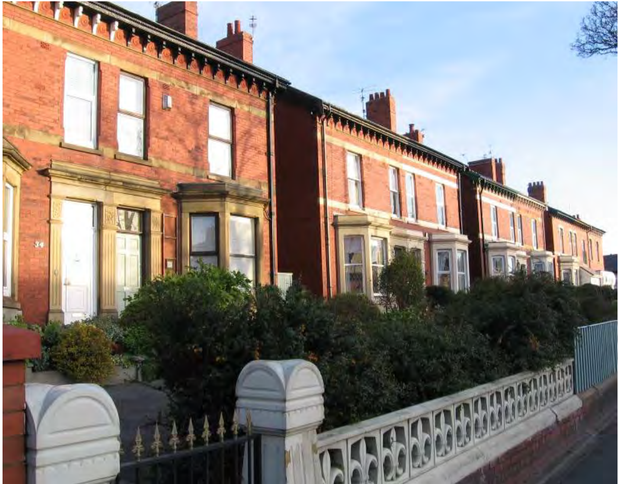
Fig. 86: Large semi detached houses – Nos. 30-42
