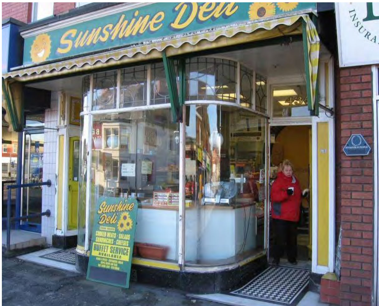
Fig. 38: Rare example of an early 20 th century shopfront, No. 43 Whitegate Drive
