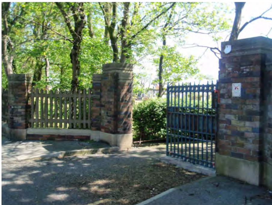
Fig. 53: Boundary treatments to the Mansfield Road edge of the cemetery
