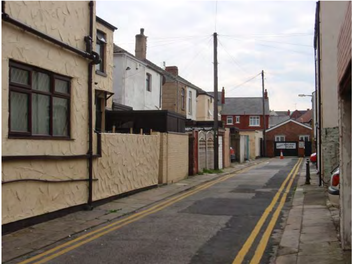
Fig. 58: Backs of terraces on the south-east side of Byron Street
