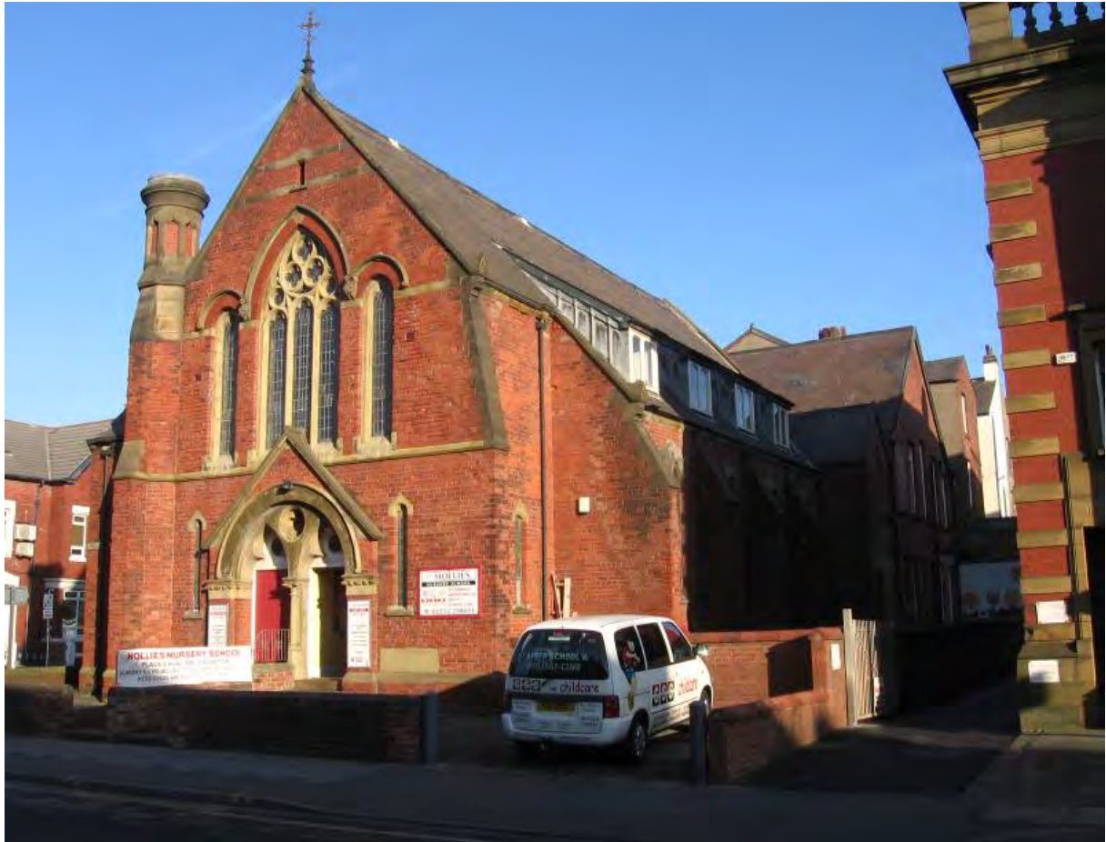
Fig.21: Former United Methodist Church on Abingdon Street is now a children's nursery
