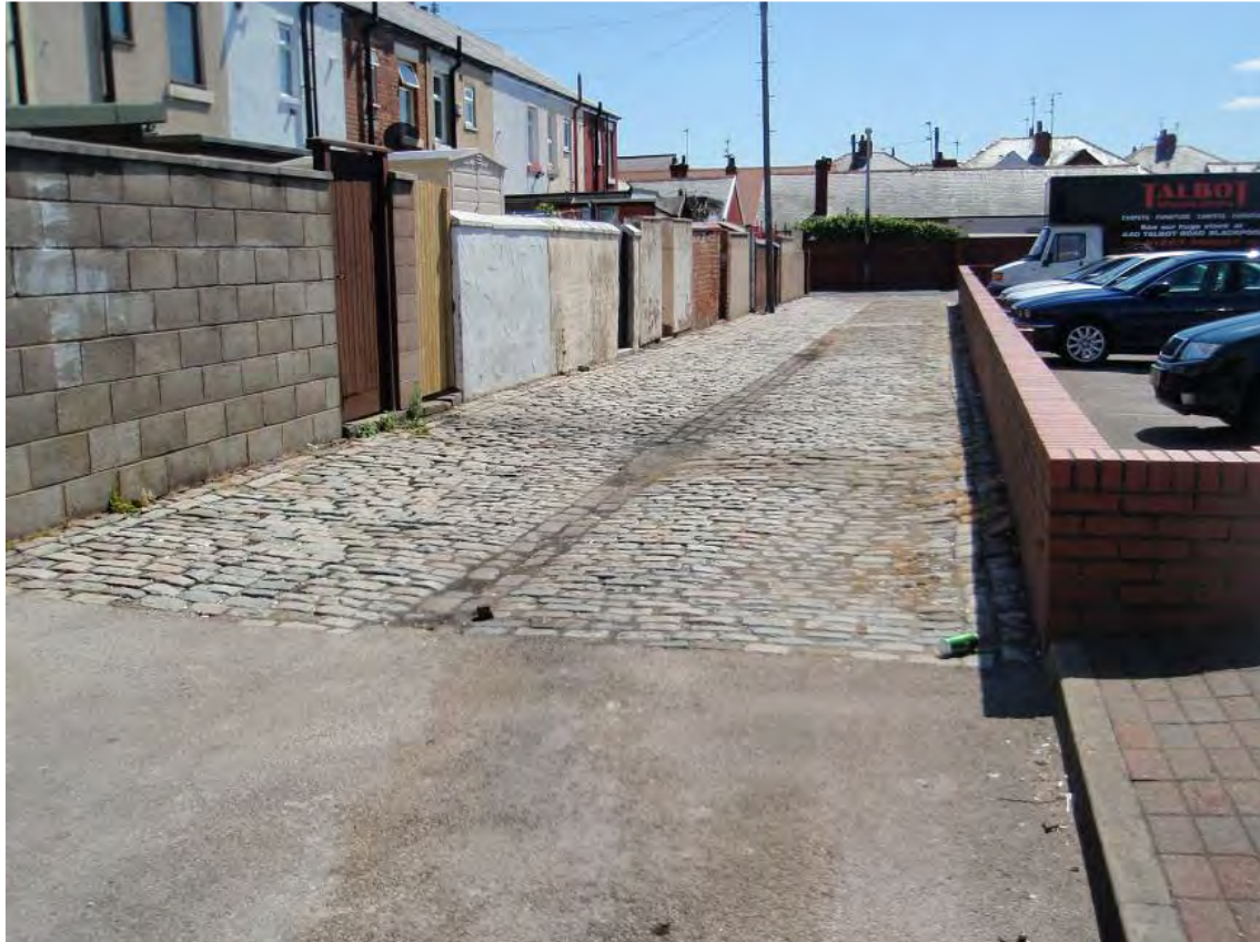
Fig. 57: Setted surface to the rear of Whittaker Avenue
