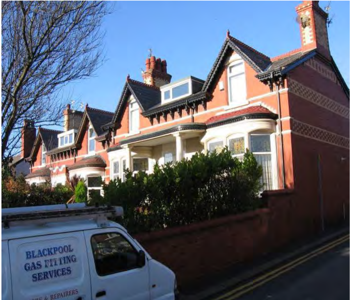
Fig. 114: Nos. 2-4, an unusual example of a pair of semi-detached one and half storey houses with good details.
