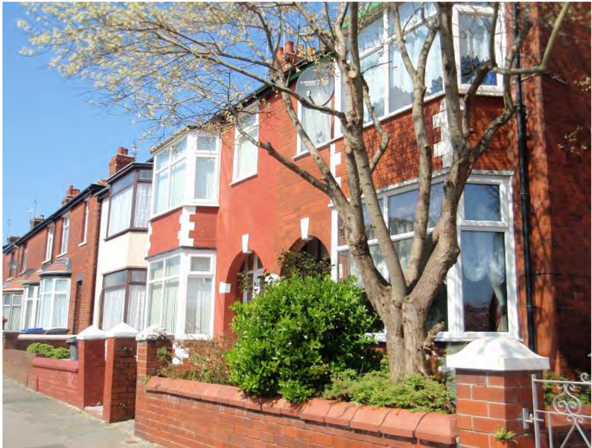
Fig. 33: Different styles of bay windows on Grenfell Avenue
