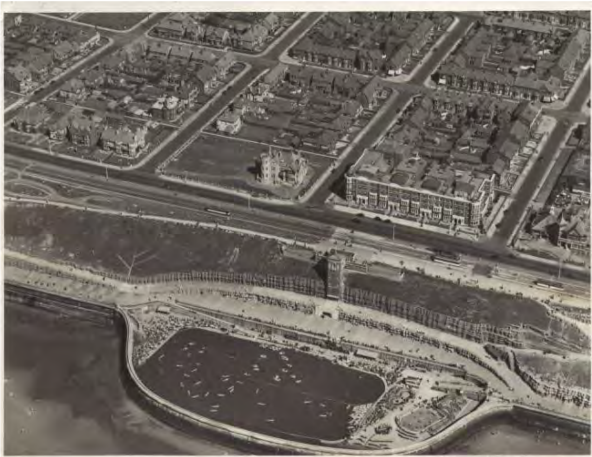
Fig. 5: North Prom from the air, c.1930, showing part of the artificial cliffs, the cabin lift, boating pool, Uncle Tom's Cabin pub, and 'The Castle', a private residence. (Image from www.rossallbeach.co.uk )
