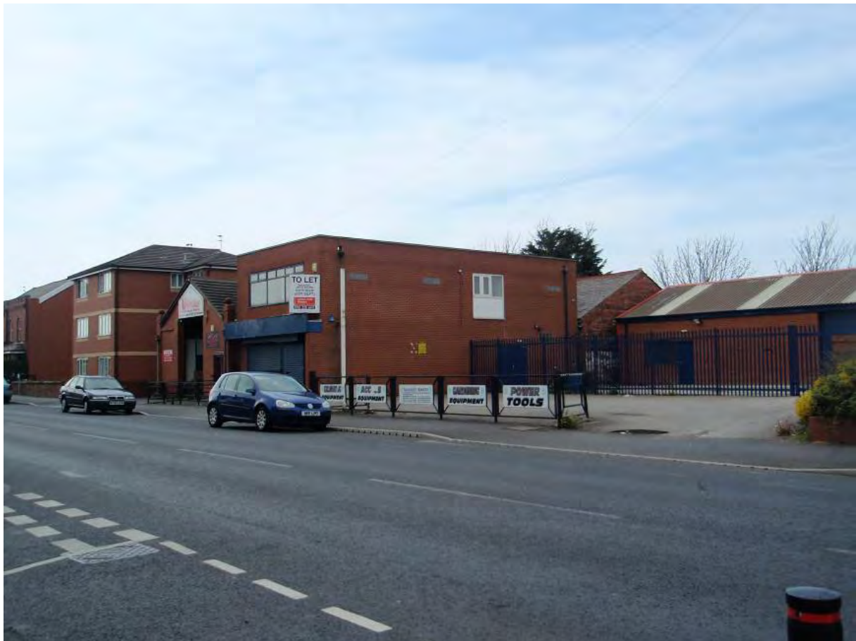
Fig. 126: Post-war infill on Talbot Road
