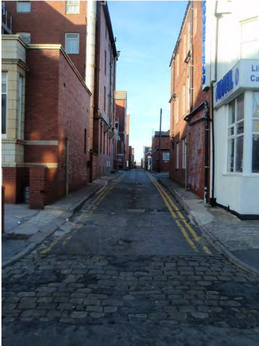
Fig. 38: Service lane to the east of the Cliffs Hotel
