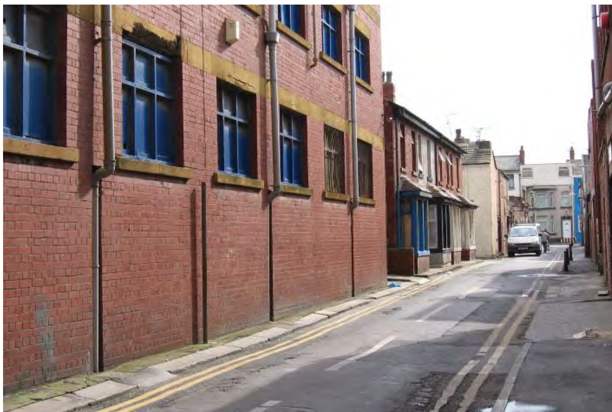
Fig. 60: The east side of Bath Street from the north
