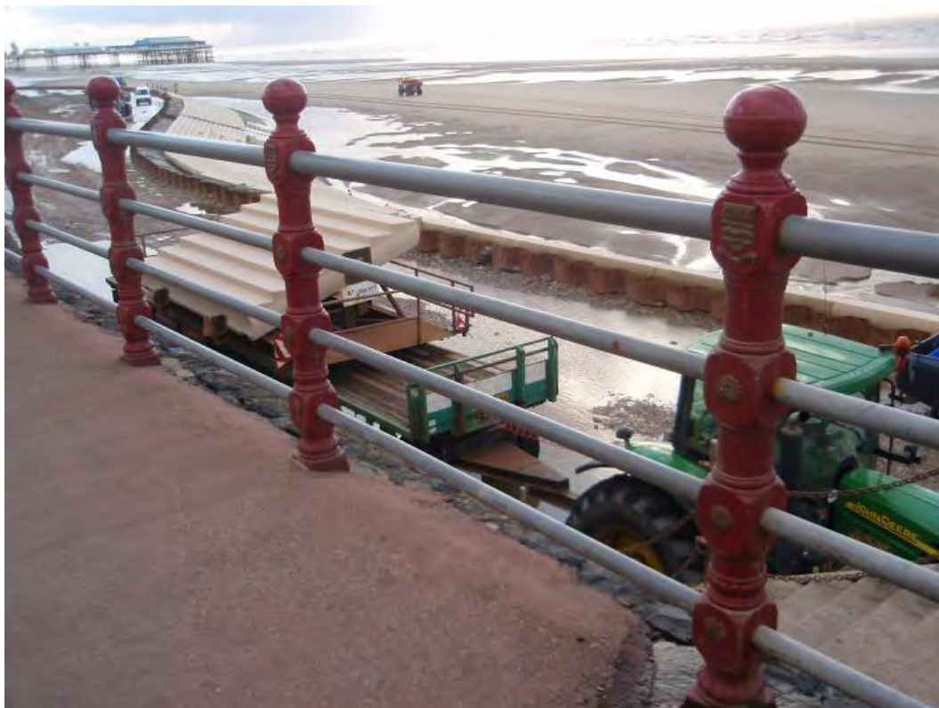
Fig. 33: 20 th -century synthetic railings near North Pier
