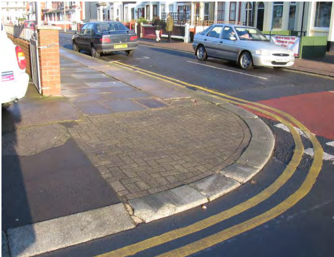
Fig.34: Typical modern mix of concrete paviours, kerbs, paving and tarmac on High Street
