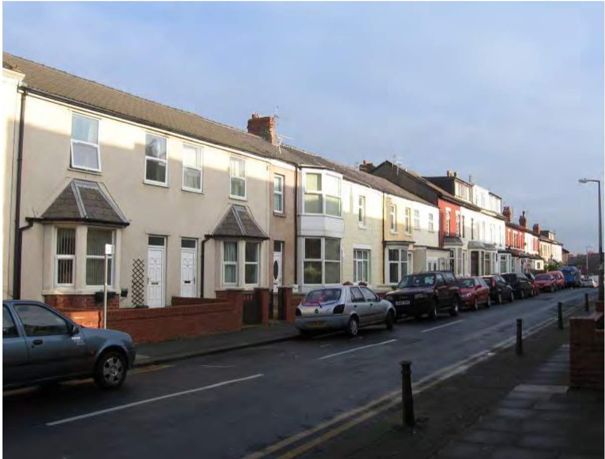
Fig.82: Eaves Street north side; terrace of mixed character with some infill
