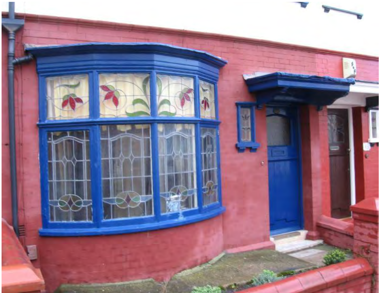
Fig.27: Ormond Avenue, 1920s leaded casements and doors.
