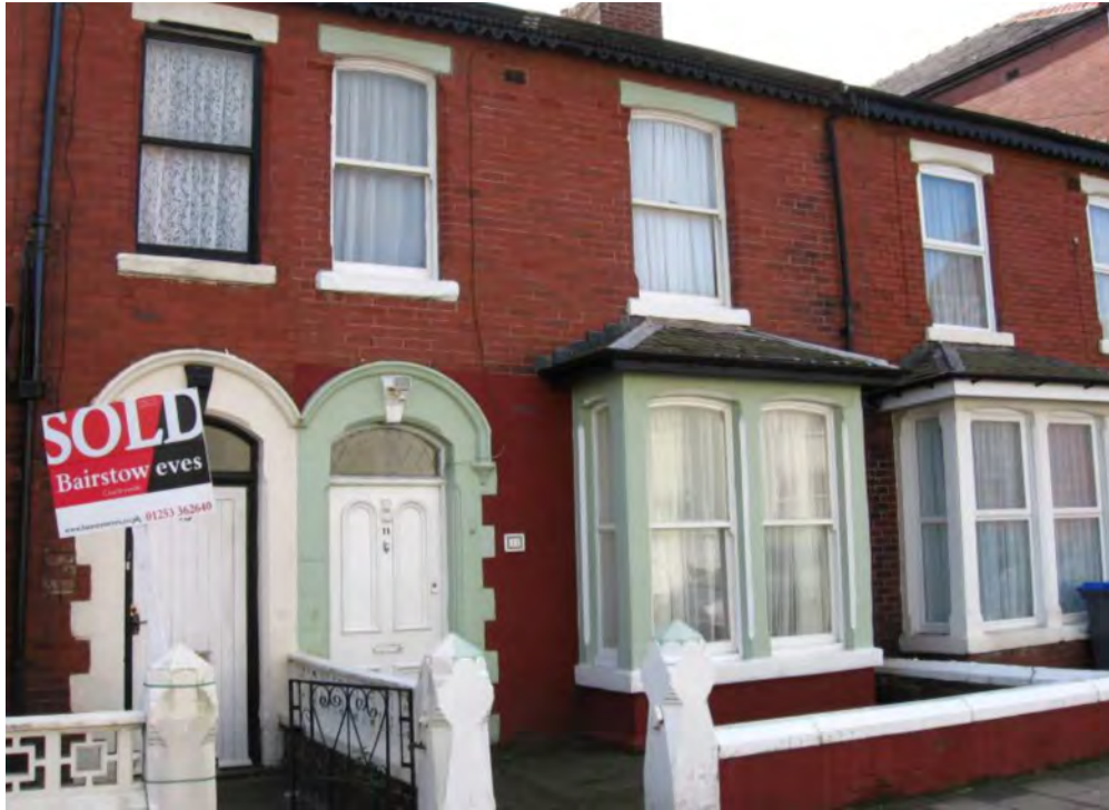
Fig.38: Rare original sash windows and panelled door at No.11 Clare Street, with replacement windows to adjoining houses
