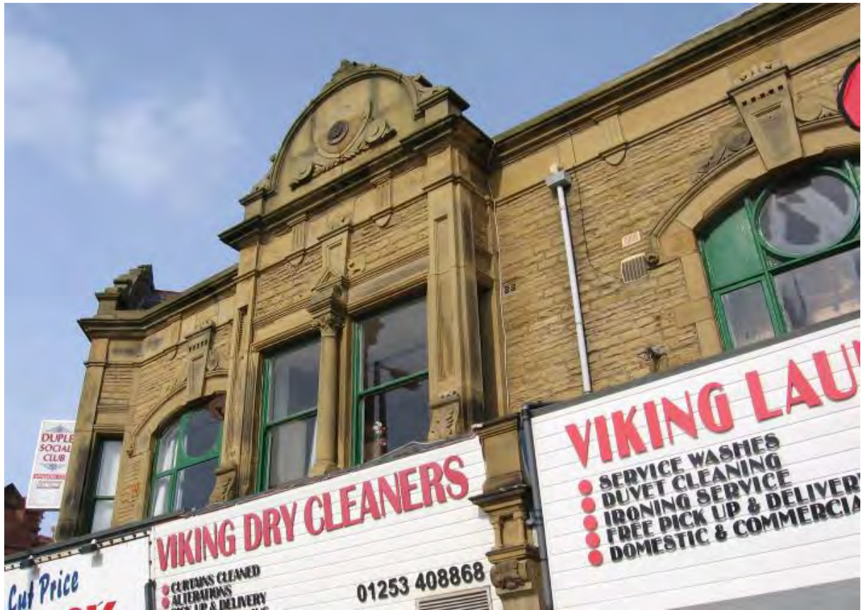
Fig. 18: South elevation of 33-36 Station Road
