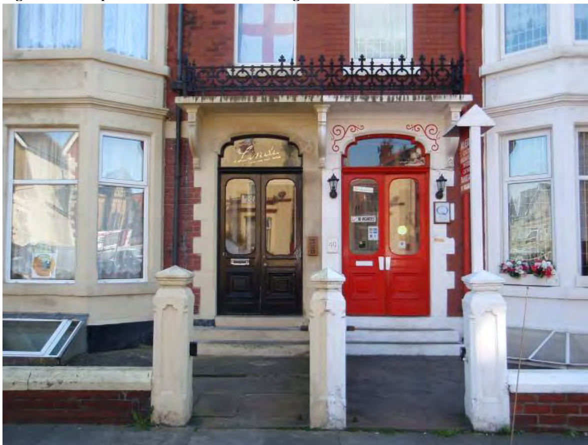
Fig. 28: Original door sets on Station Road
