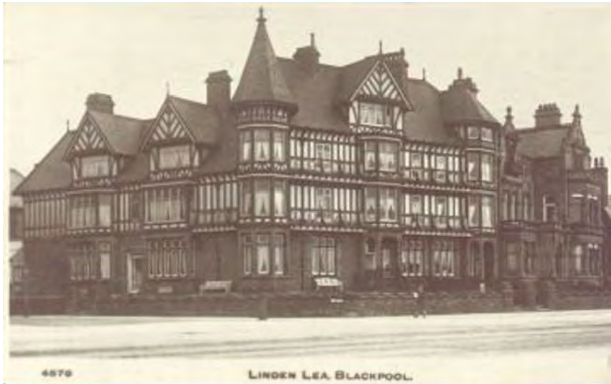
Fig. 59: 'Linden Lea' (No 487 Promenade & No. 3 Dean Street) in the early 20 th century (Image from www.rossallbeach.co.uk )
