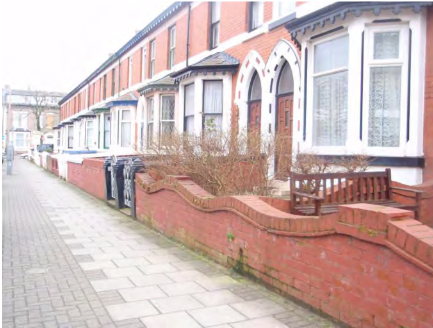
Fig. 30: A continuous, if partially rebuilt, boundary wall on the south side of Adelaide Street
