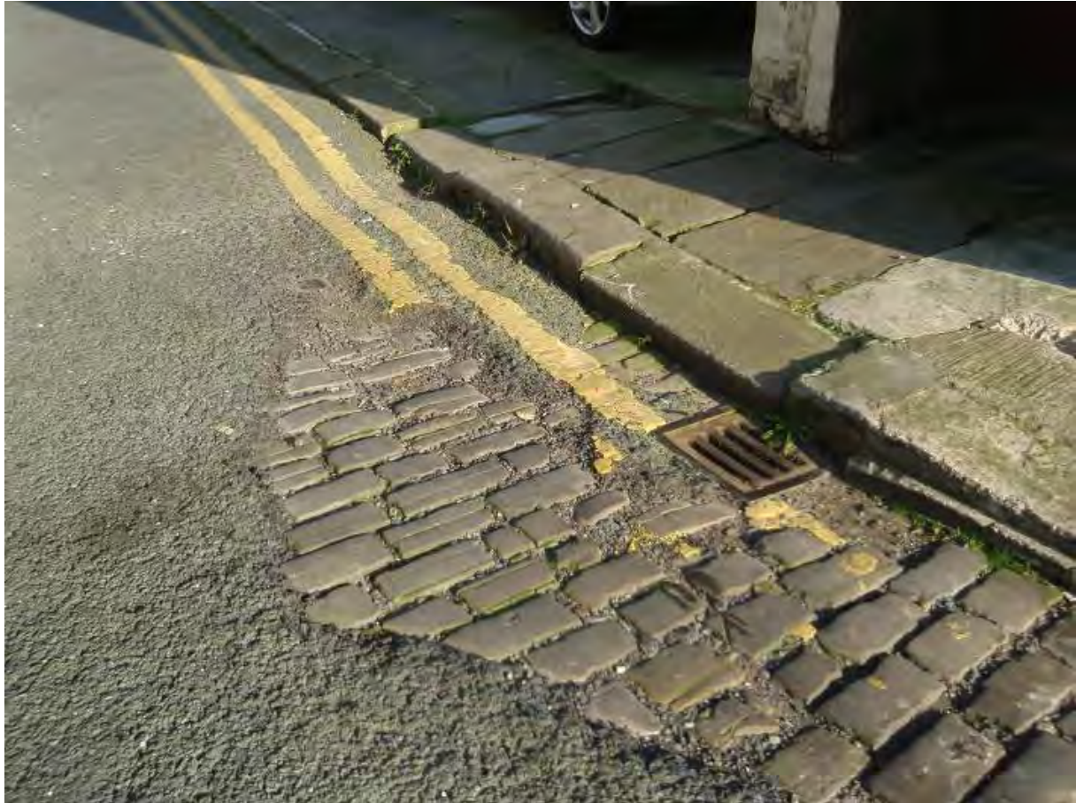
Fig. 28: Exposed stone setts on Banks Street
