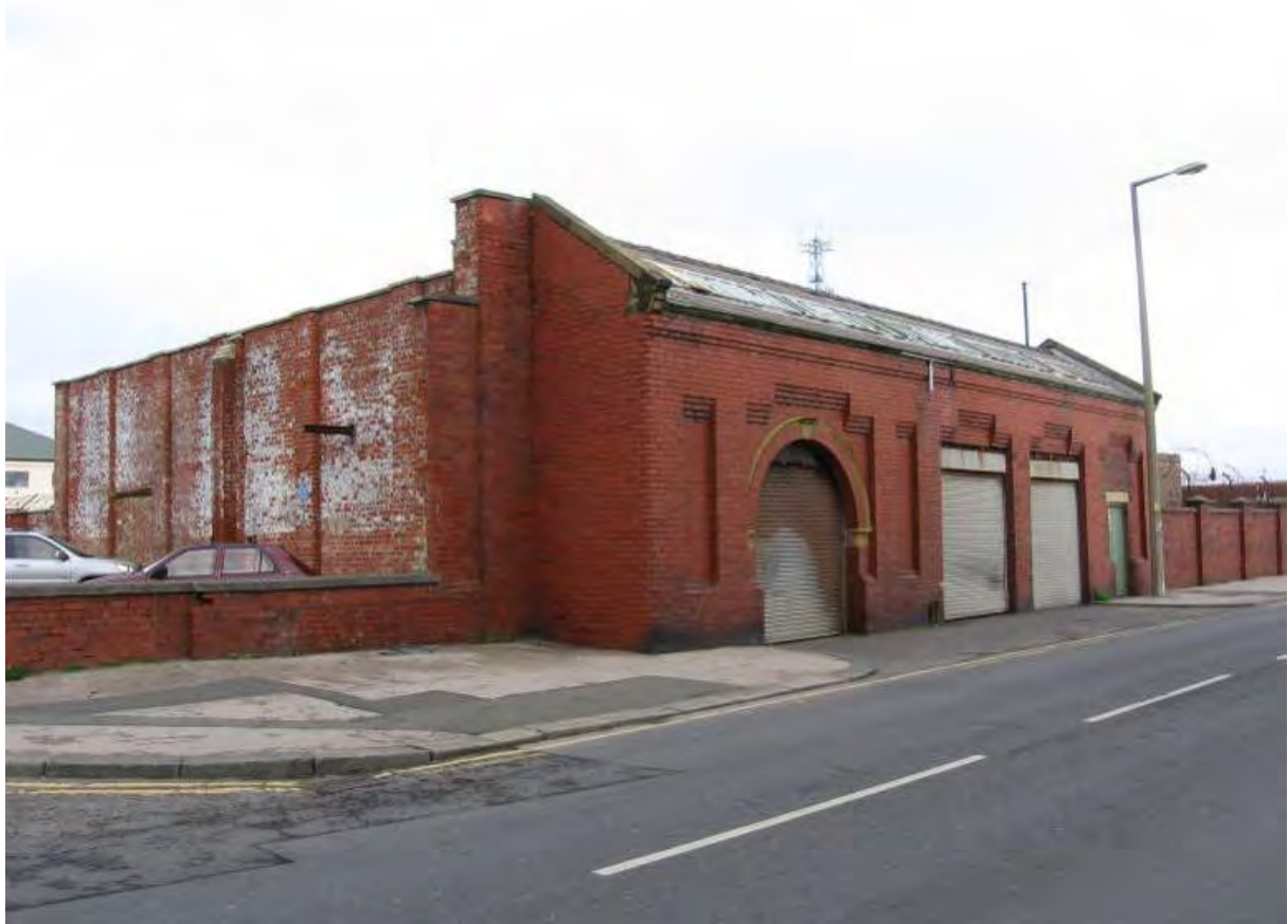
Fig.51: Remains of the former tram depot on the north side of Rigby Road
