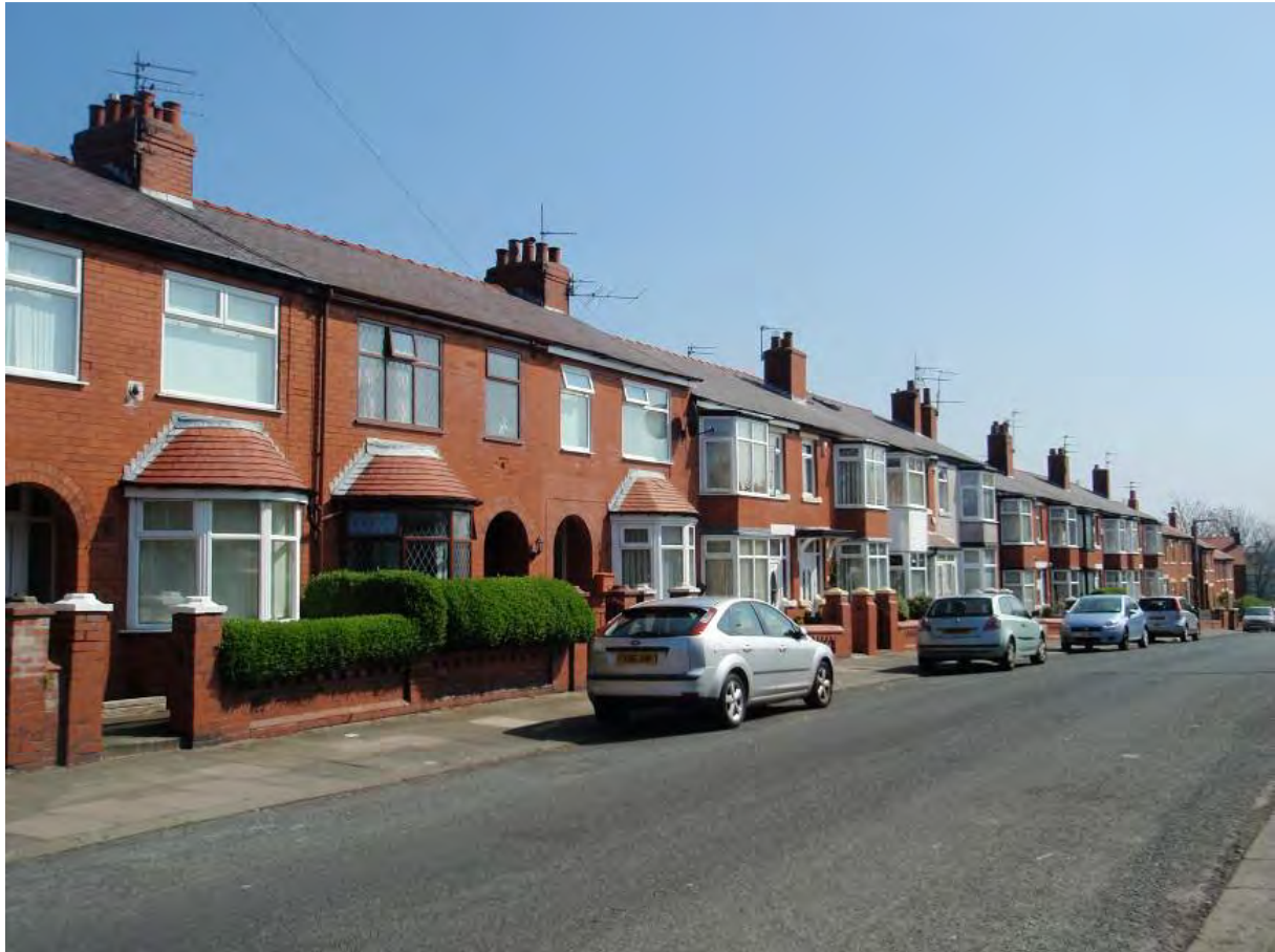
Fig. 102: North side of Rathlyn Avenue, from the west
