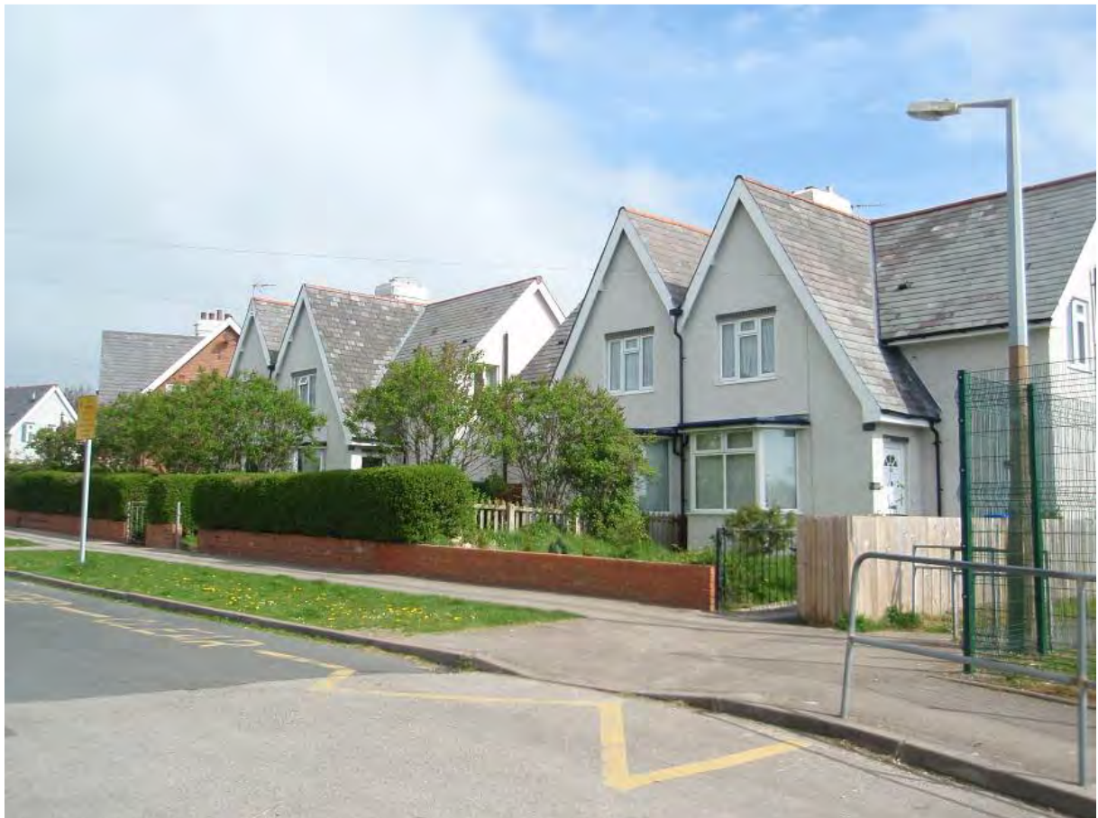
Fig. 81: Nos 31-55 Meyler Avenue
