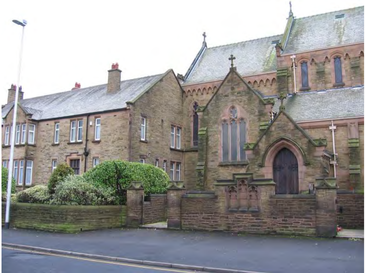
Fig. 61. St Kentigern, the presbytery and boundary walls.
