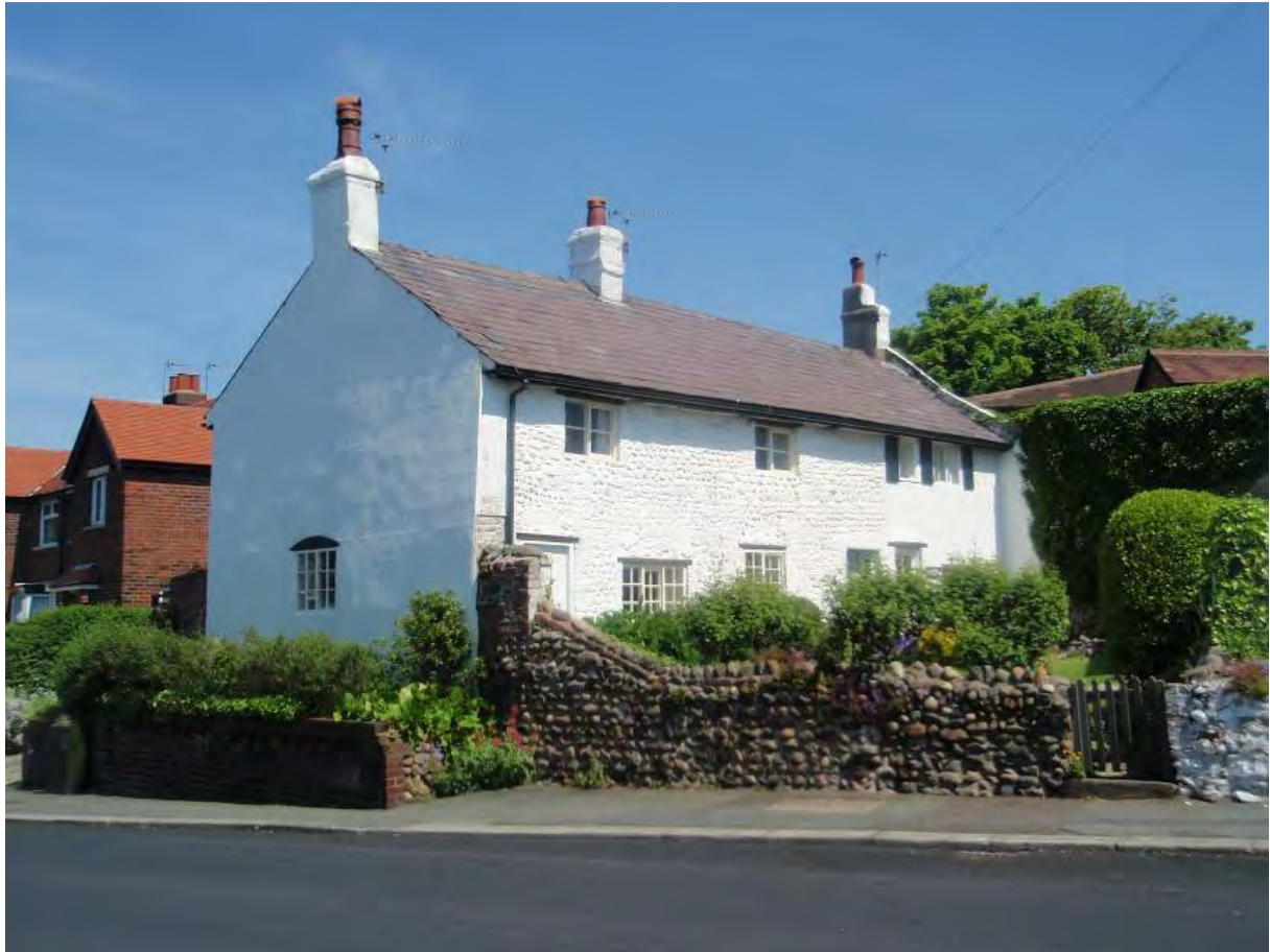
Fig. 30: No 239 Layton Road, cobble construction
