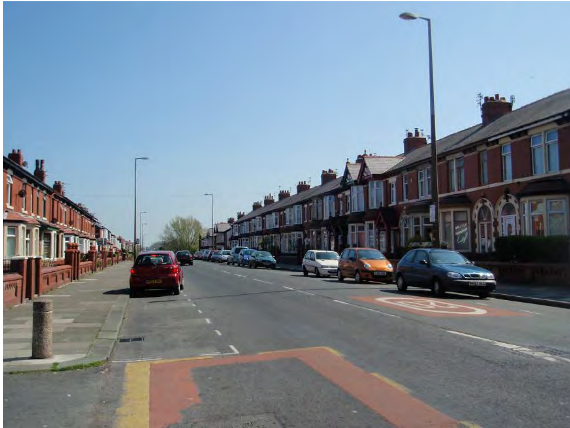
Fig. 31: Grange Road, retained chimney stacks and pots
