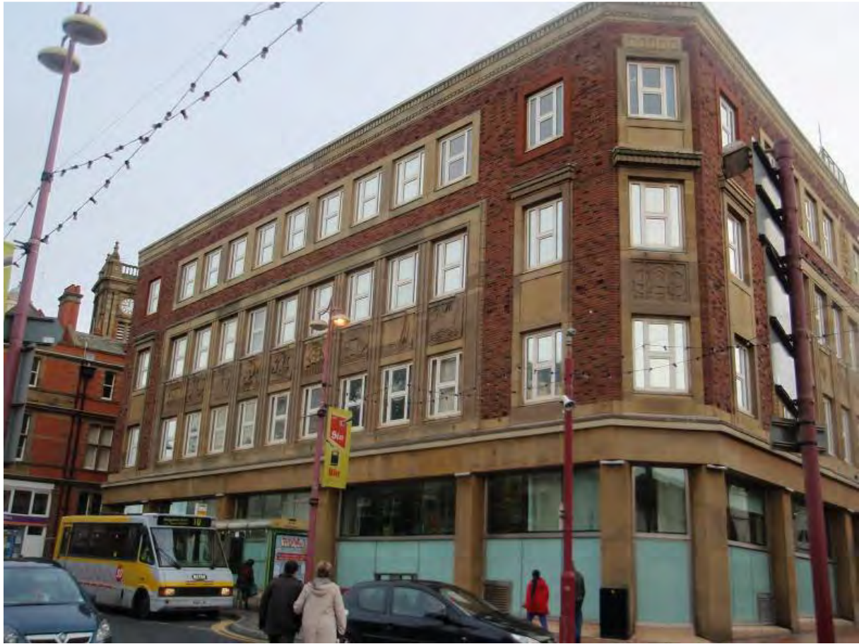
Fig. 71: The west elevation of the Progress Building with the Town Hall in the background
