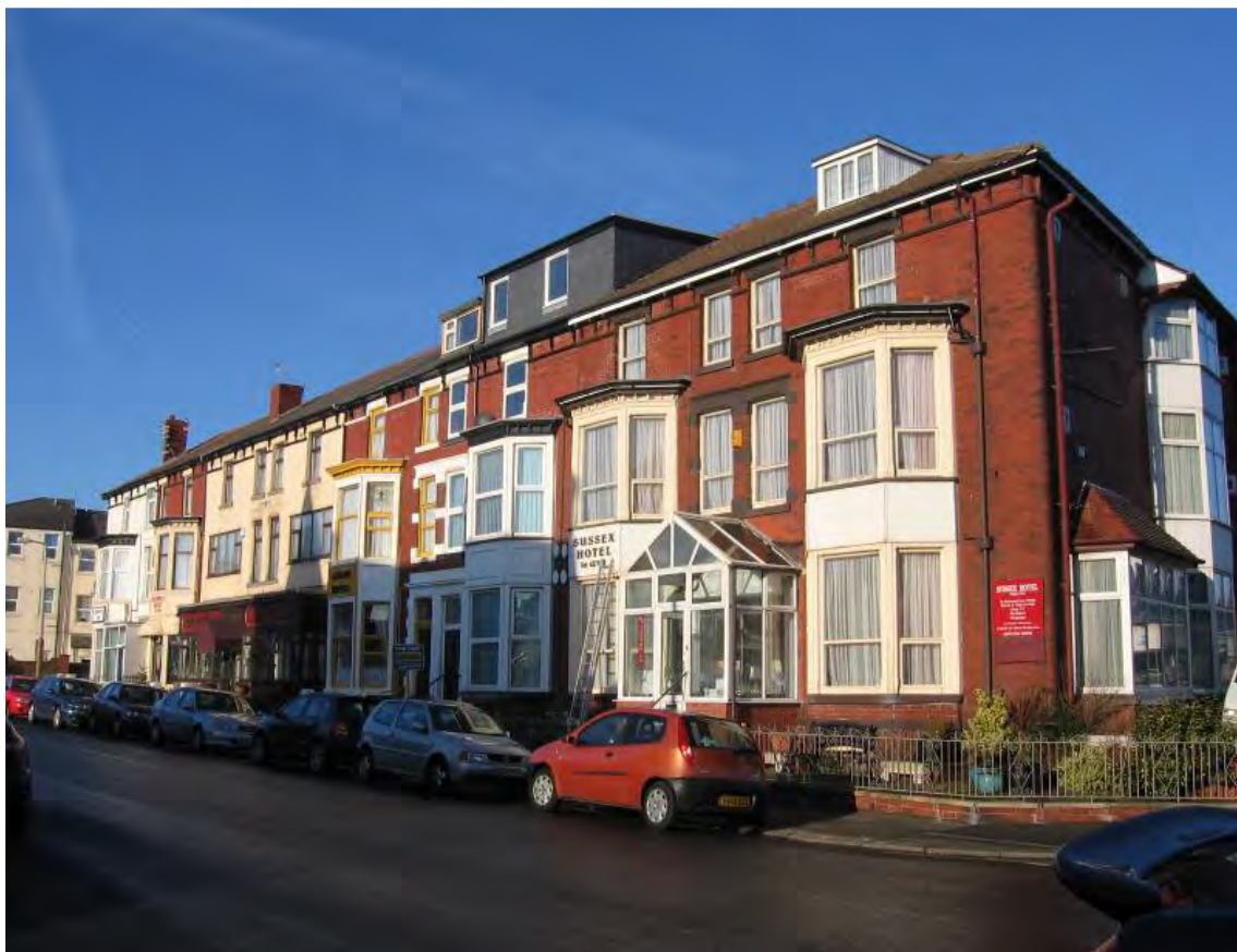
Fig.78: Terrace built c.1880 on the north side
