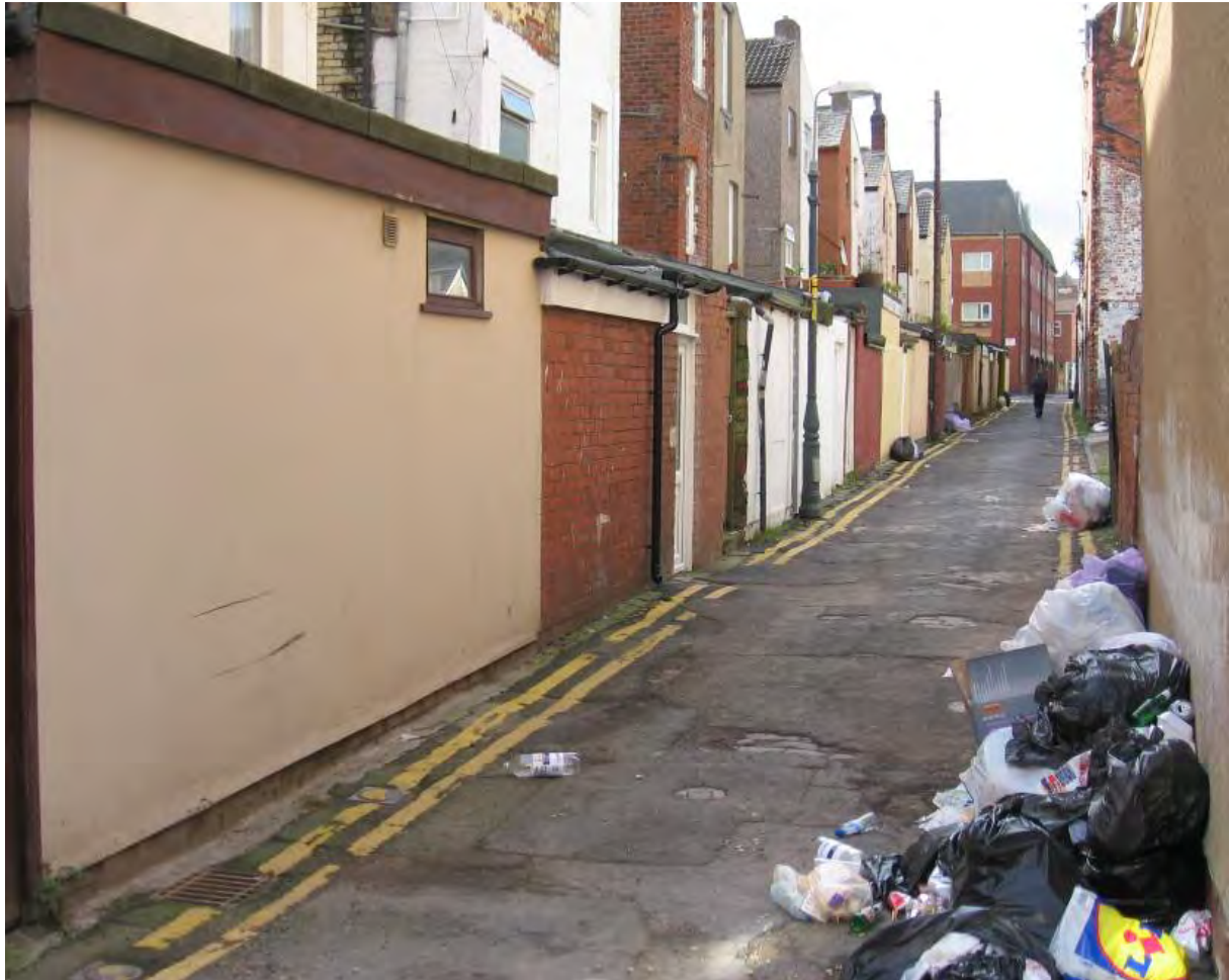
Fig.24: Alley off Coop Street, with rear extensions and rebuilt boundary walls
