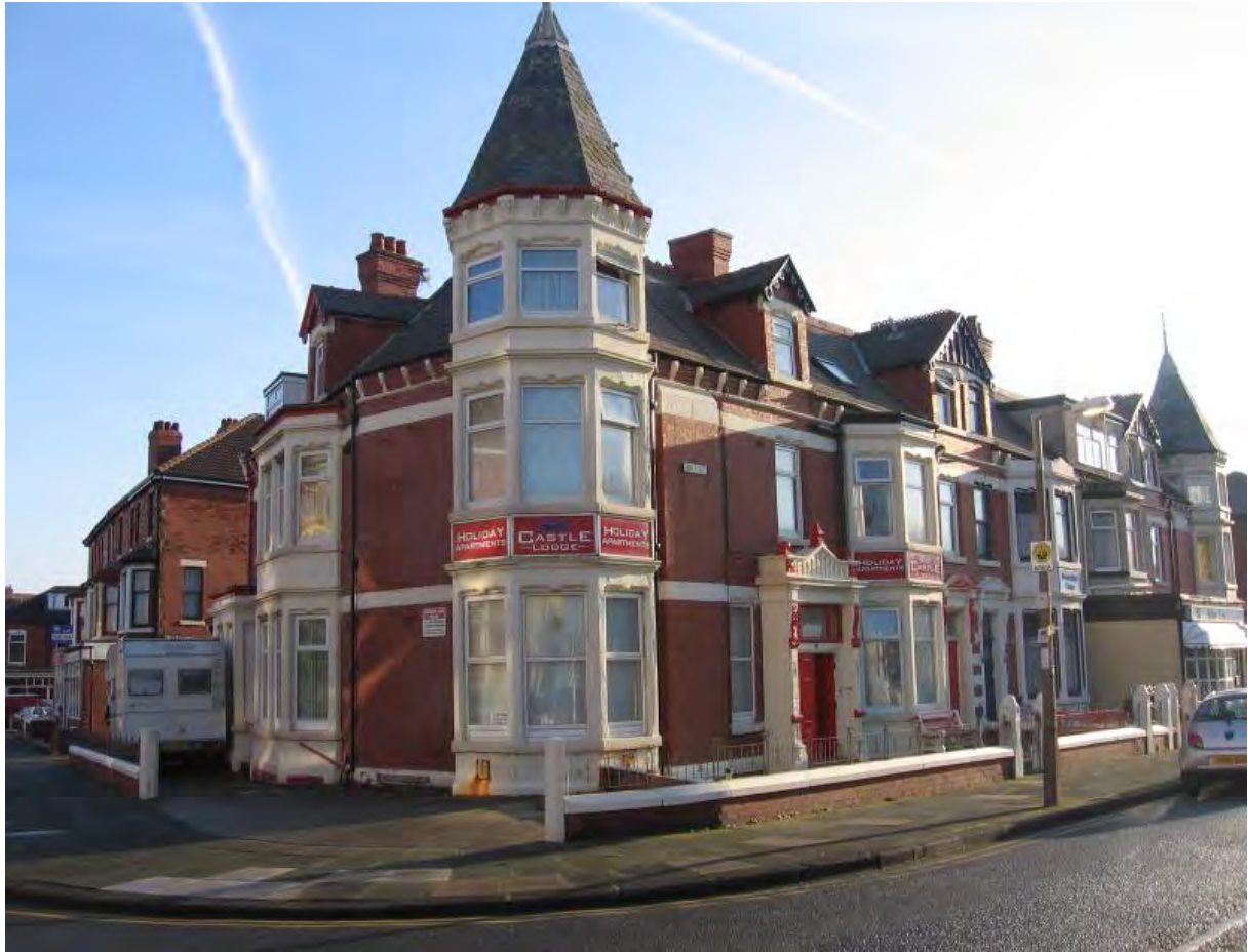
Fig.72: Rich corner detailing at No. 99 Lord Street, built c.1900
