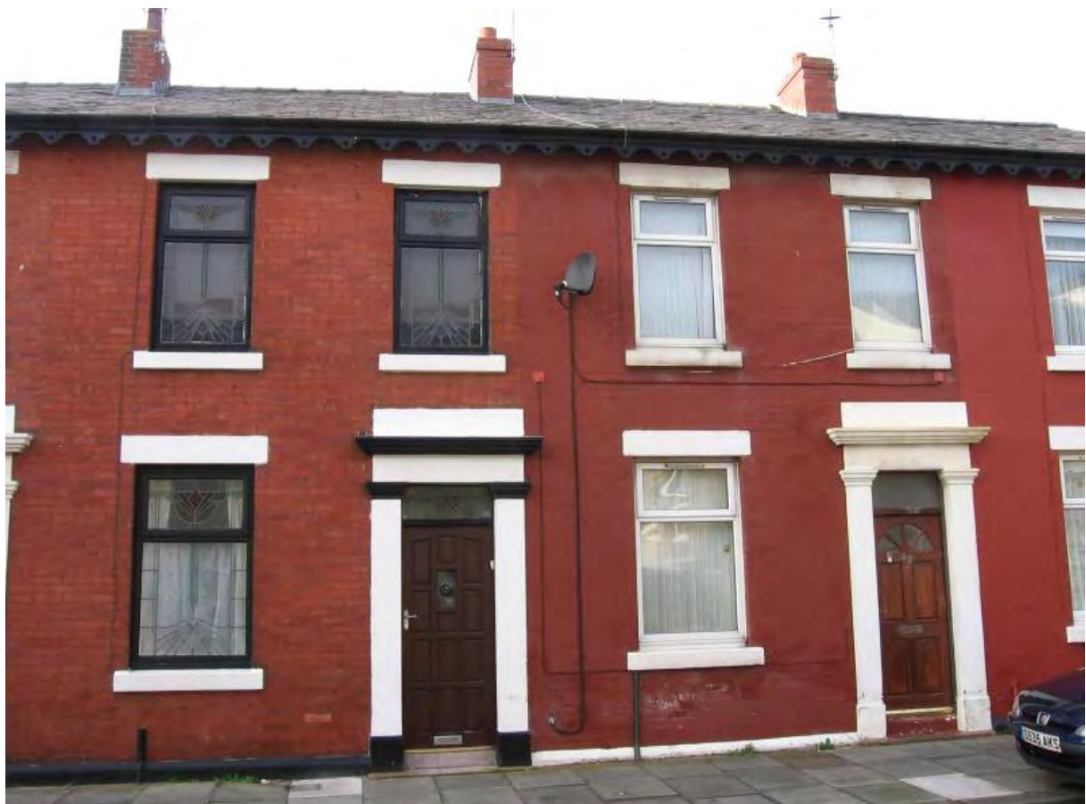
Fig.38: Plain workers' housing on Richmond Road, built c.1900
