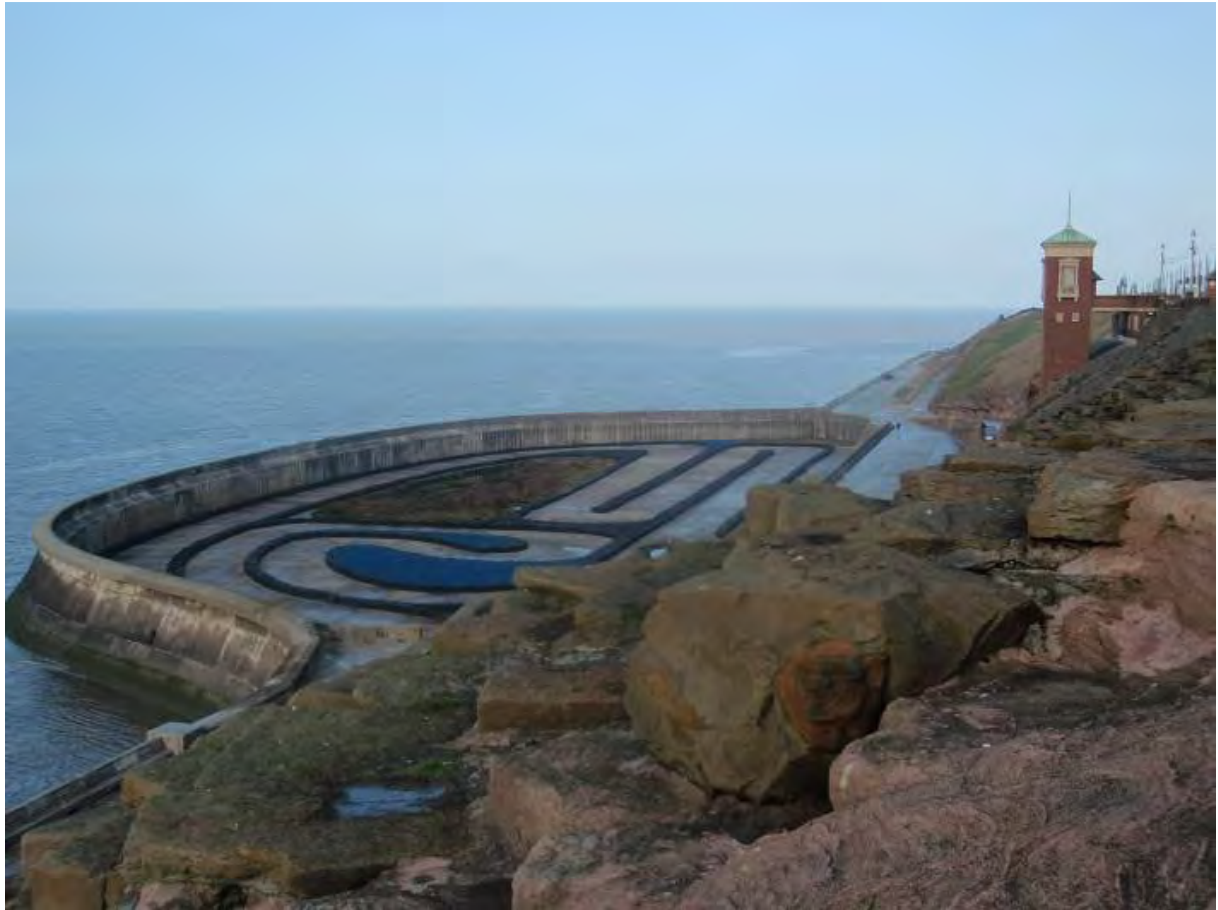
Fig. 39: The artificial cliffs, cabin lift and former boating pool off North Promenade
