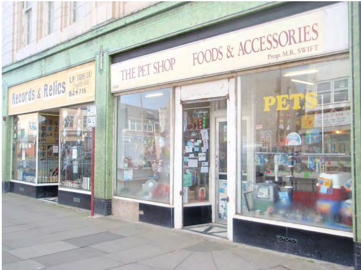
Fig.23: Shopfronts to Cauce Street
