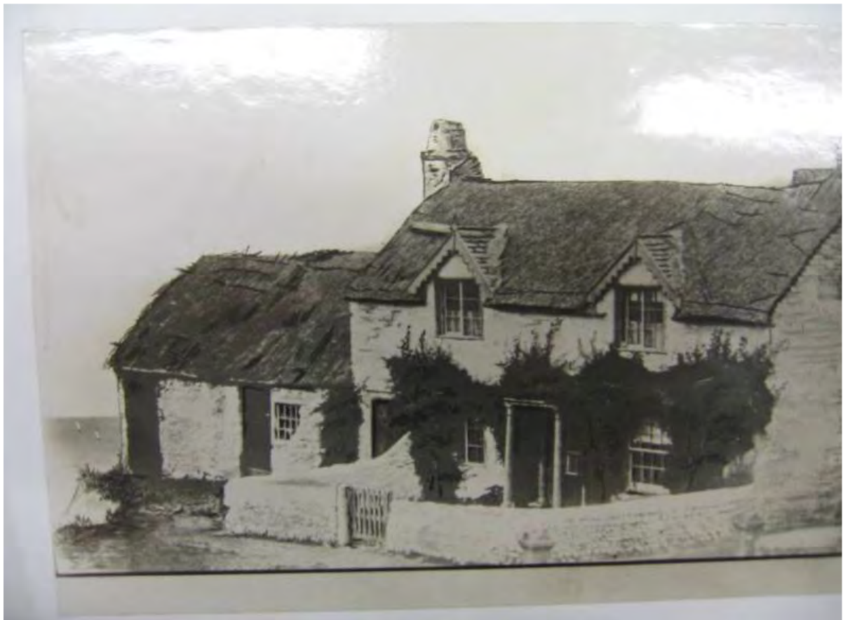
Fig.3: Cliff Cottage at Fumblers Hill, now Cocker Square, was demolished c.1865 for improvements to the promenade (Blackpool Library)
