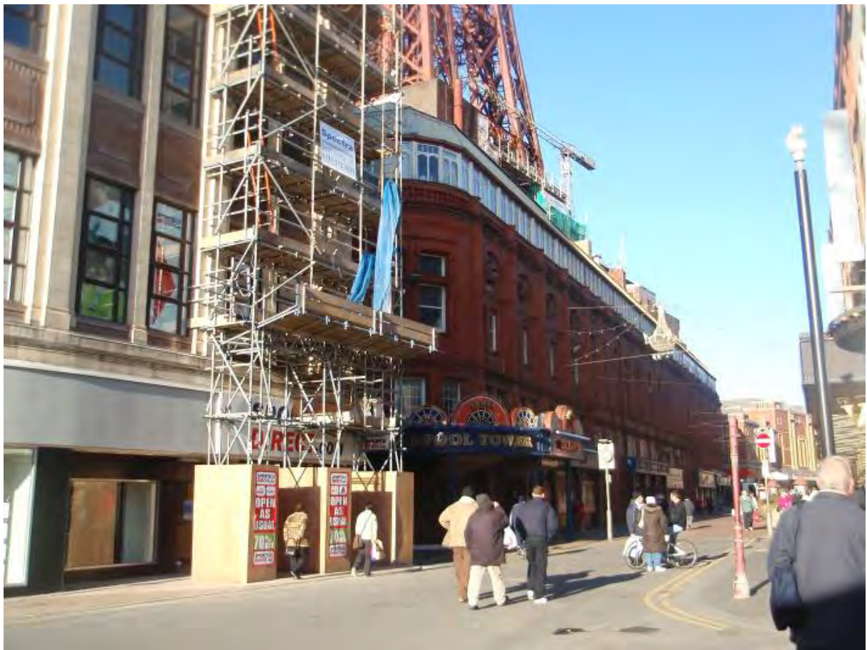
Fig. 54: The east side of Tower Buildings on Bank Hey Street
