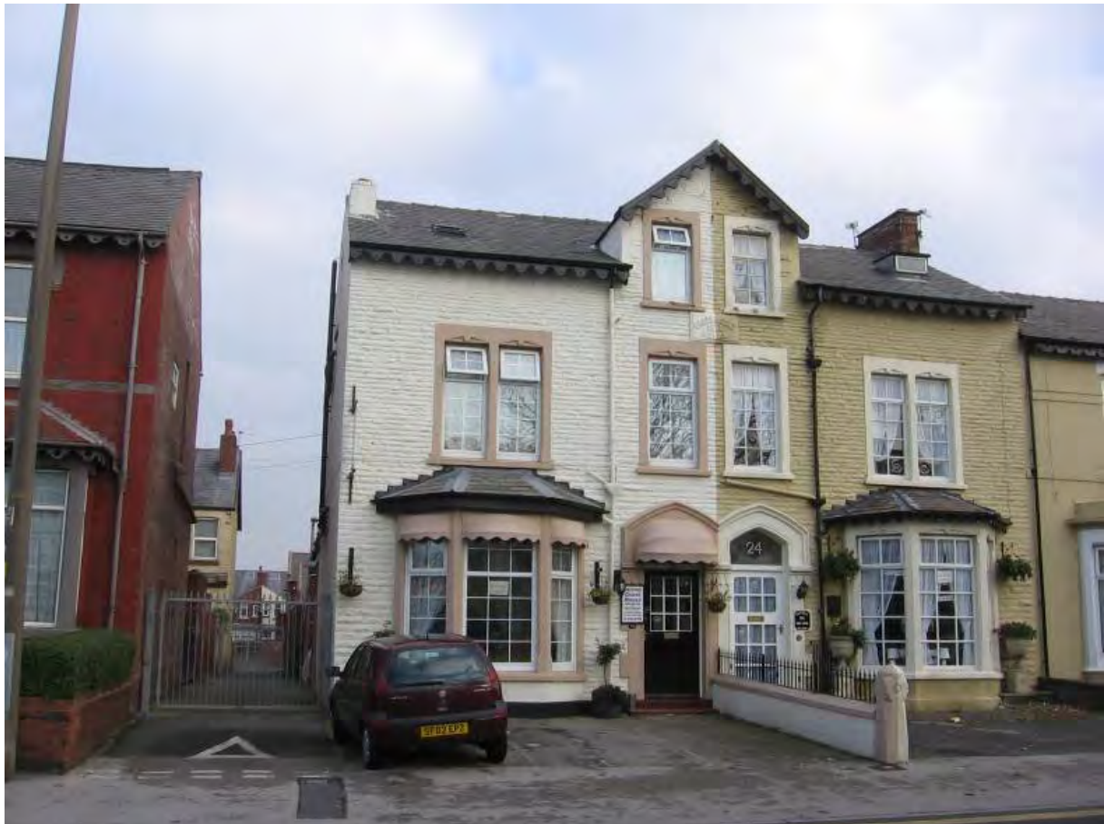
Fig. 67: Greenmount Villas, Park Road
