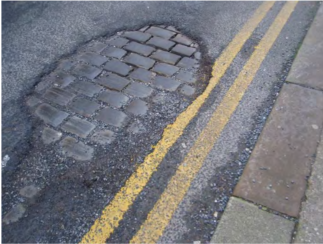
Fig.33: Stone setts showing through worn tarmac on a side street of Abingdon Street
