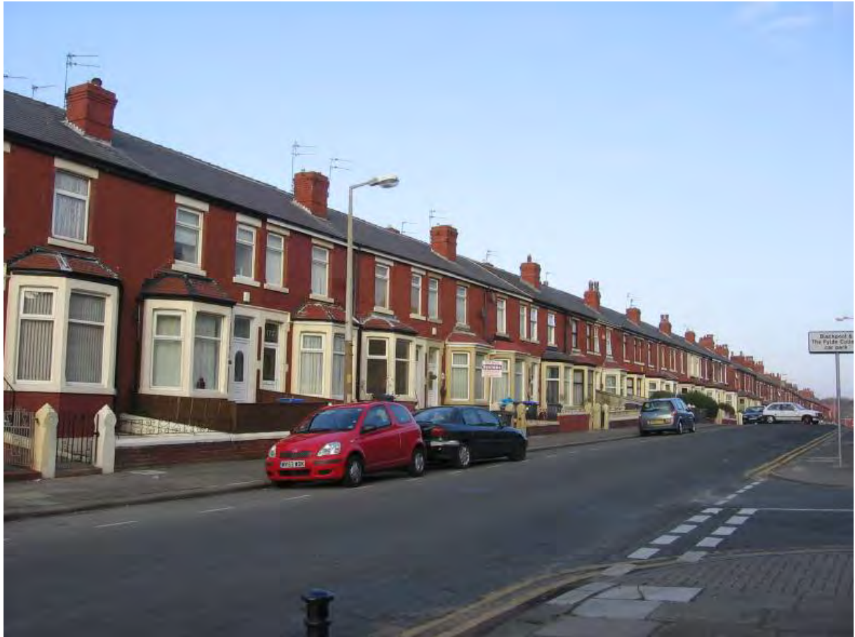
Fig. 20: Long framed views along Palatine Road
