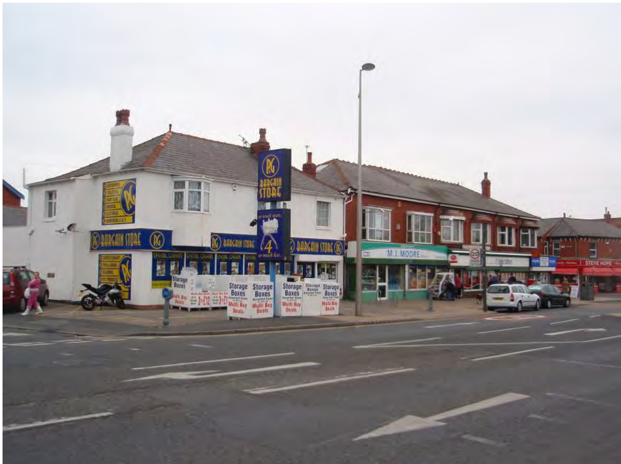
Fig. 38: Intrusive signage to Nos 37-51 Westcliffe Drive
