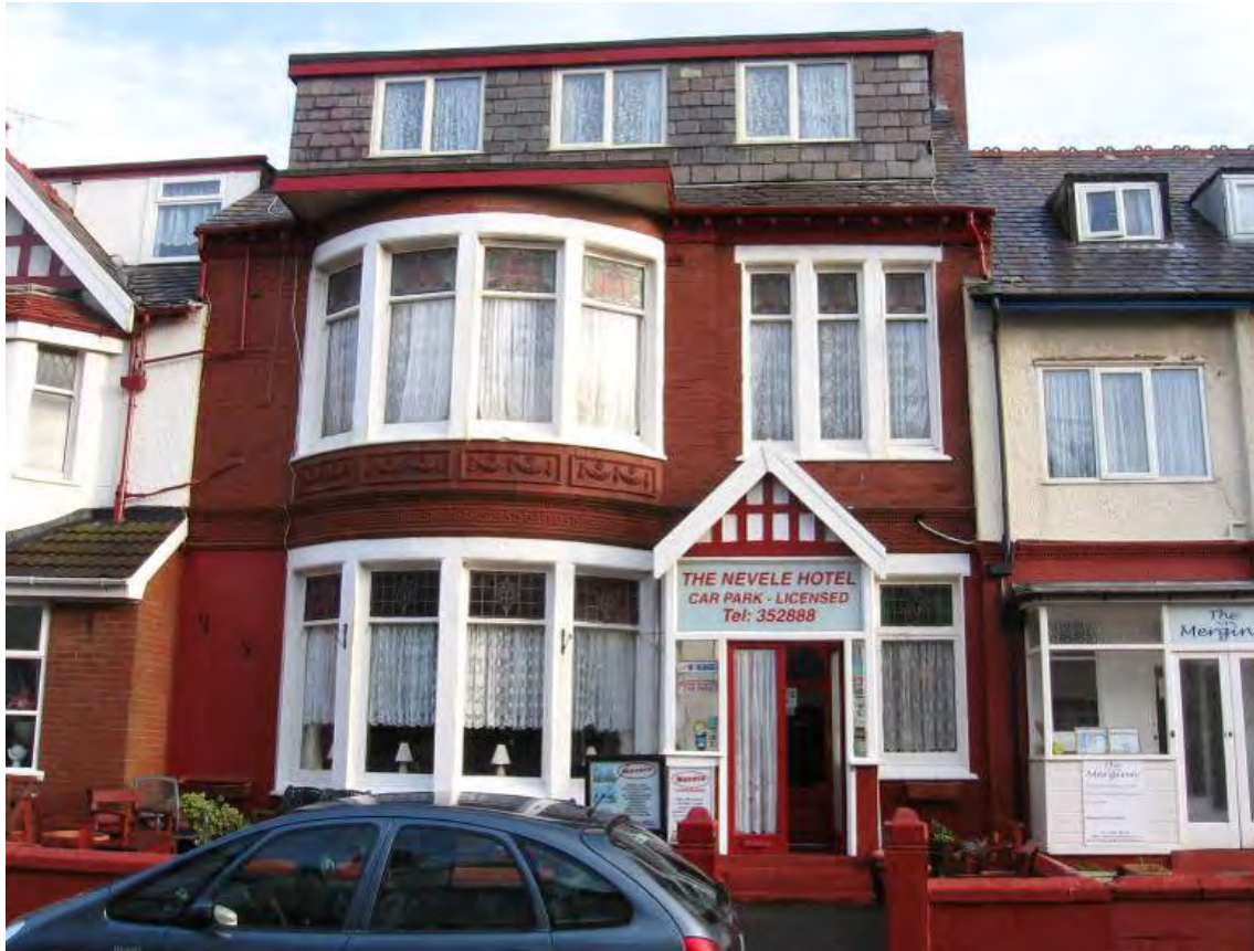
Fig. 44: Leaded casement windows and added attic dormer on a Gynn Avenue hotel
