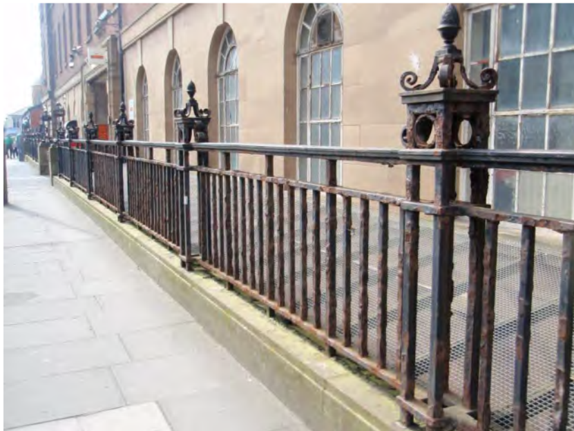
Fig. 69: Wrought iron railings to the rear of the post office
