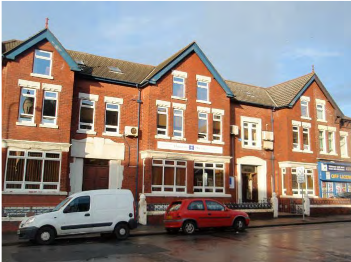
Fig.52: Nos. 4-12 on the north side of Springfield Road
