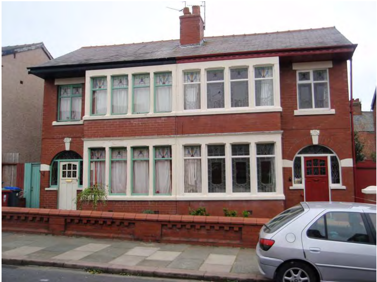
Fig.34: Original windows and glazing, and doors, at Nos 22-24 North Road
