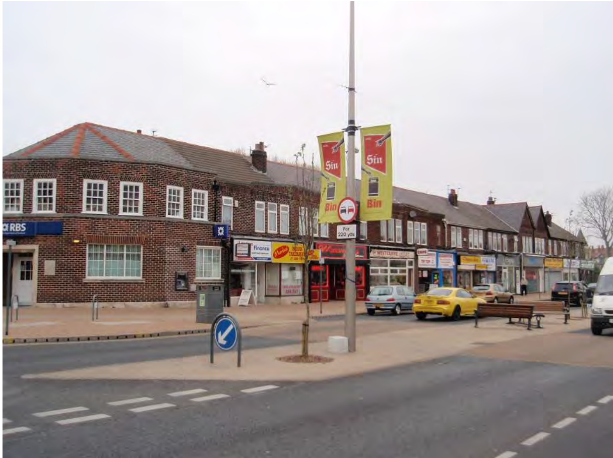
Fig. 116: Nos 2-28 from the south
