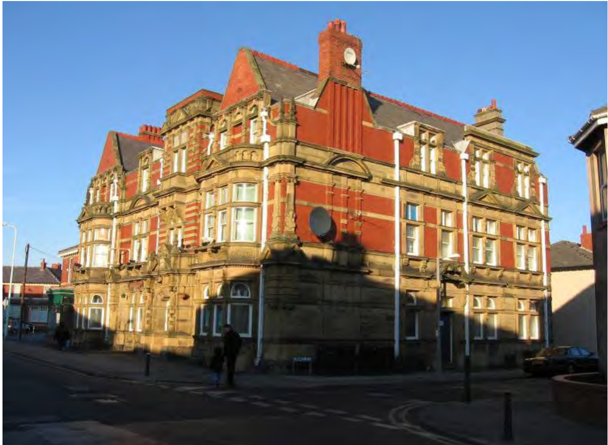
Fig 76: The Empress prior to painting of stonework
