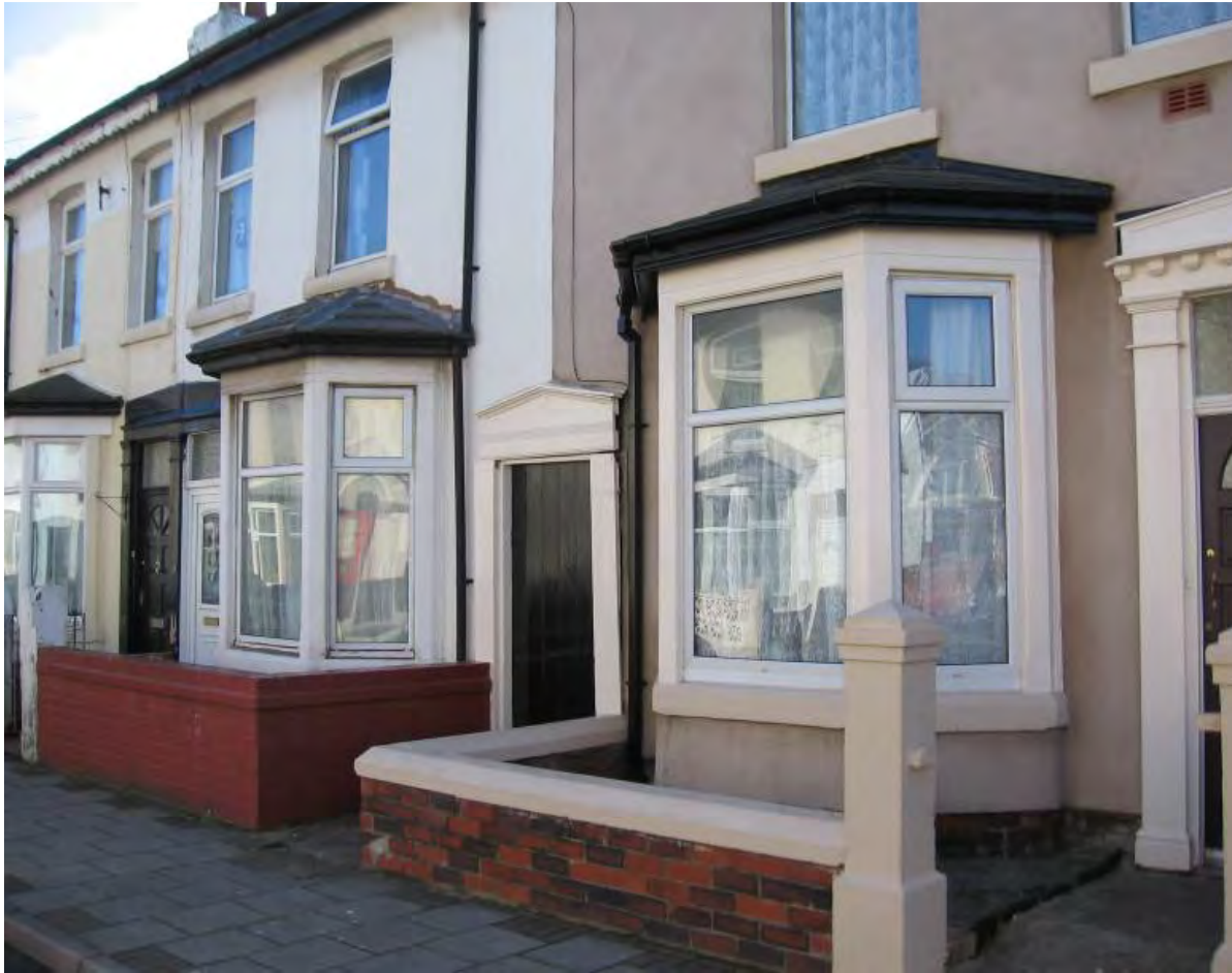
Fig.9: Duke Street, one of the earliest terraced streets, with plain stone details for bays and doorways
