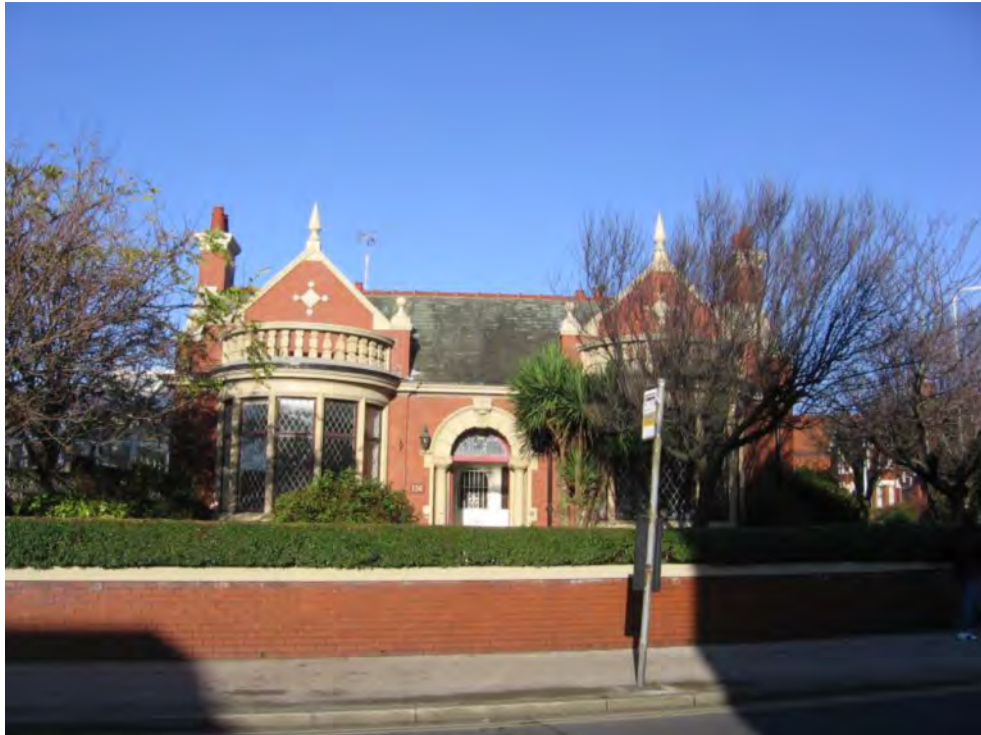
Fig. 29: No. 136 Hornby Road: stone bays and dressings
