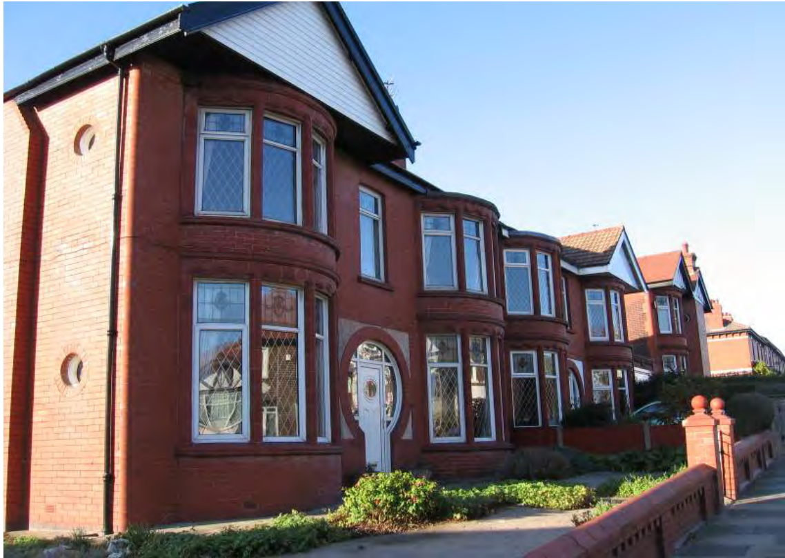
Fig. 93: Nos. 43-45 – large semi-detached houses towards park.
