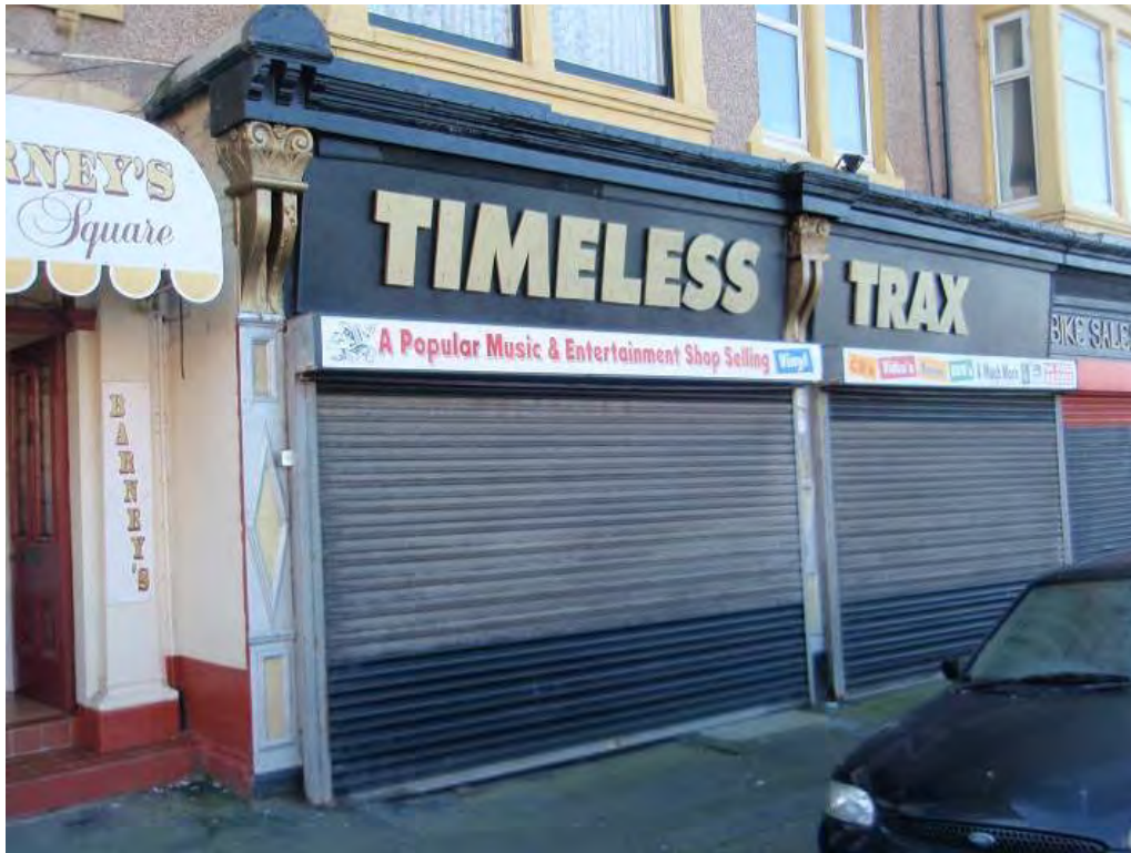
Fig. 20: Timber shopfront to the south side of Cocker Square.
