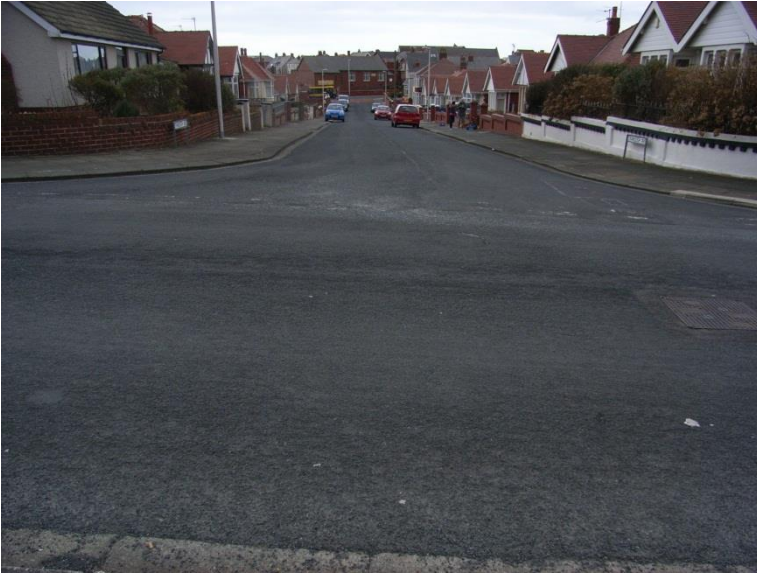
Figure 26 Cranleigh Avenue from Countess Crescent
