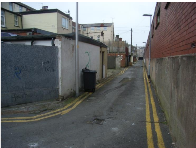
Figure 55 Rear of properties on Lonsdale Road
