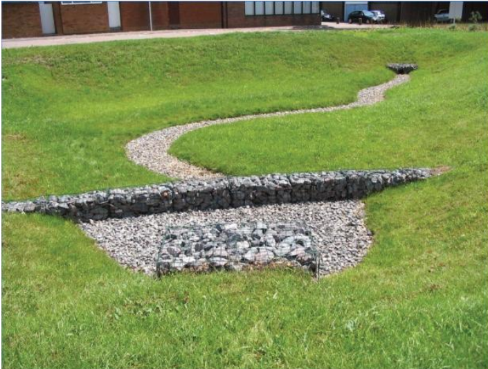
Figure 4 Example of a detention basin - 'Sustainable Drainage - Retrofitting the Built Environment' by Arup
