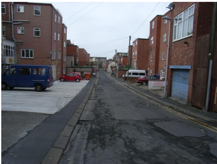
Figure 48 Rear of properties between Albert Road and Charnley Road
