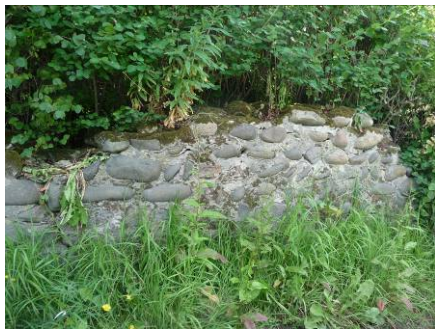
Plate 11. A piece of surviving cobble wall on Chapel Road
