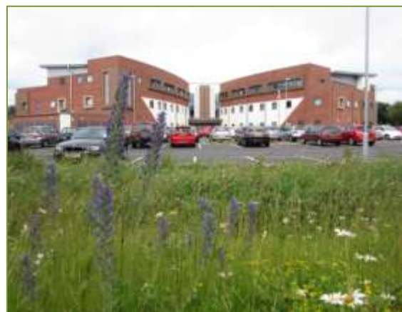
SuDS scheme at Moor Park
