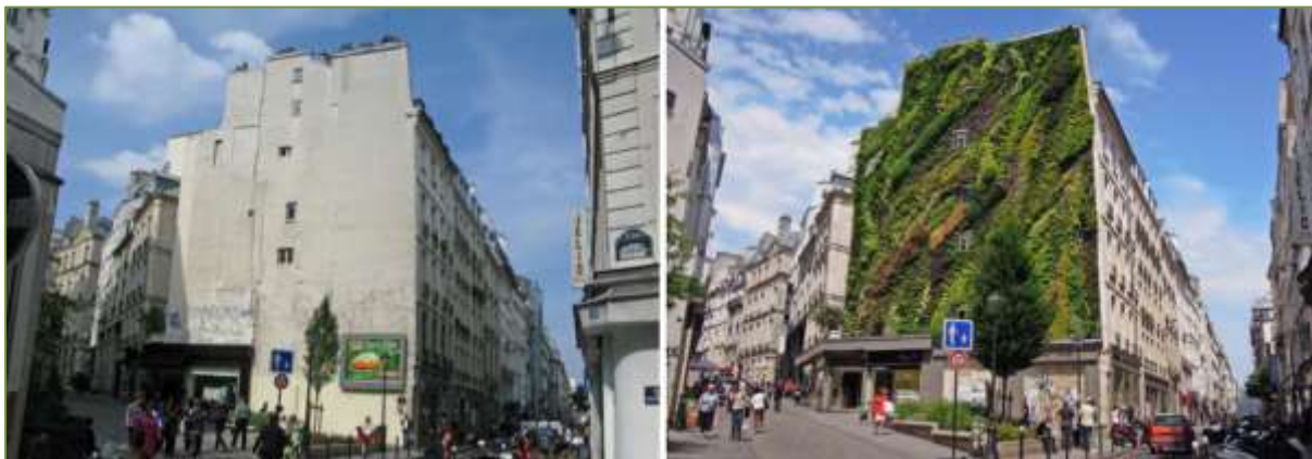
Retrofitted green wall in Paris
