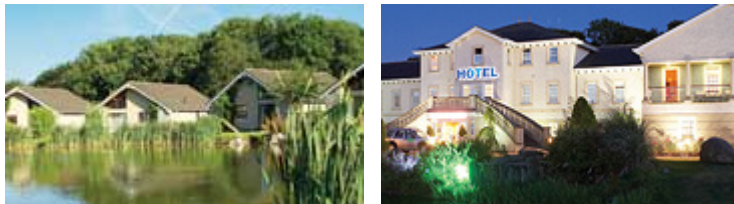
Figures 7.8 & 7.9: Built Cottages & Hotel at Ribby Hall Village
