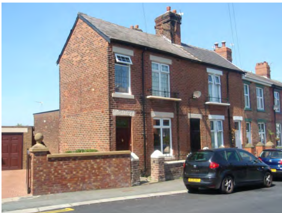
Fig. 132: Nos 158-160 Layton Road
