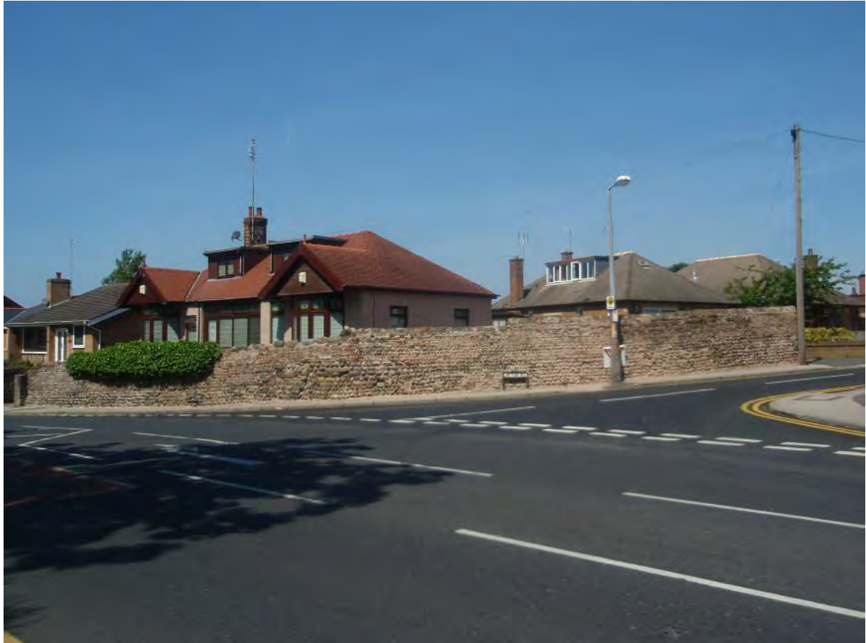
Fig. 133: Cobble wall at the south-west end of Layton Road, with an interwar bungalow behind
