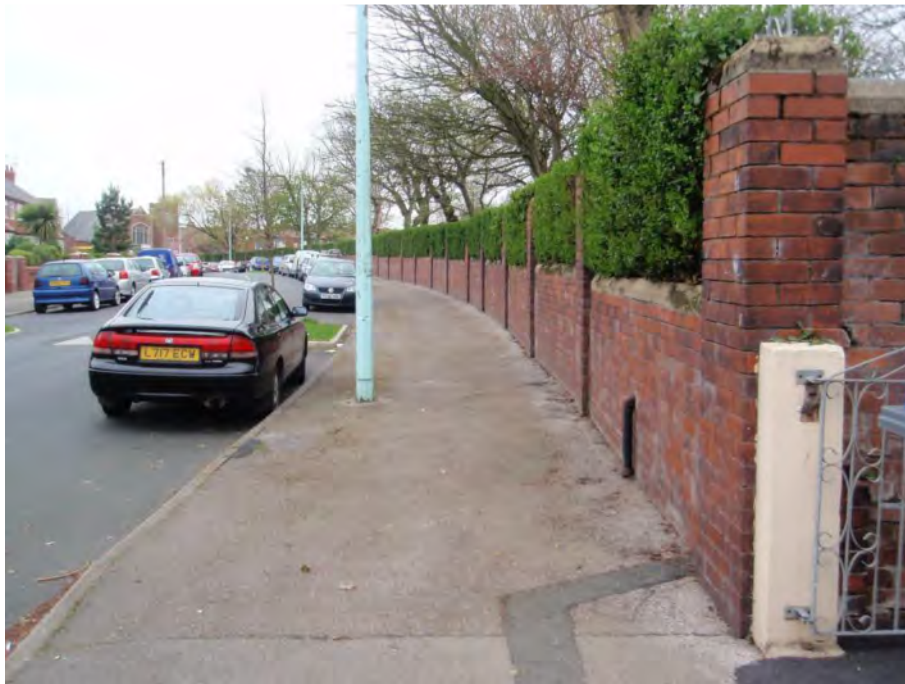
Fig. 52: Boundary wall and hedge to Layton Cemetery, on Annesley Avenue.
