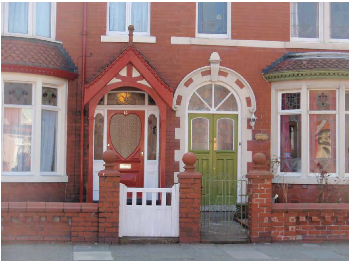
Fig. 37: Timber canopies to Nos 12-14 Grange Road
