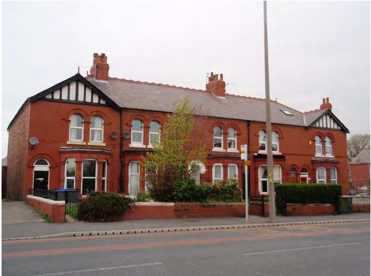
Fig. 128: Nos 273-281 Talbot Road
