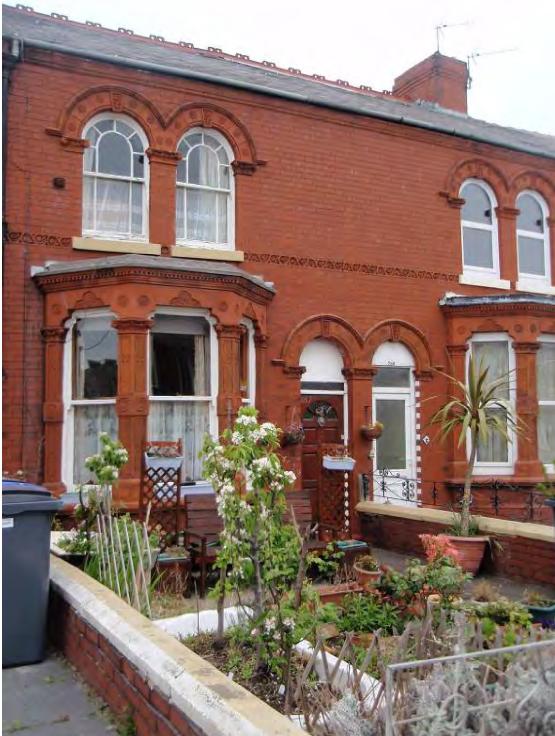
Fig. 48: Terracotta decoration to terraces on Talbot Road
