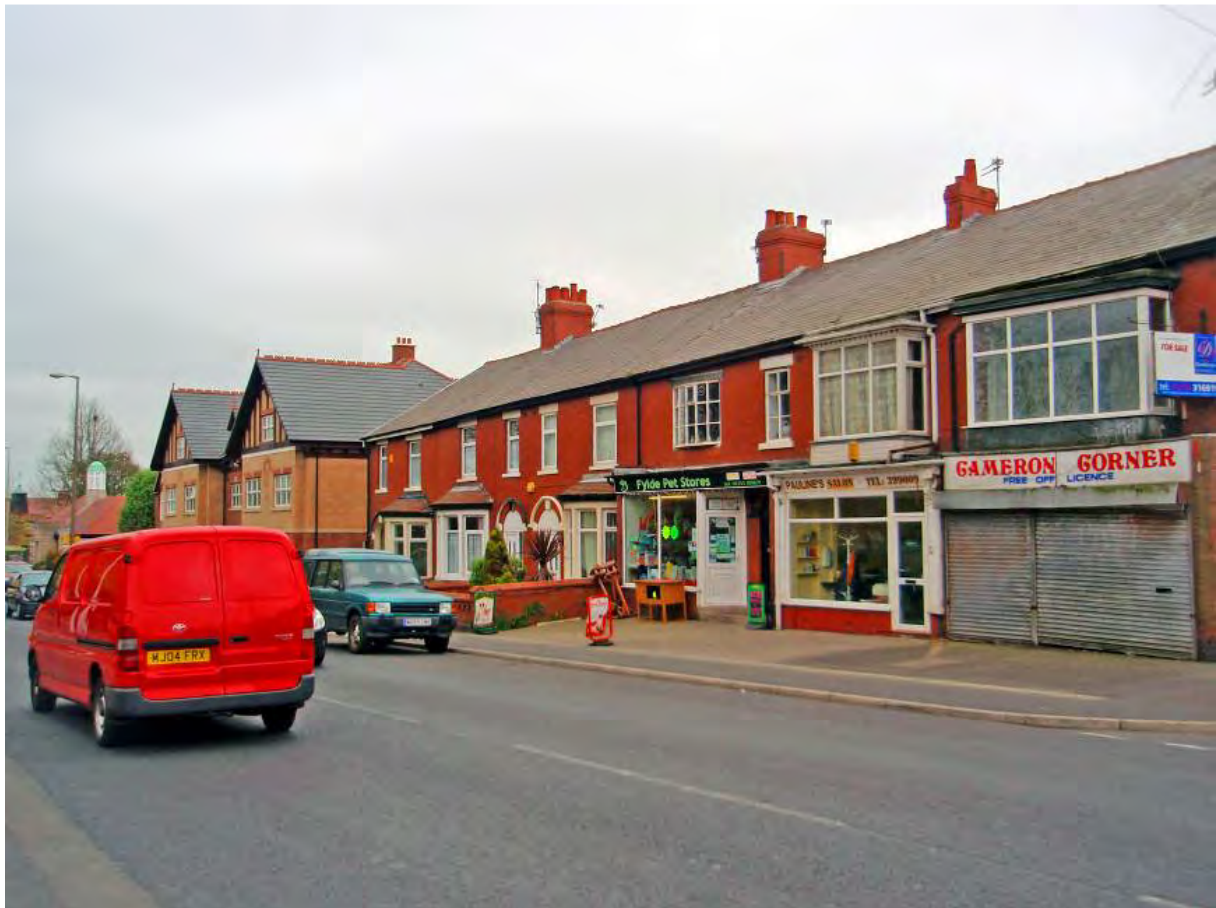
Fig. 54: Nos 460-470 Talbot Road have their front boundary walls removed
