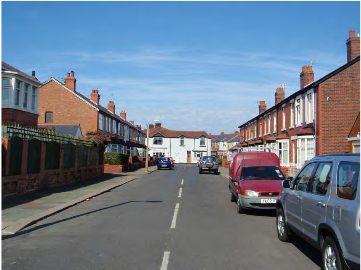
Fig. 88: Looking west down Alder Grove
