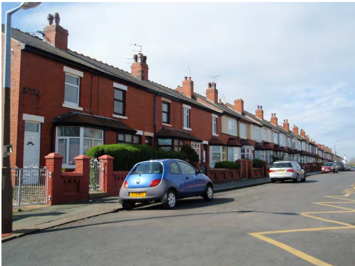
Fig. 79: The south side of Lynwood Avenue, from the east
