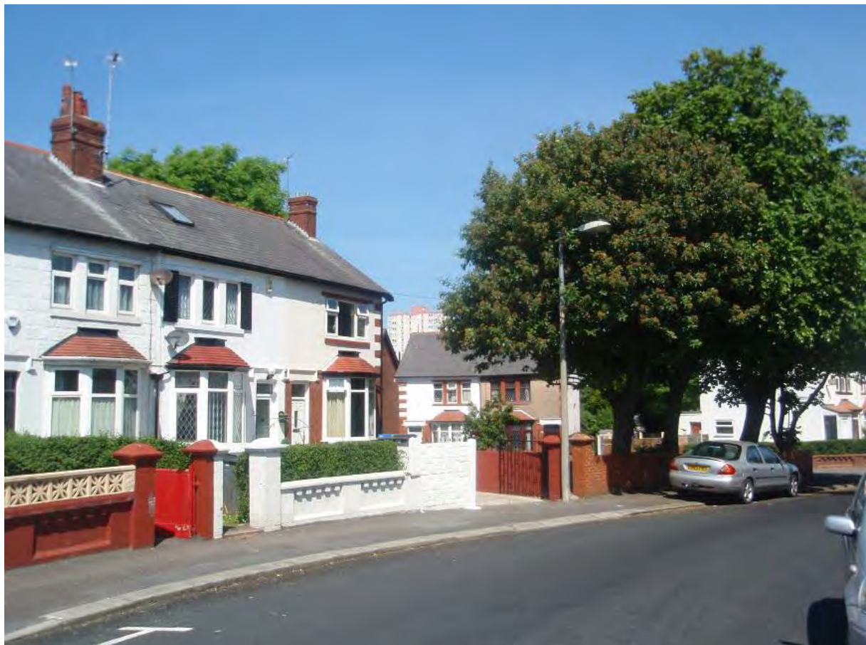
Fig.130: Nos 112-118 Layton Road
