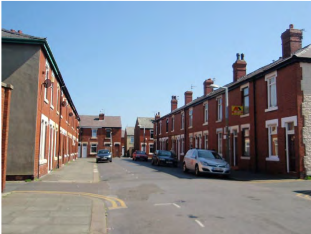
Fig. 94: Huntley Street, looking east
