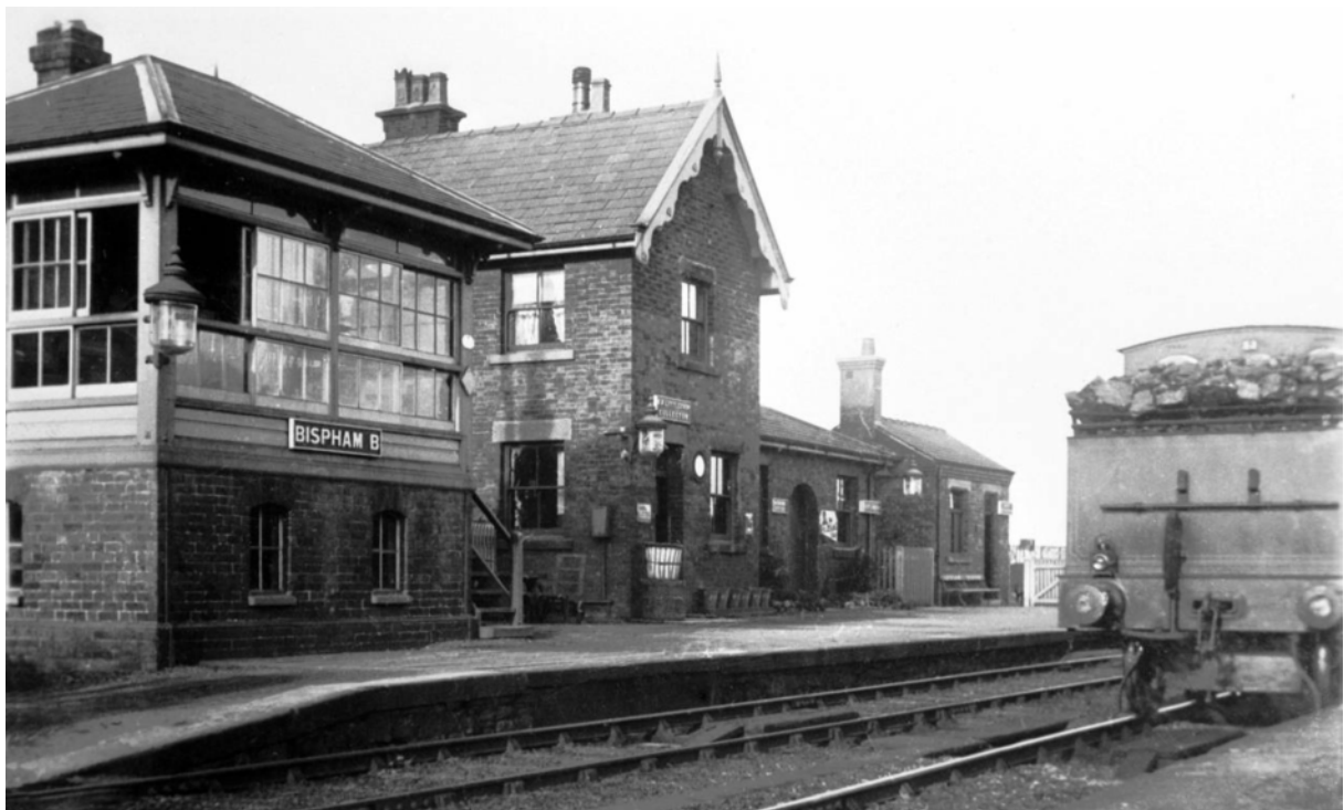
Fig. 6: Bispham (now Layton) Station in the early 20 th -century; the station house and adjacent single-storey buildings are still extant (courtesy Ted Lightbown).
