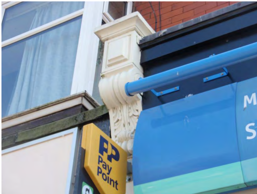
Fig. 40: Part of a historic shop front on Layton Road, possibly part of the original Co-op store. Two good examples of shopfront design can be seen at No. 1 Layton Road (Ragamuffins) and the RBS Bank at Nos 2-6 Westcliffe Drive. The former retains its timber cornice and pilasters, and the colour scheme, signage and retained corner
