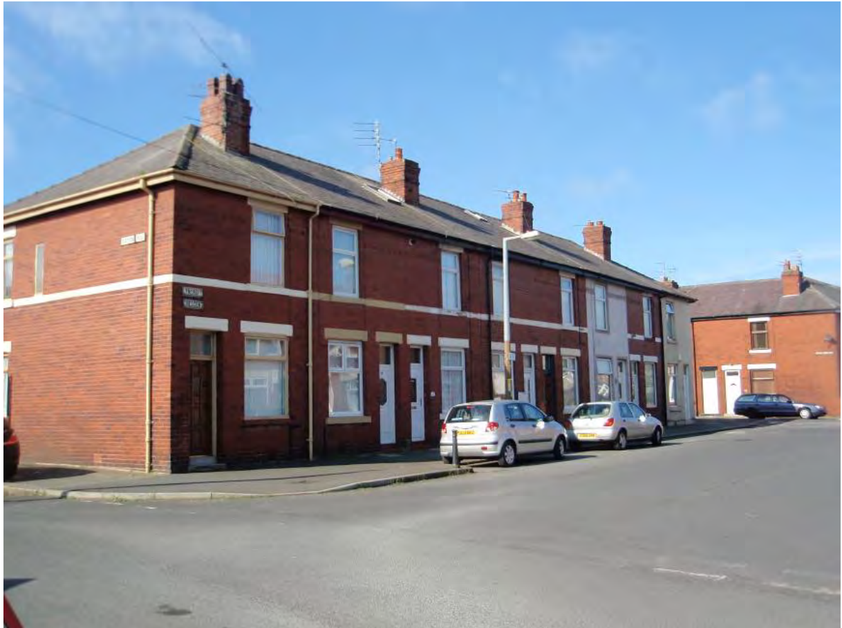
Fig. 100: Nos 6-20 Lyncroft Crescent
