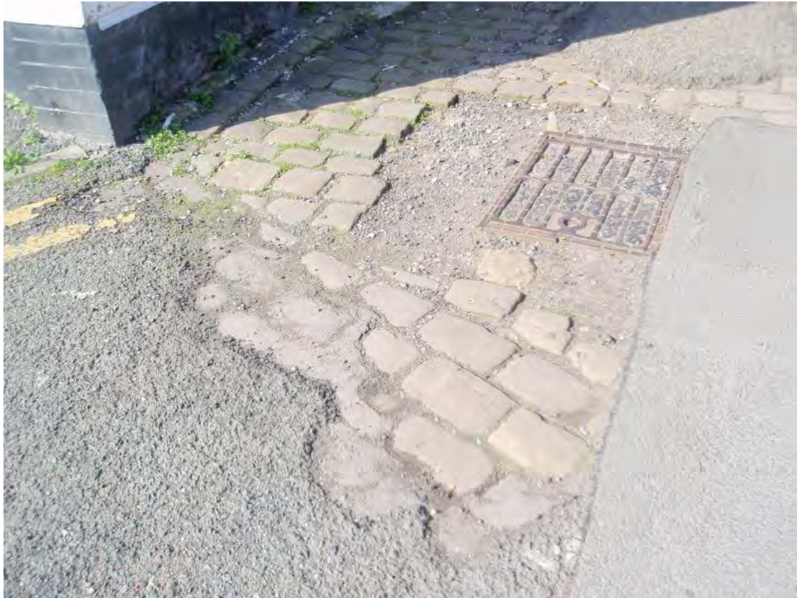
Fig. 56: Setts below tarmac on Alder Grove
