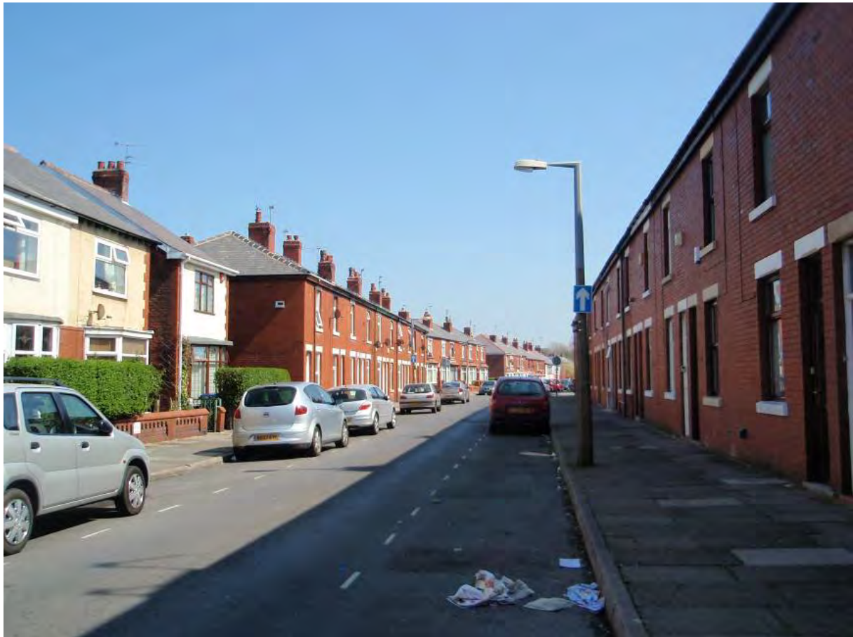
Fig. 93: North side of Grenfell Avenue, looking east
