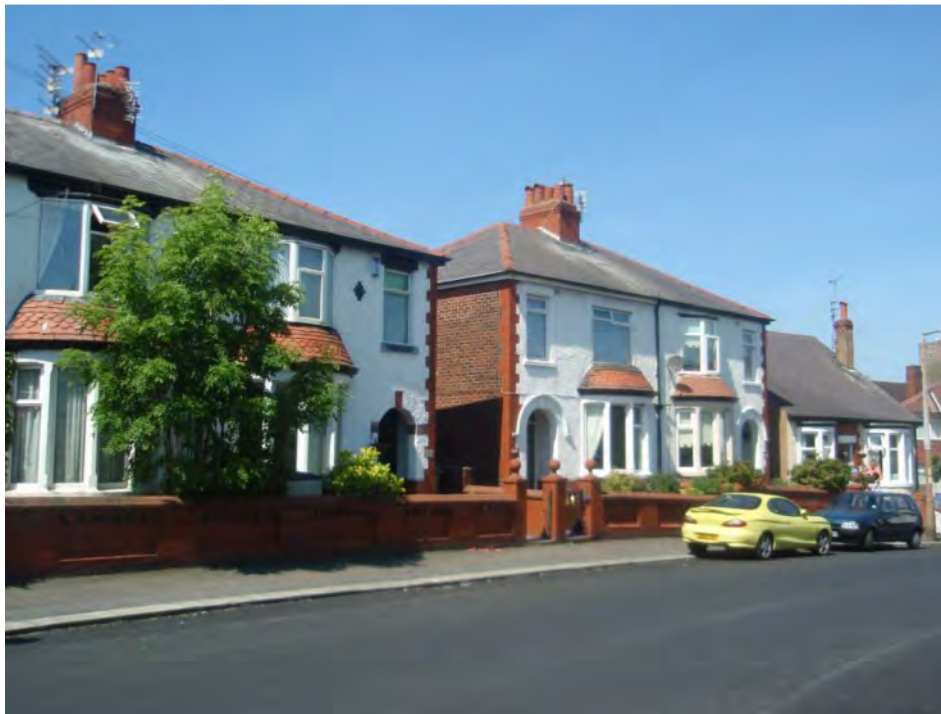
Fig. 131: Nos 128-136 Layton Road
