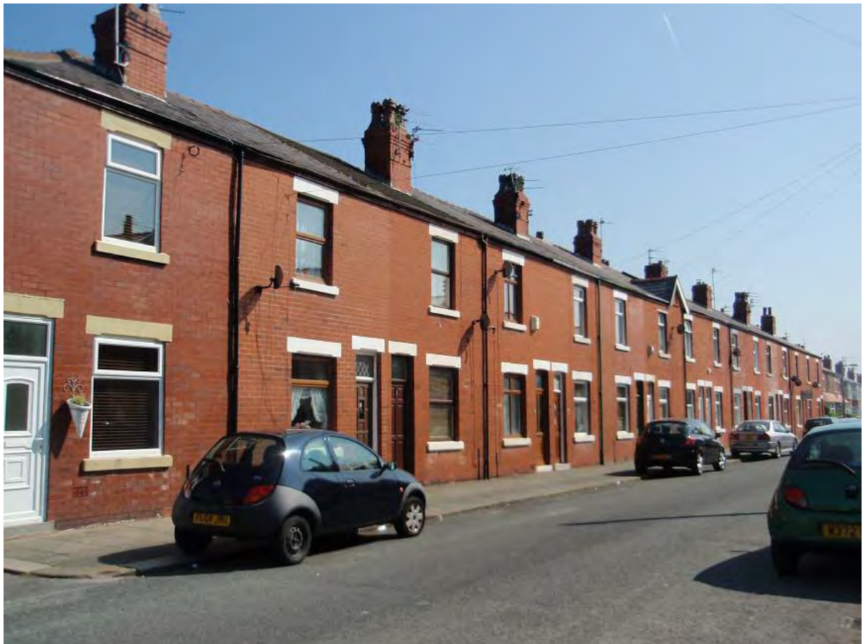
Fig. 27: The north side of Rathlyn Avenue, punctuated by a small gable
