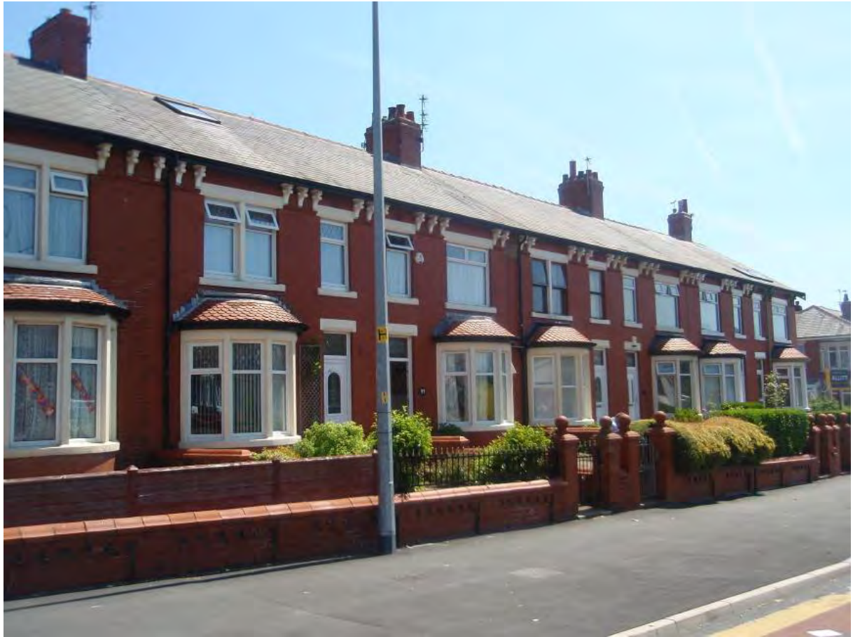
Fig. 138: Nos 89-103 Layton Road
