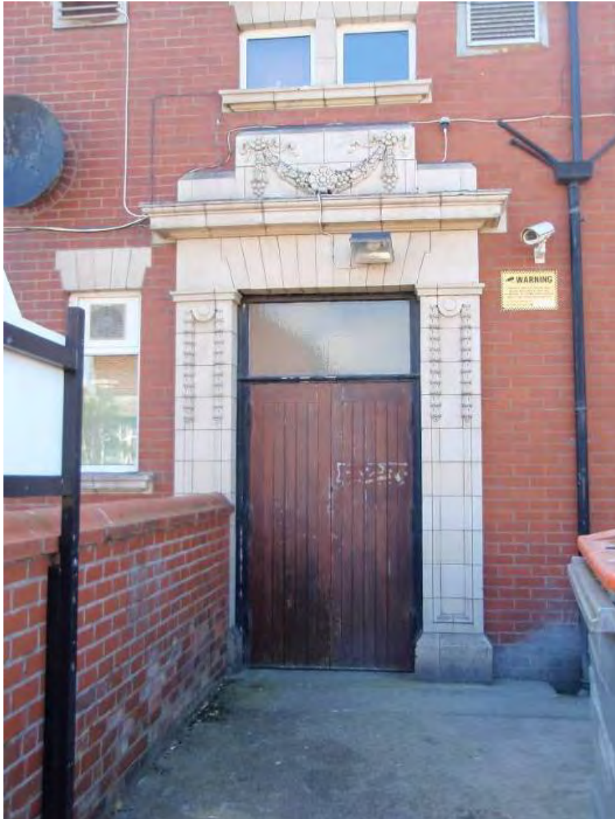
Fig. 29: Buff faience to the Granby Avenue entrance to Layton Institute
