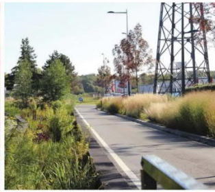
Swale buffer planted
