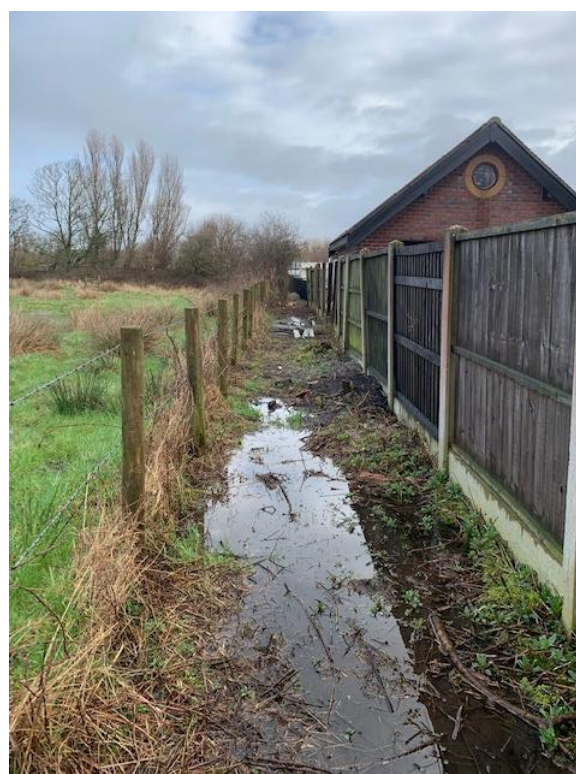
Photo 16: Footpath 50 showing flooding
