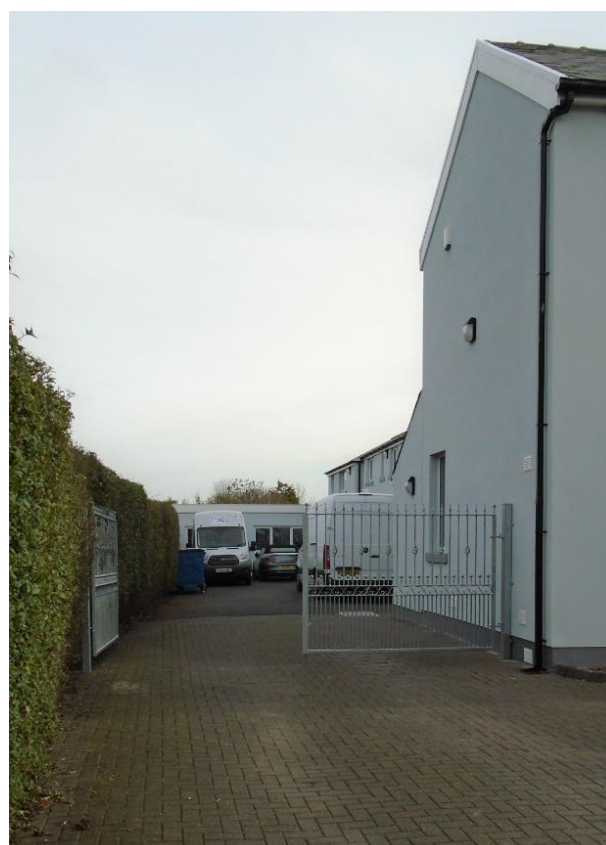
Photo 14: Footpath 49 partially blocked by building off Midgeland Road
