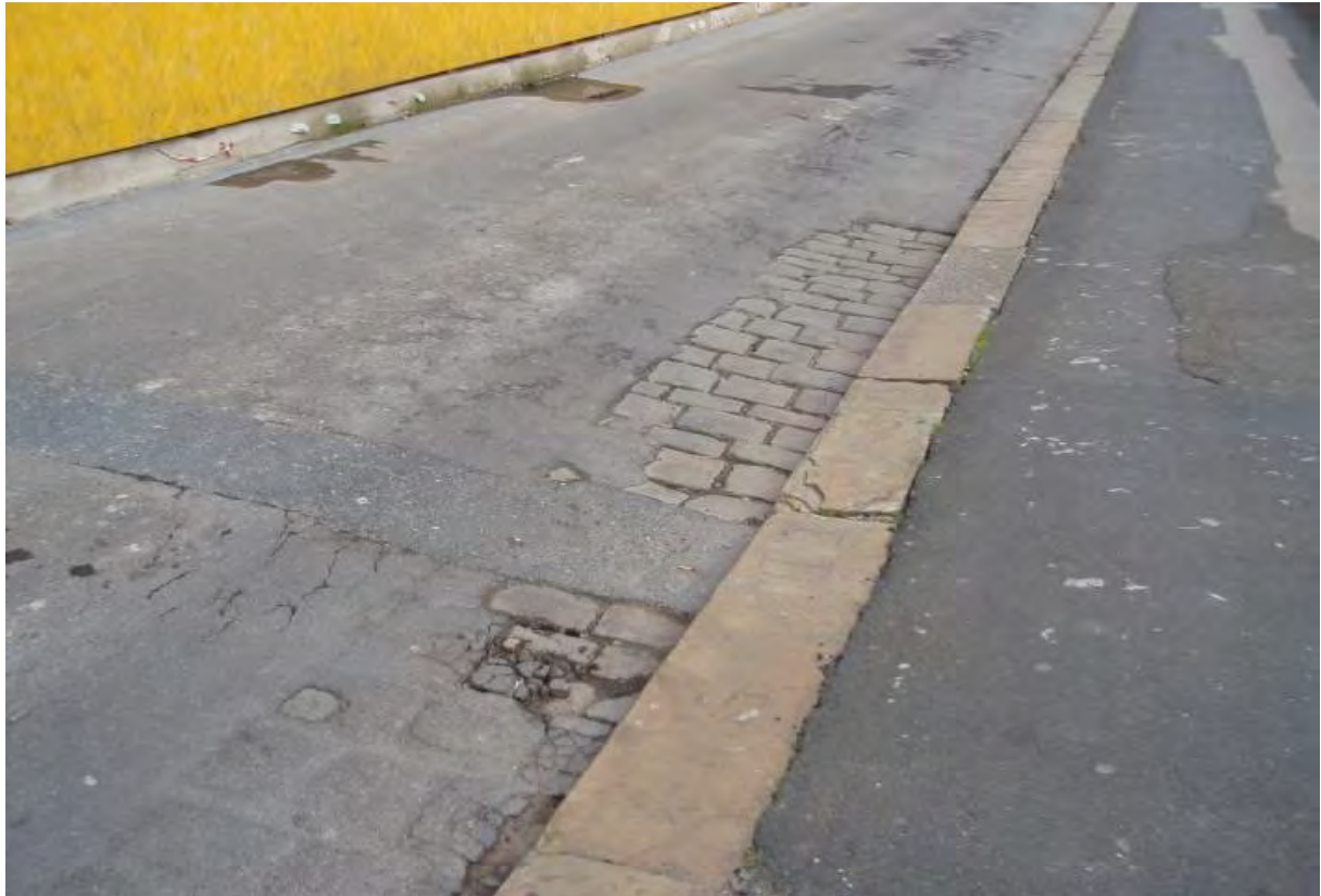
Fig. 40: Stone kerbs and setts, below tarmac on Balmoral Road
