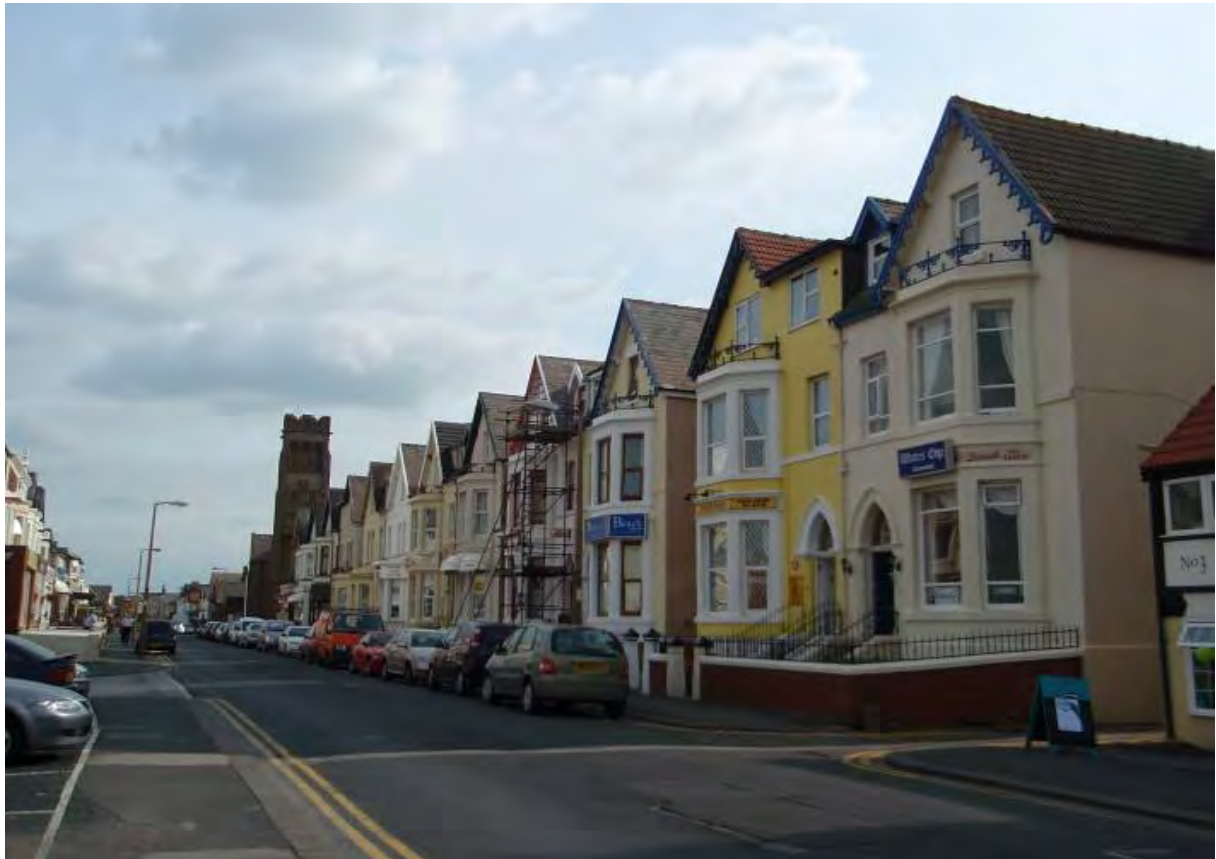
Fig. 23: Timber barge boards to boarding houses on the south side of Dean Street
