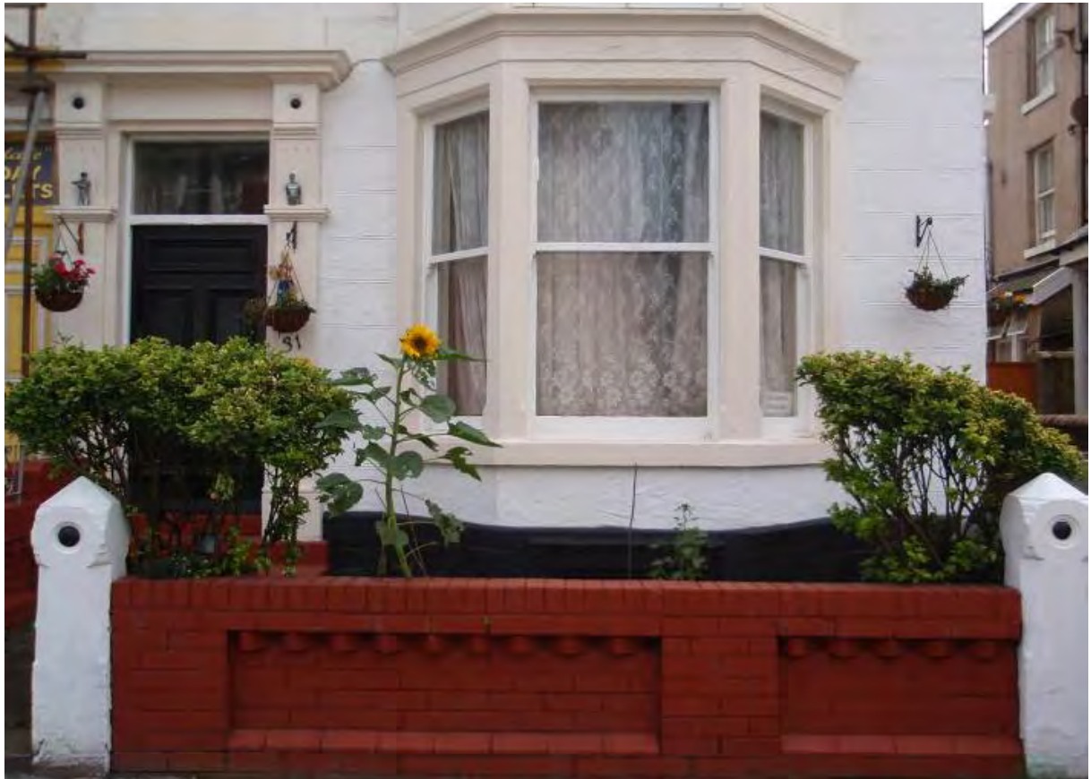
Fig. 24: Sash windows and panelled door on a property on Osbourne Road.
