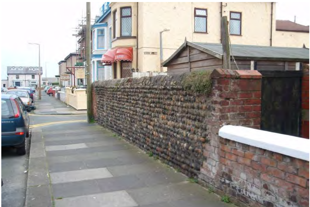
Fig. 37: Traditional cobble wall on Rawcliffe Street
