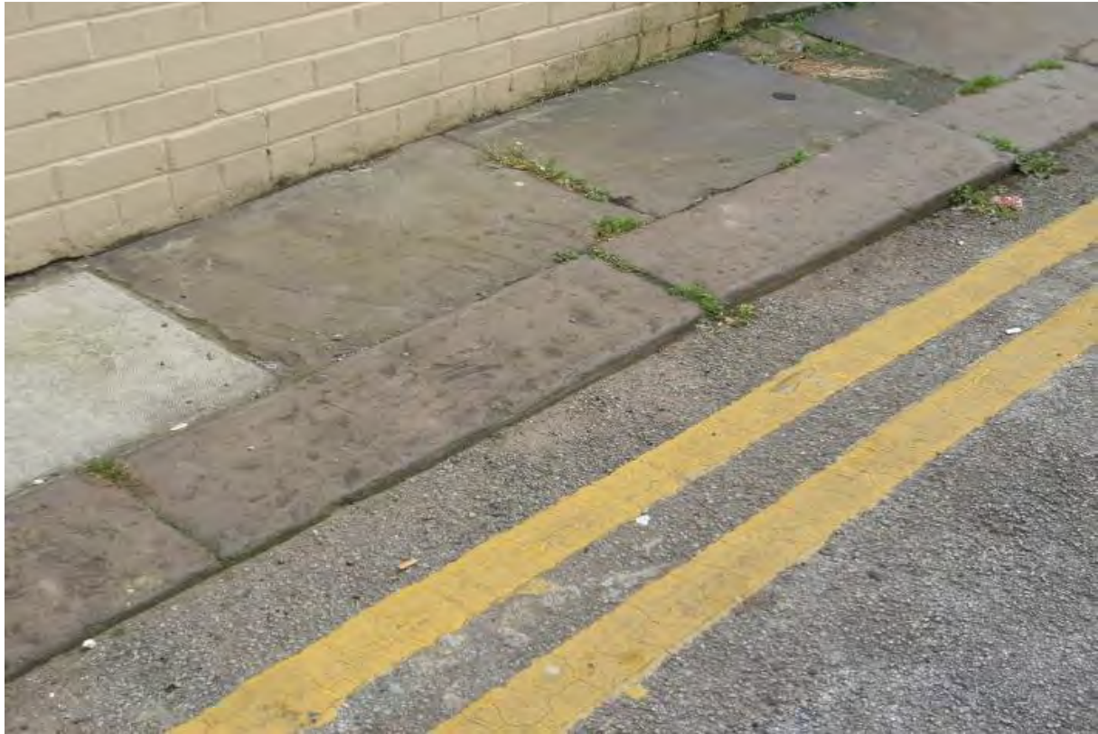
Fig. 42: Natural stone paving and kerbs on Byron Street
