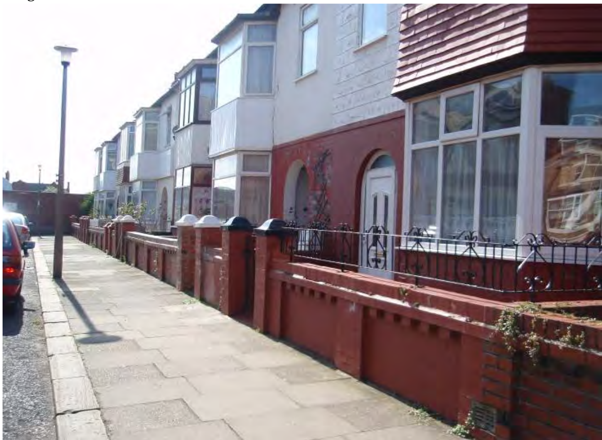
Fig. 36: Intact interwar brick boundary walls on Brighton Avenue
