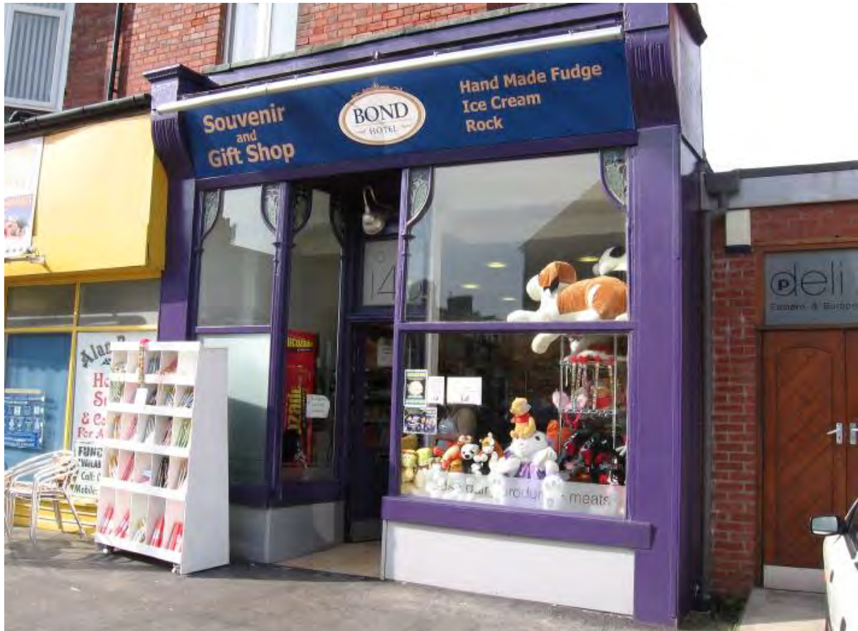
Fig. 30: Early 20 th -century timber shopfront at No. 145 Bond Street
