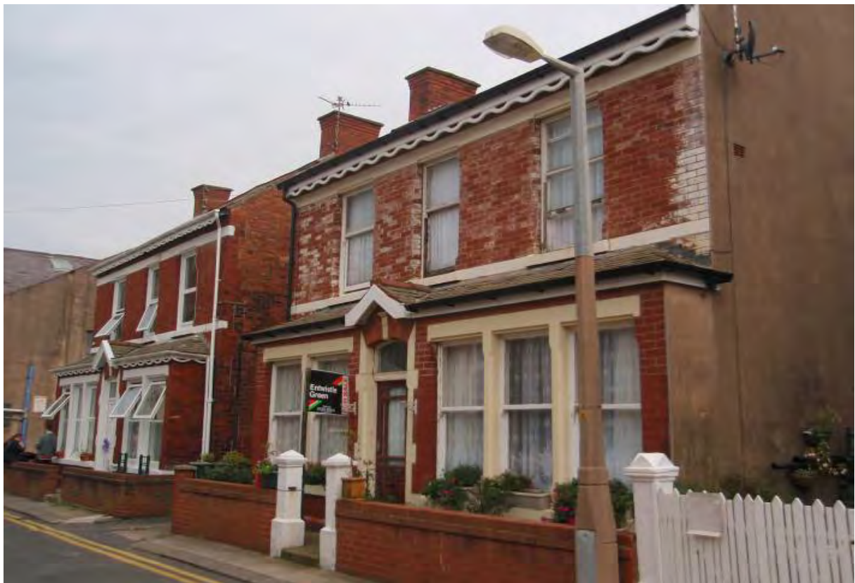
Fig. 45: Sash windows, exposed brickwork and decorative eaves cornice to a property on Byron Street
