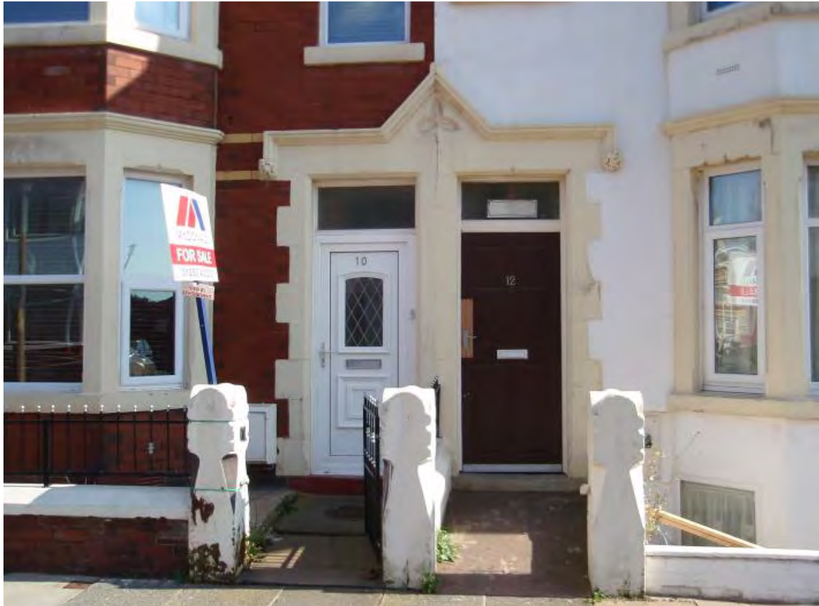
Fig. 27: Gothic paired entrance details on Brighton Avenue
