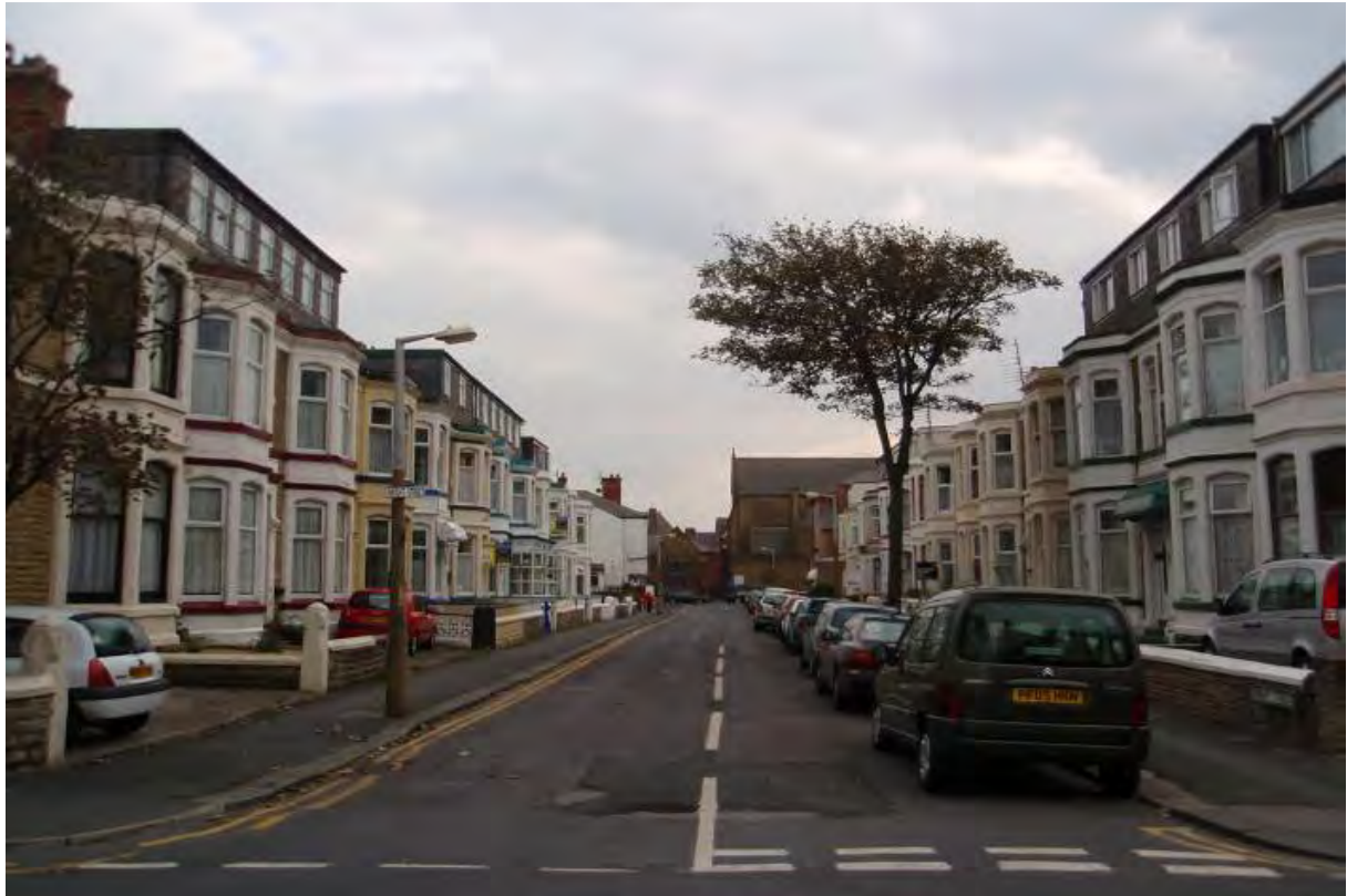
Fig. 13: View looking south down Bright Street from Rawcliffe Street
