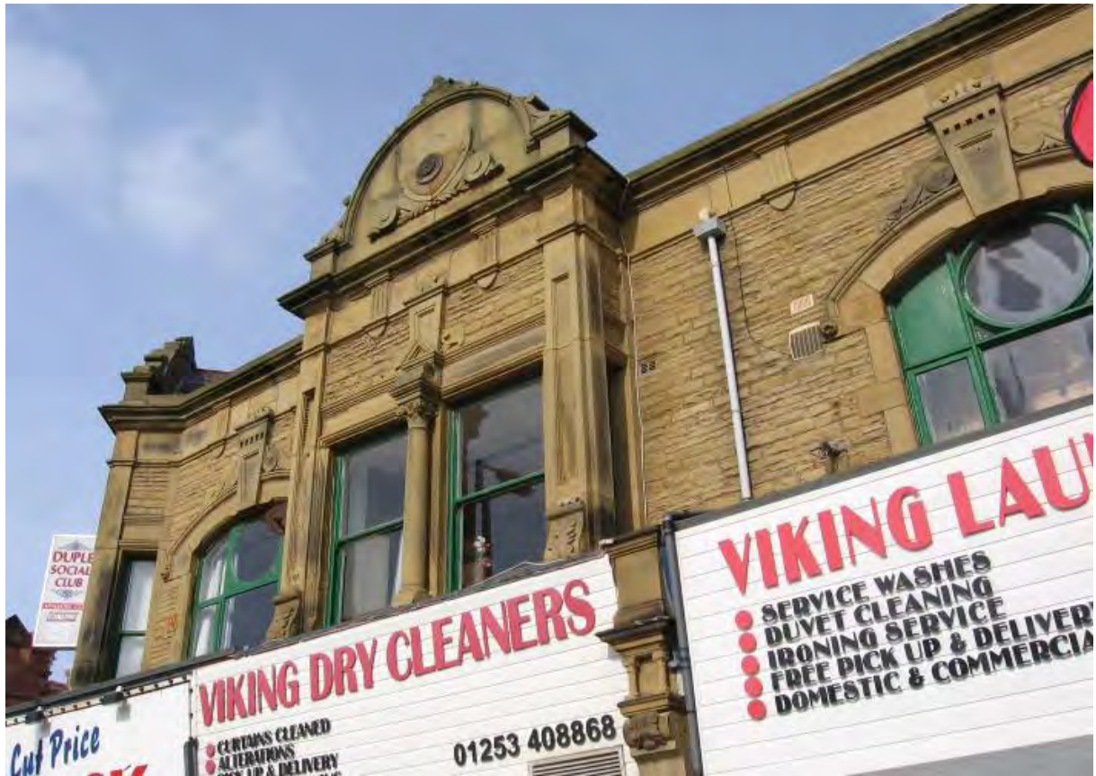
Fig. 18: South elevation of 33-36 Station Road
