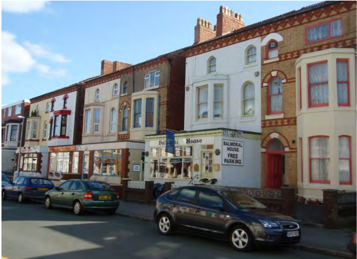
Fig. 21: Contrasting treatments to a row of boarding houses on Withnell Road; the house to the right retains original yellow brick with red brick details; other houses been rendered and painted.
