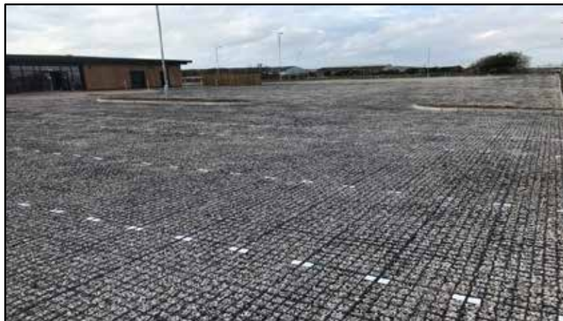
Image Seven: New Car Park featuring sustainable drainage.
