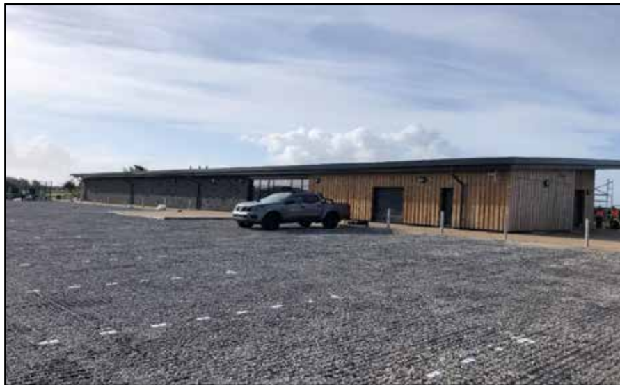
Image Two: Sports Pavilion 90% complete.
