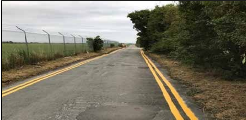
Image Three: Division Lane West pre upgrade.
