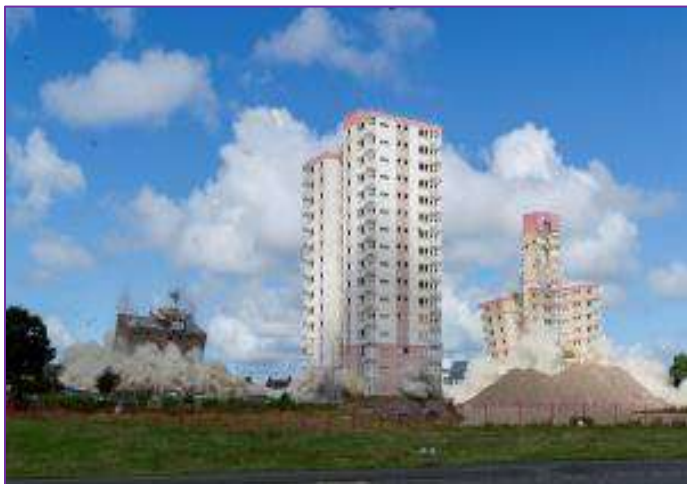
Figure 2: Queens Park demolition
