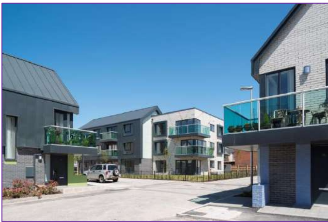
Figure 11: New family homes at Queens Park redevelopment
