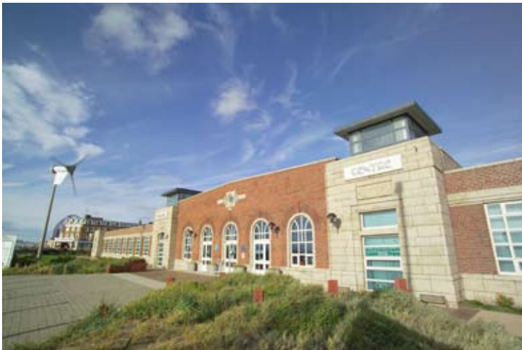
Solaris Centre, South Promenade
