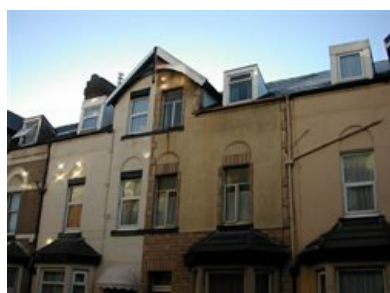
Roof dormers, different window treatments and cladding on Yorkshire Street
