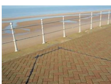
Balustrades to lower walkway
