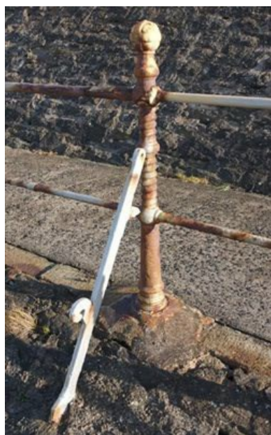
Corroding balustrade
