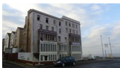
Former Ambassador Hotel viewed from Derby Road, now demolished
