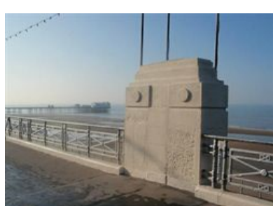
Piers and balustrades to upper walkway
