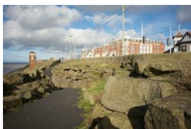
View towards cabin lift from cliff path
