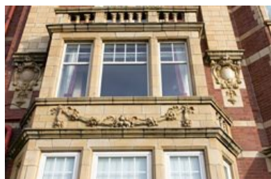
Windows with faience decoration, Cliffs Hotel
