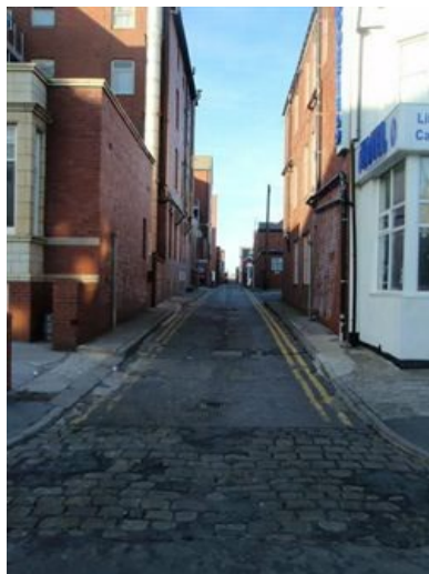
Service lane to the east of the Cliffs Hotel
