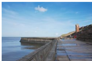
View towards Cabin lift and former boating pool along Lower Walk
