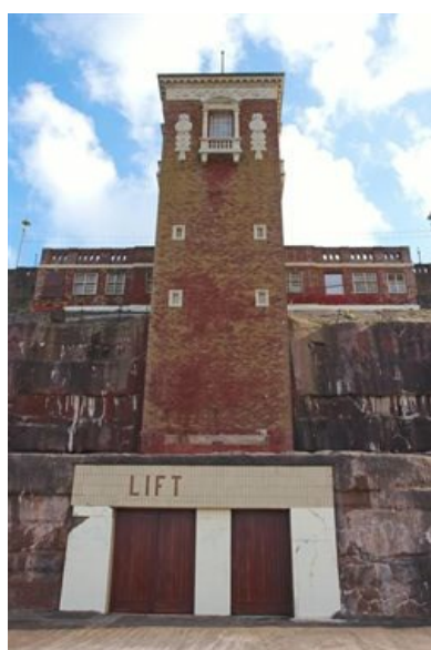
Entrance to non-functioning lift from Lower Walk
