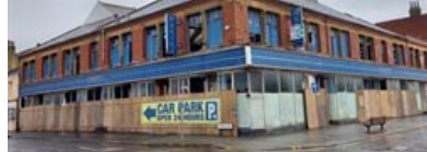
Former Woolworth's store
