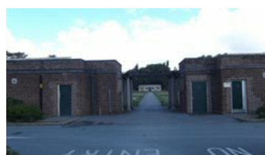
Male and female toilets at the entrance to the bowling greens
