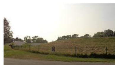
View of BMX track from East Park Drive
