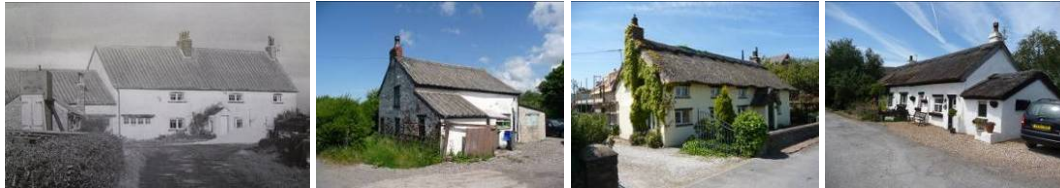
Plate 26. Early cobbled houses from left: Midgeland Farm, The Pod (?), Worthington Road, Fisher's Lane (LB).
