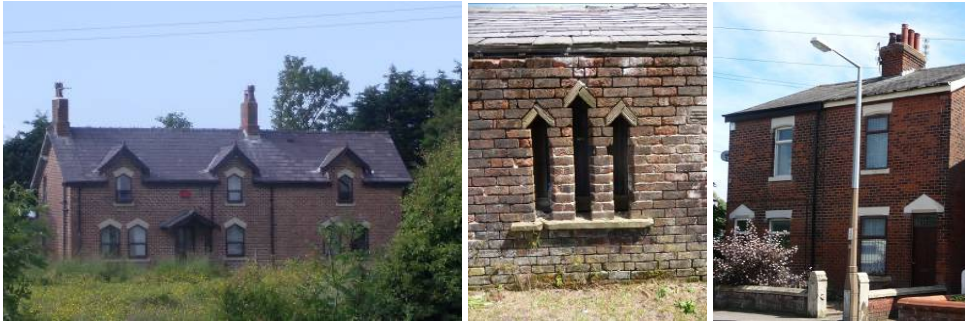
Plate 34. Triangular lintels make a brief but distinctive appearance in this character area; Rosehill Cottage on the right is only just inside character area 2.
