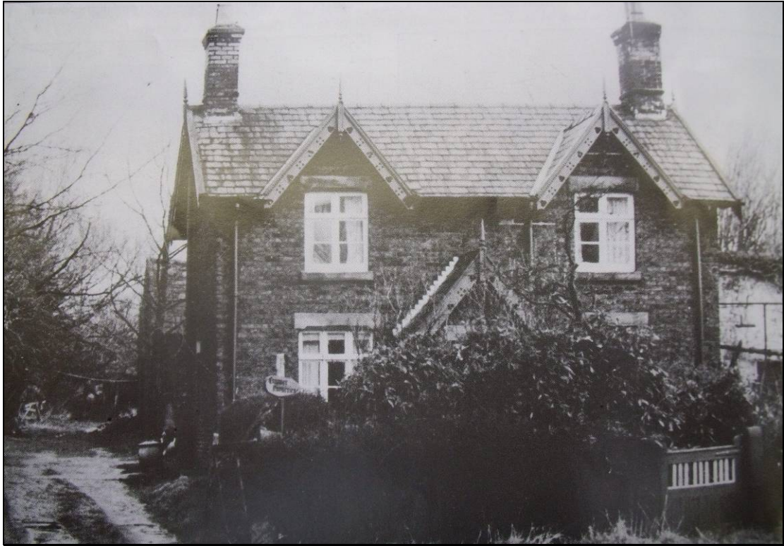
Plate 17. Cropper Road nurseries built in 1872 and now demolished to make way for the Peel Road industrial estate. The use of decorated bargeboards on the side elevations, the dormers and the central porch, plus the pinnacles on each gable and tall chimneys heightened the house to create an airier more spacious cottage than the earlier cobbles cottages.
