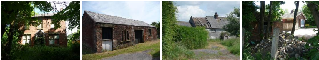
Plate 42. Buildings under threat: Worther House off Division Lane (left) the barn on Moss House Road, Midgeland Farm and an ominous pile of cobbles next to a new house on Ecclesgate Lane and a brick cart shed – was this one that got away?
