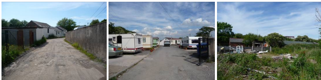
Plate 44. Unsympathetic boundary treatment, poor landscaping and a lack of maintenance have introduced a feeling of neglect around Whalley and Lilac Farms
