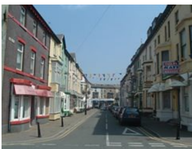
Modern fixed blinds on historic buildings.
