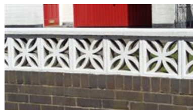
Modern decorative concrete block walling.
