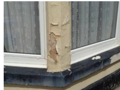
Modern paint traps water which freezes in the stone causing it to crack and flake away.
