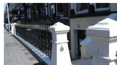
Wrought iron railings on Adelaide Street.
