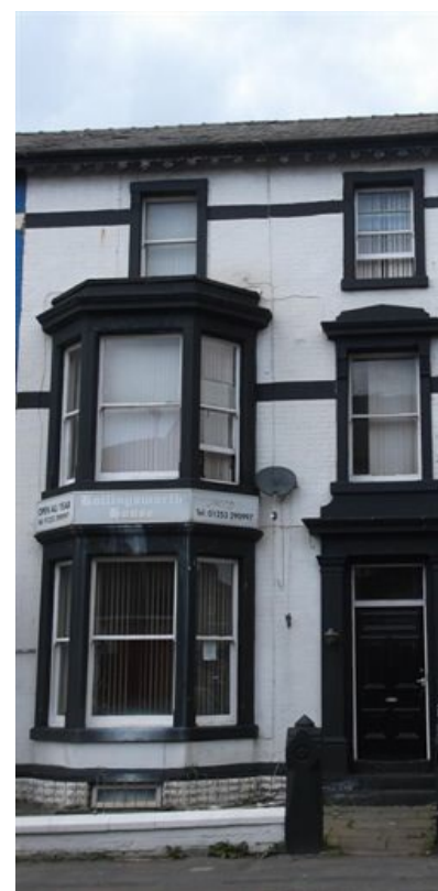
Guest house with original sliding sashes.
