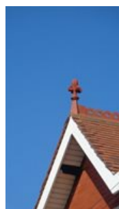
Terracotta finial and ridge cresting.
