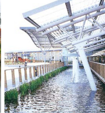
(c) Roof water is directed into this storage pond which serves as an attractive feature of Wheatley Services Area on the M40
