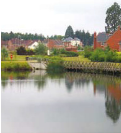
(b) Ponds and wetlands are typically fitted as the final stage of a SUDS system for a major development
