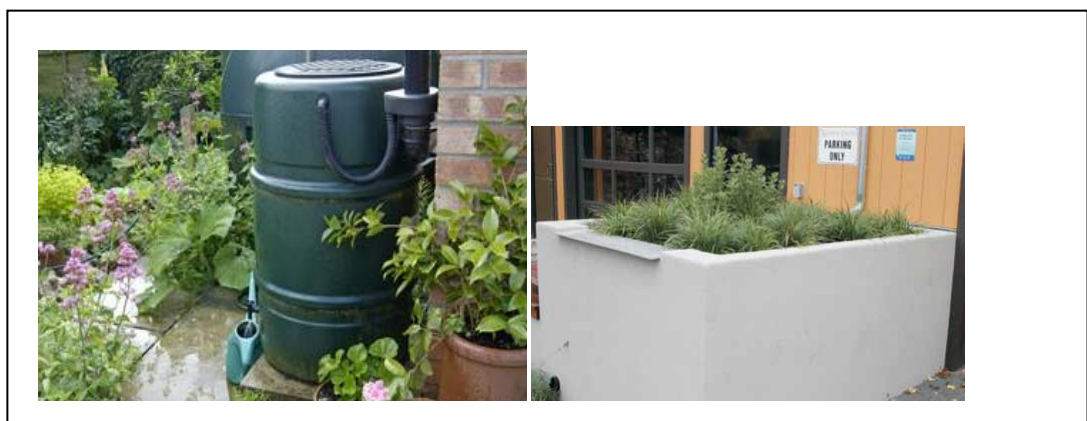
Figure 2-9 Examples of water butts and disconnection planters
