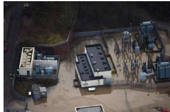
Flooded power station at Lancaster in December 2015
