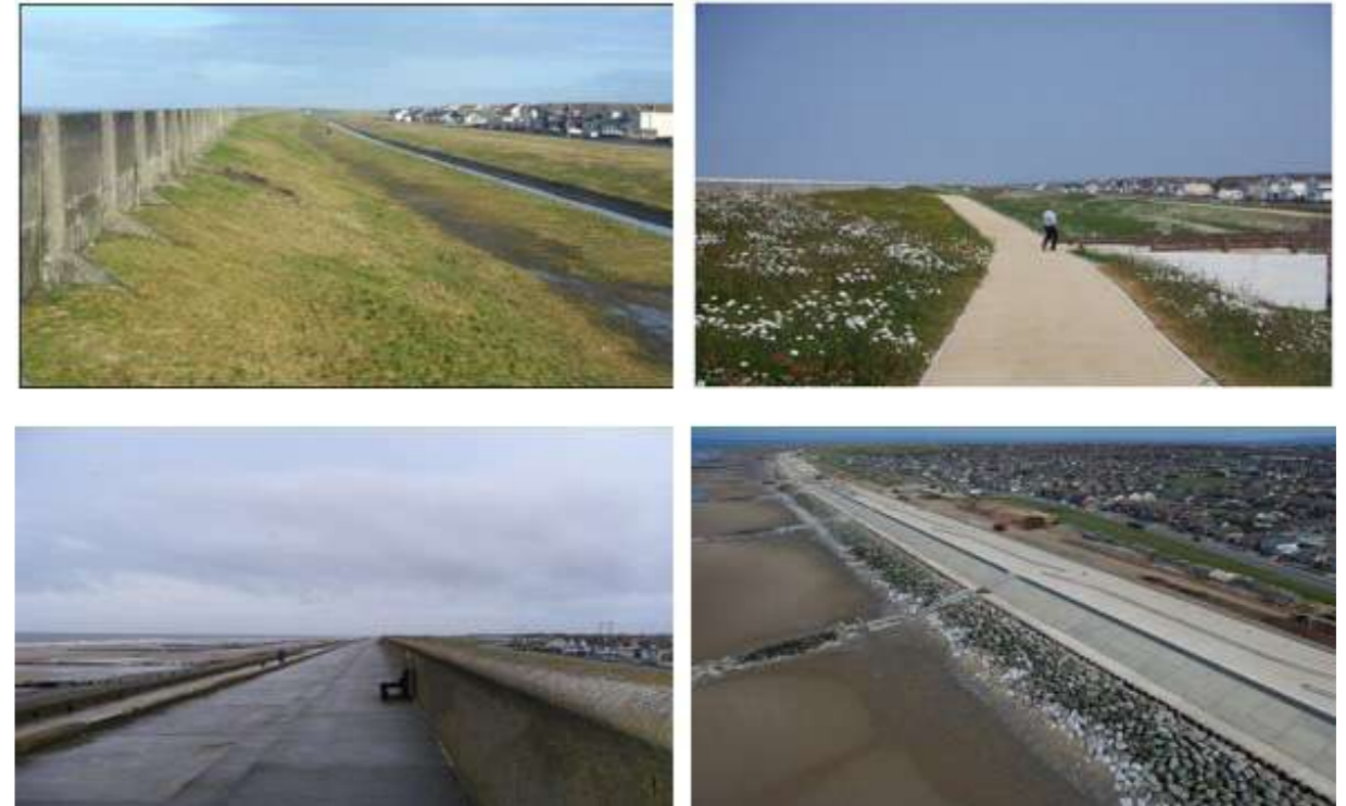
Figure 13: Rossall Coastal Defences Before & After
