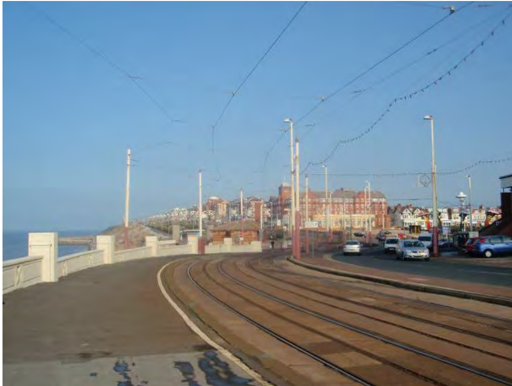
Fig. 12: View north towards Gynn Square
