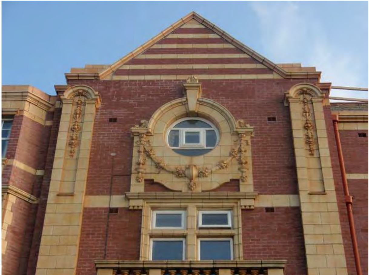
Fig. 18: Yellow terracotta faience details to the Cliffs Hotel
