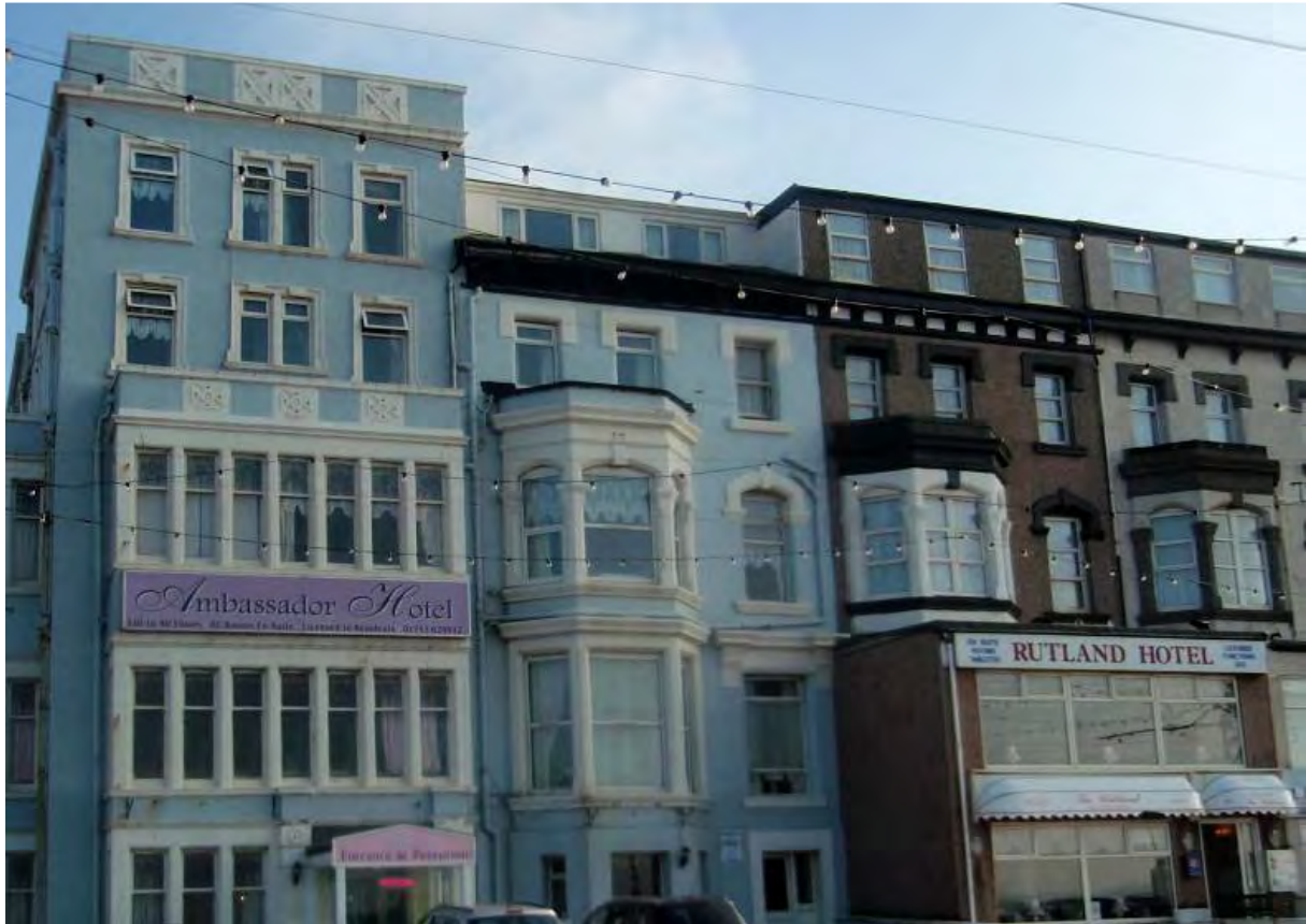
Fig. 19: Sash windows to the square bays of the Ambassador Hotel, and unsympathetic uPVC replacements in the neighbouring building
