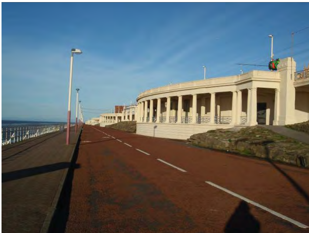
Fig. 13: Looking north along the lower walkway
