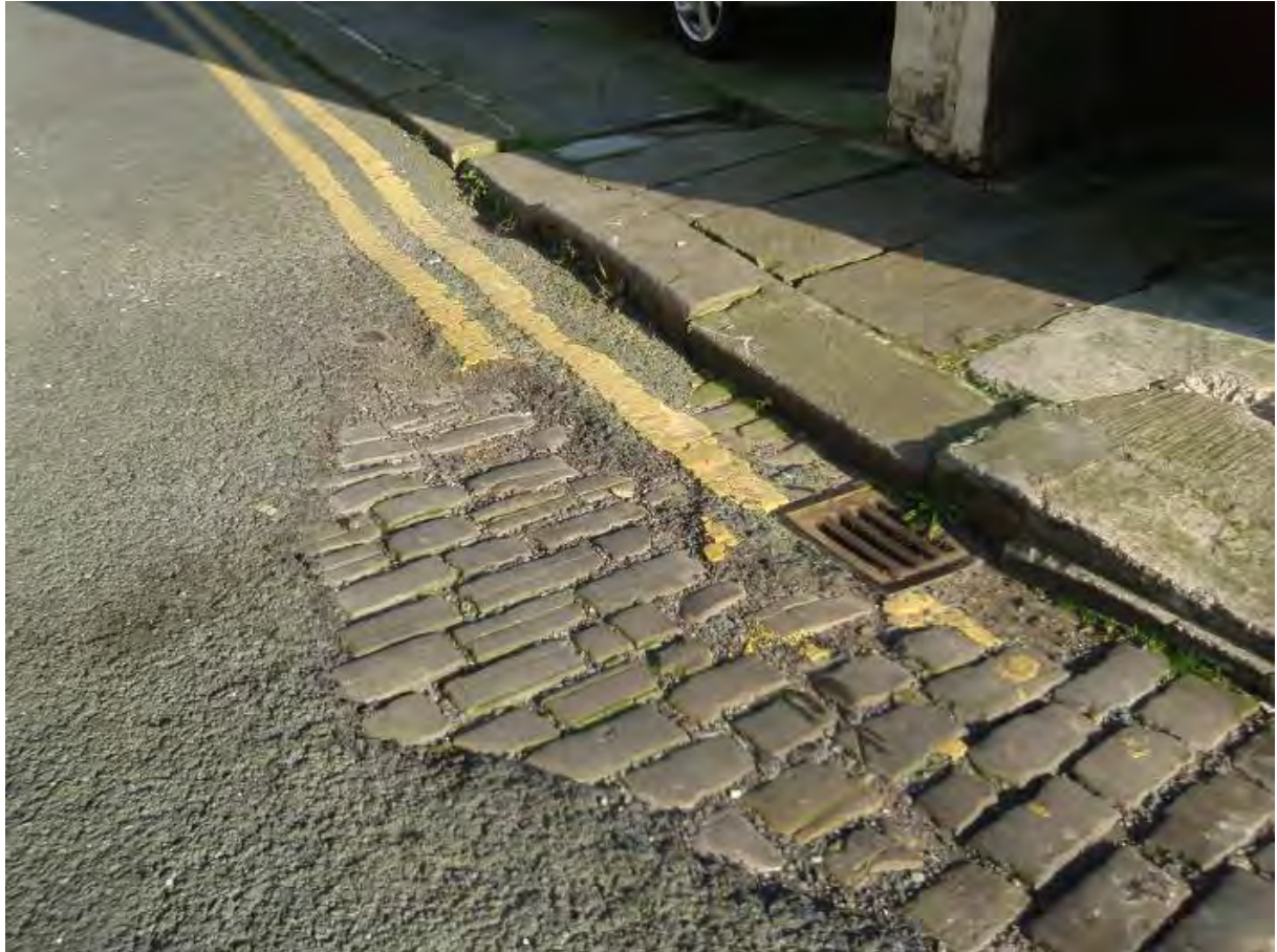
Fig. 28: Exposed stone setts on Banks Street
