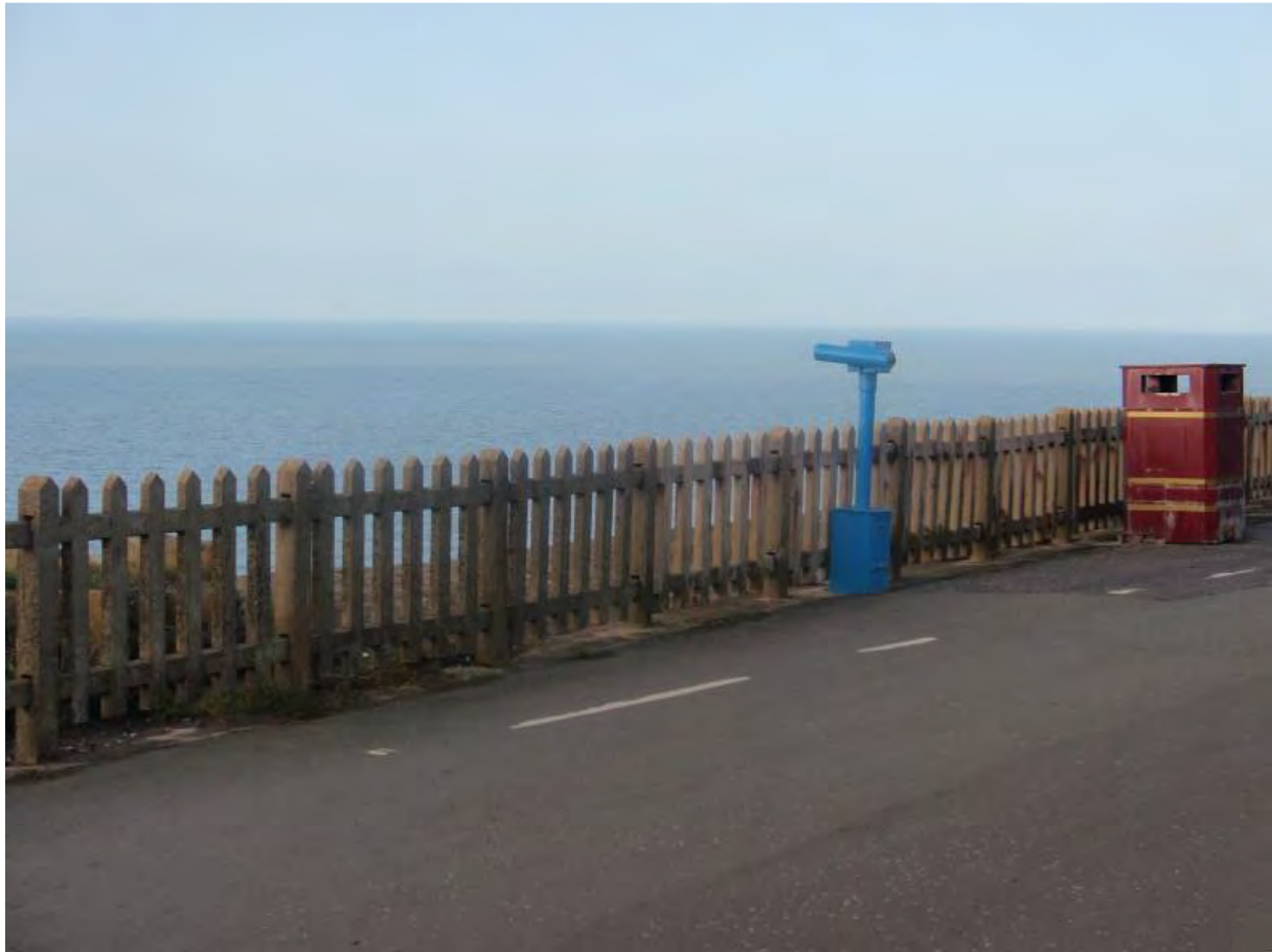
Fig. 25: Concrete fence at north of Promenade
