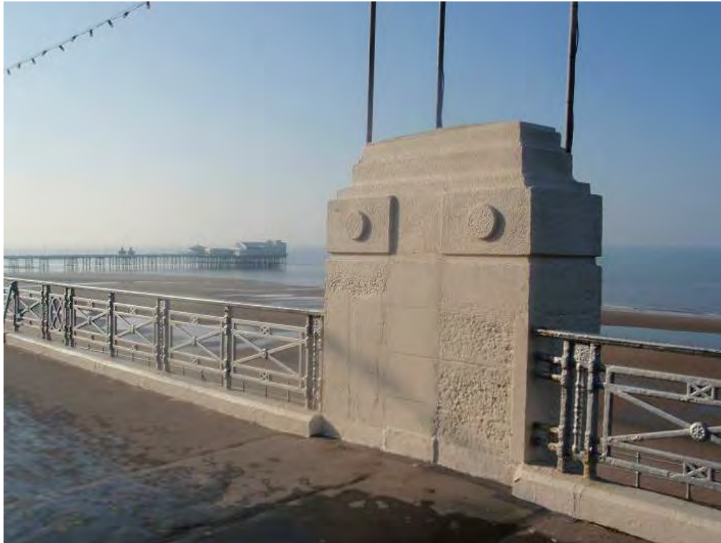
Fig. 23: Piers and balustrades to upper walkway
