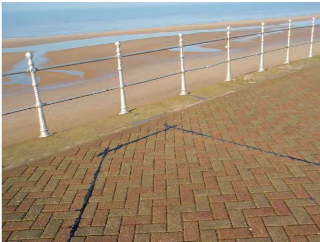
Fig. 24: Balustrades to lower walkway
