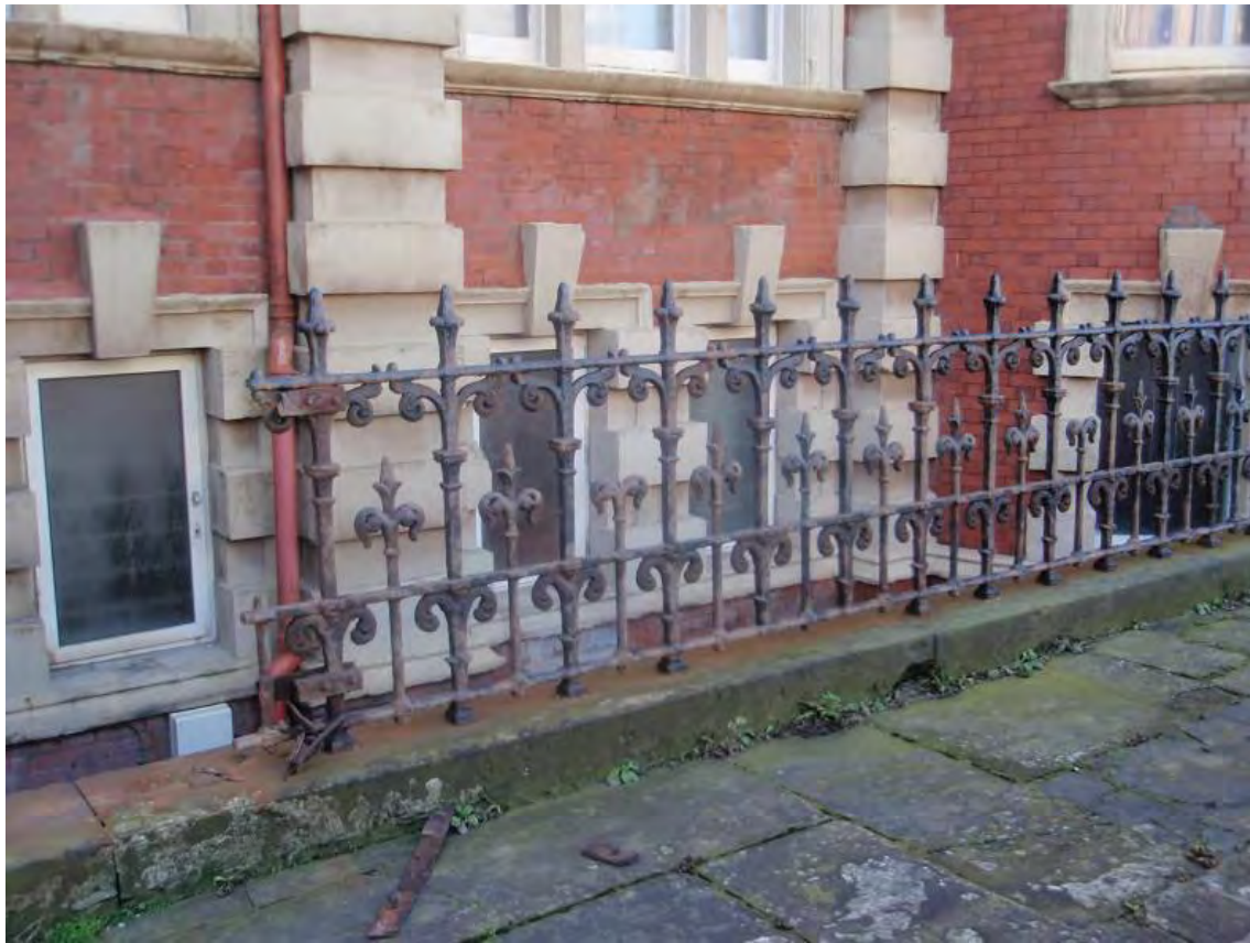
Fig. 26: Cast-iron railings at rear of the Imperial
