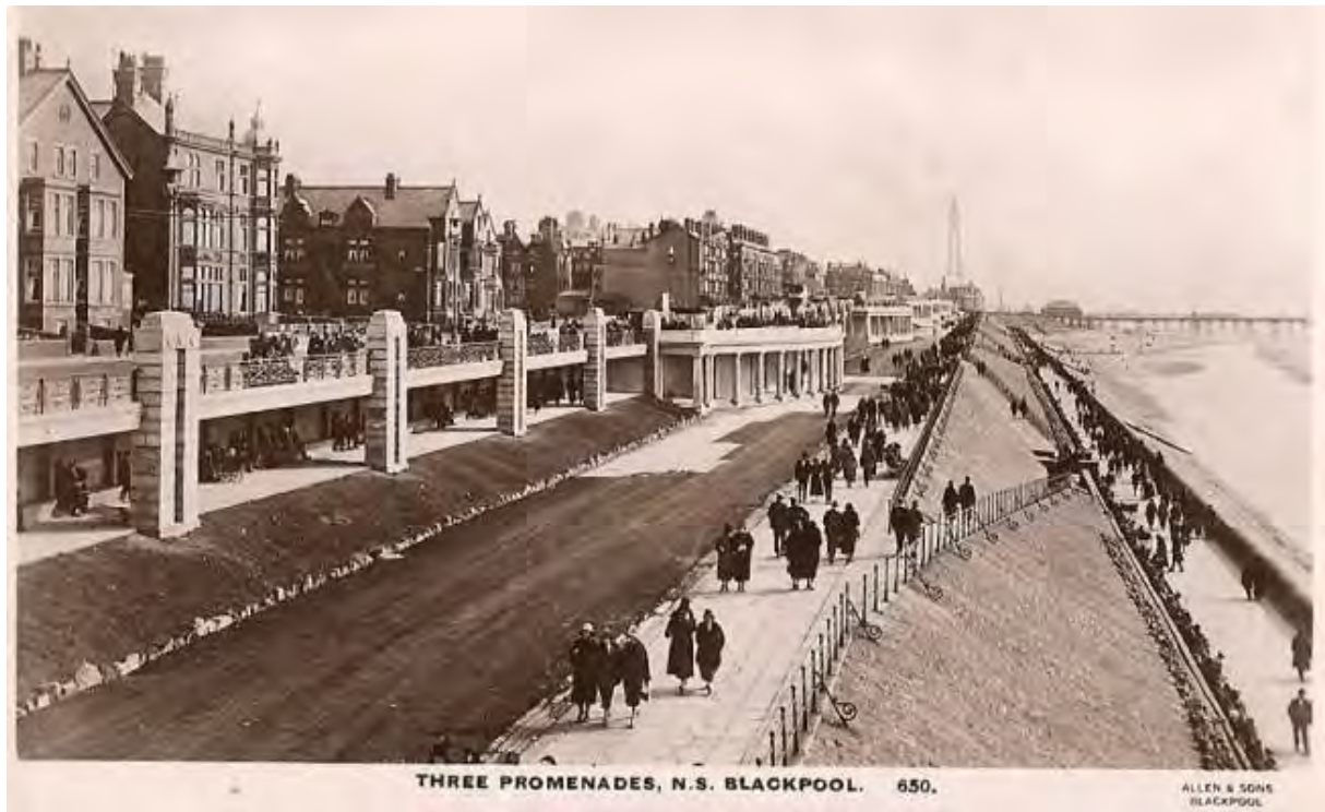
Fig.9: The Lower Walk, Middle Walk with colonnades, and the upper promenade (Queen's Drive), North Promenade, c.1920 (Image from www.rossallbeach.co.uk )
