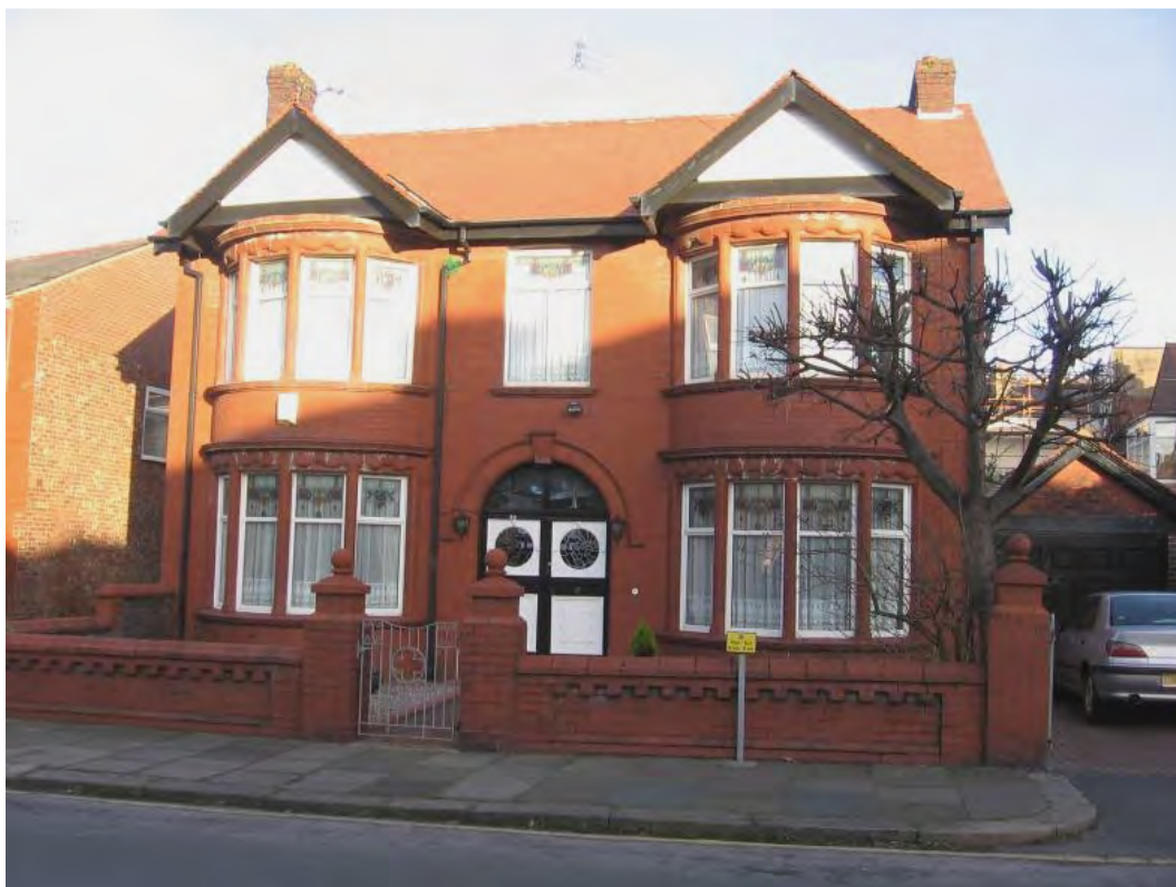
Fig. 85: Nos. 29-31 Leicester Road: intact houses with possibly contemporary garage
