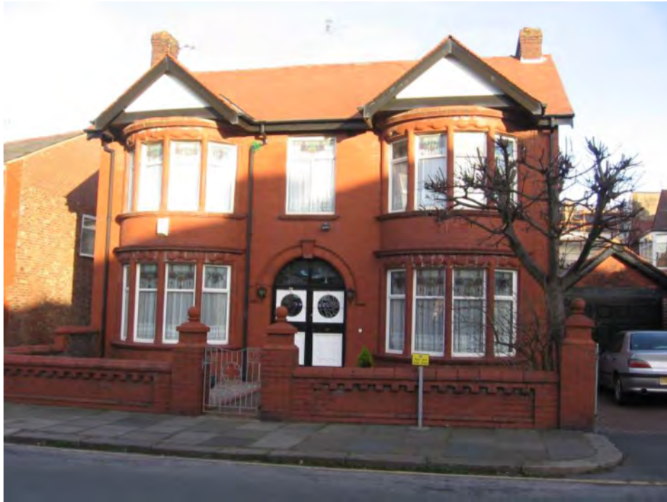
Fig. 44: Boundary walls, piers and gatepiers, Nos. 29-31 Leicester Road
