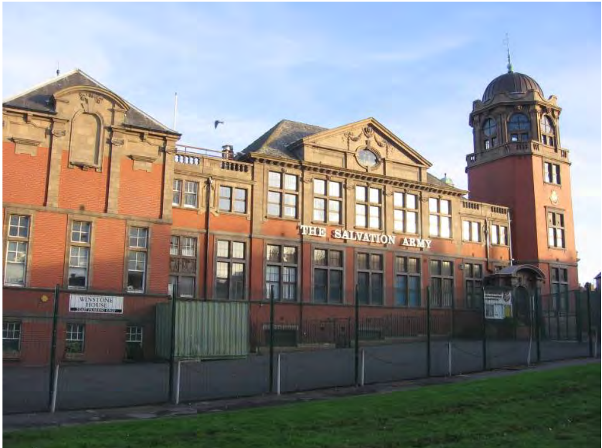
Fig. 64: The former Grammar School from the west
