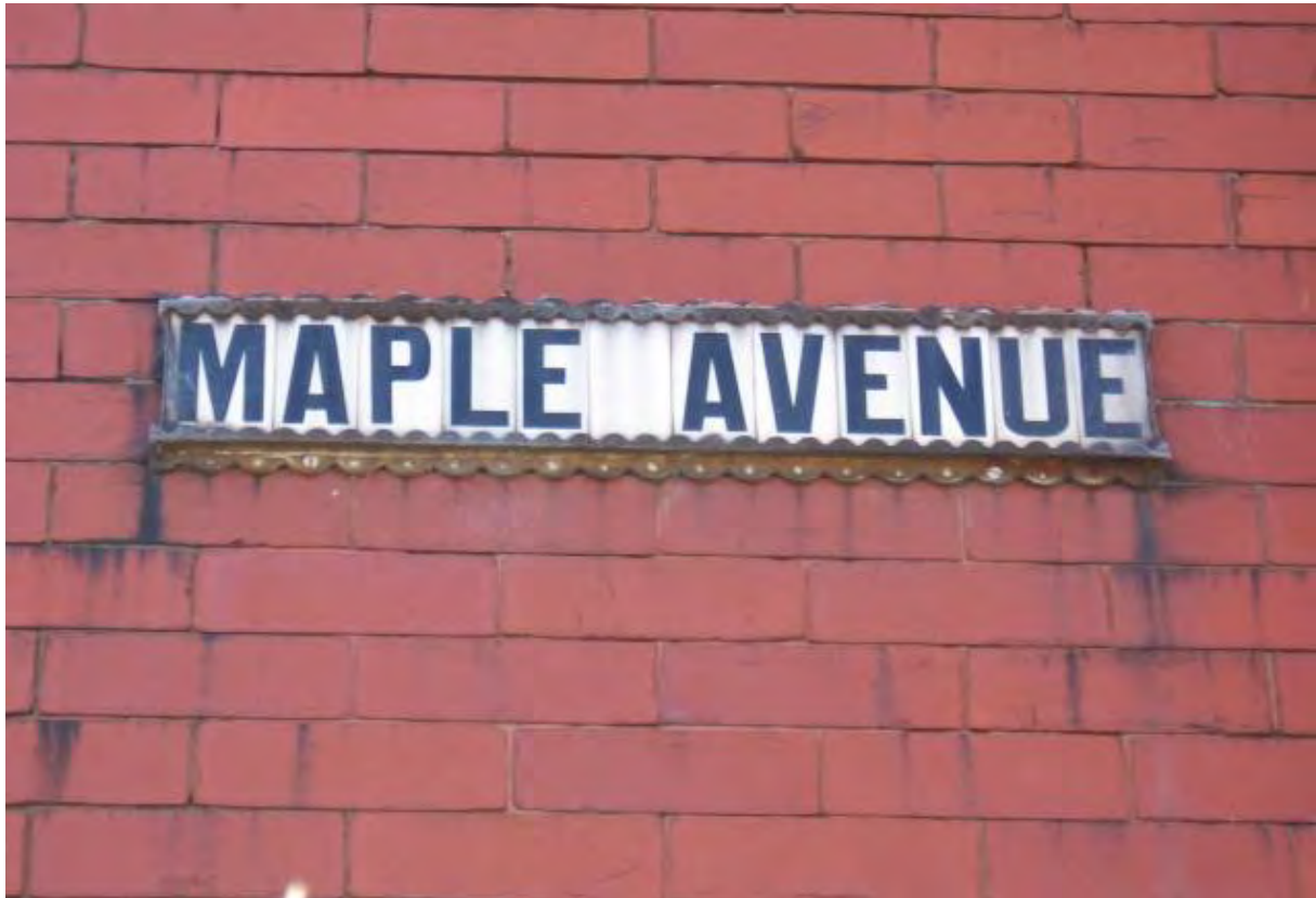
Fig. 102: Typical cast iron and tiled street sign
