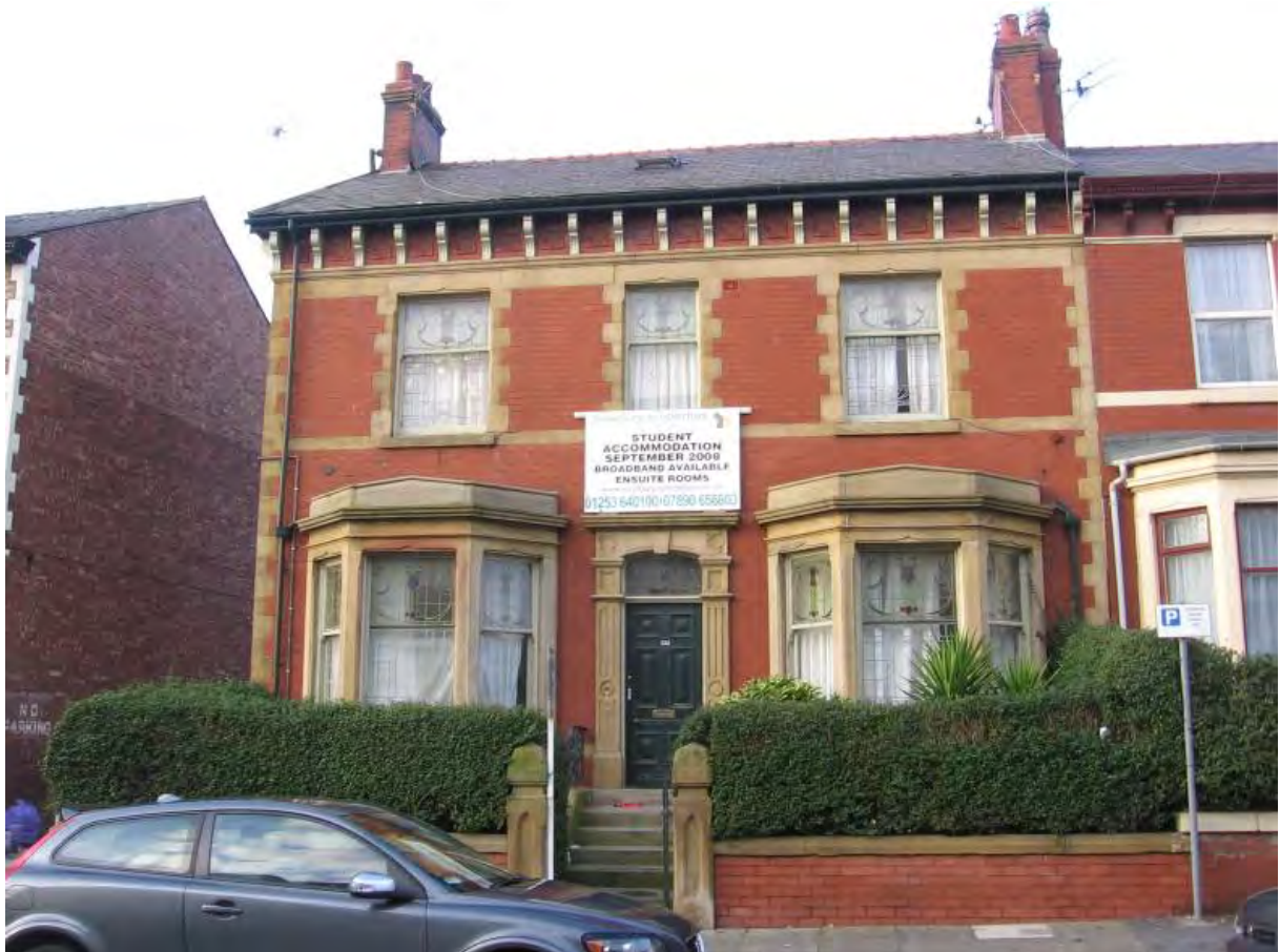
Fig. 31: Bay windows and stone dressings: Palatine Road
