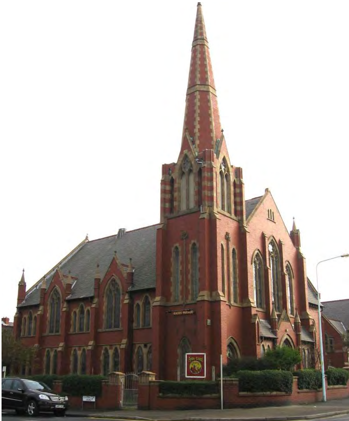
Fig. 60: Former Methodist Church
