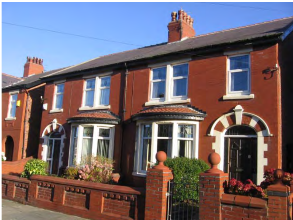
Fig. 45: Intact decorative brick boundary walls and gatepiers with terracotta details, Longton Road.
