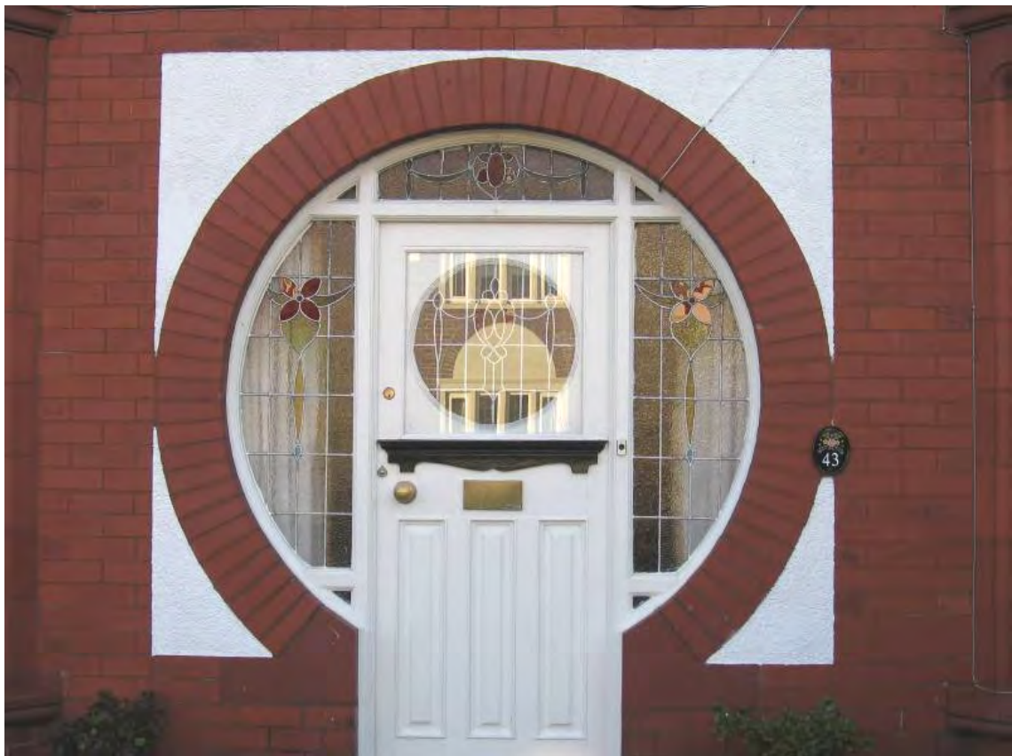
Fig. 94: Unaltered doorway at No 43
