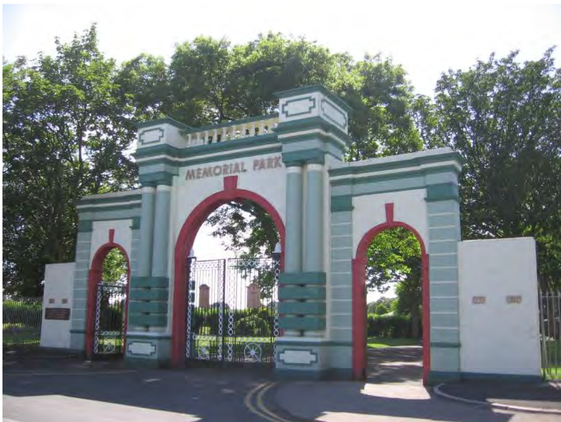
Fig. 11: Part of the screen from Raikes Hall pleasure gardens at Fleetwood Memorial Park.
