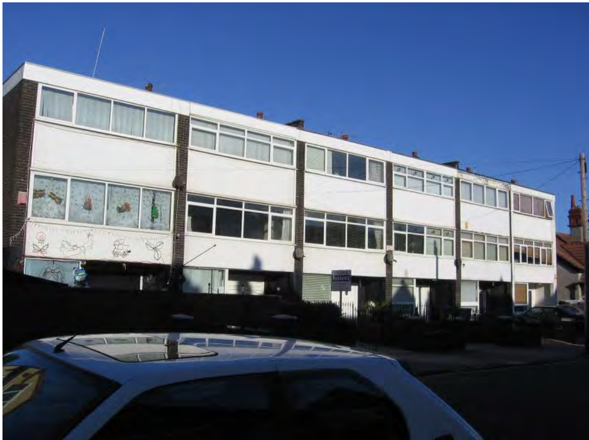
Fig. 77: Flats, Nos. 153-163 Read's Avenue
