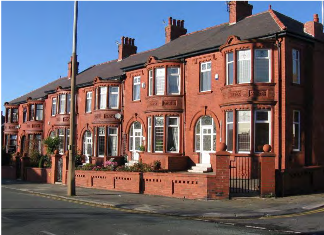
Fig. 109: Little altered, well-detailed terrace (Nos. 32-40) on the north side, built 1920s
