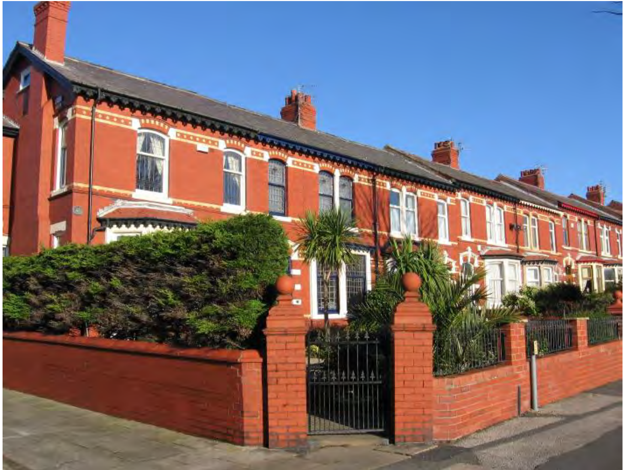
Fig. 113: Little altered terraces and garden walls (Nos. 30-60), north side
