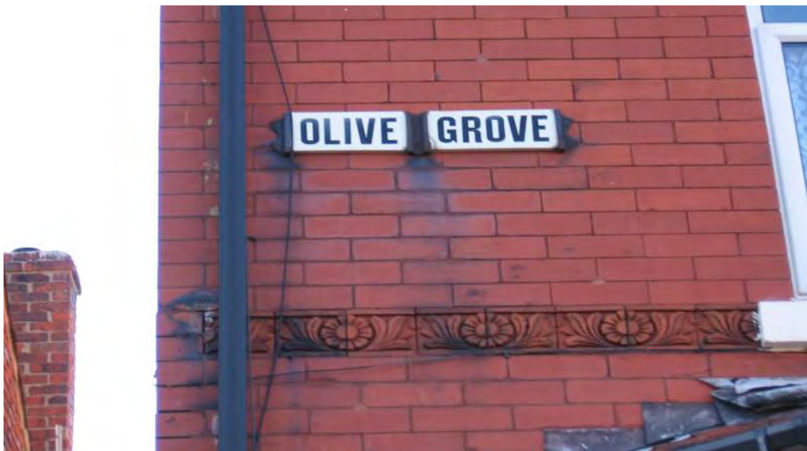
Fig. 105: Cast iron and ceramic street sign on a terraced house
