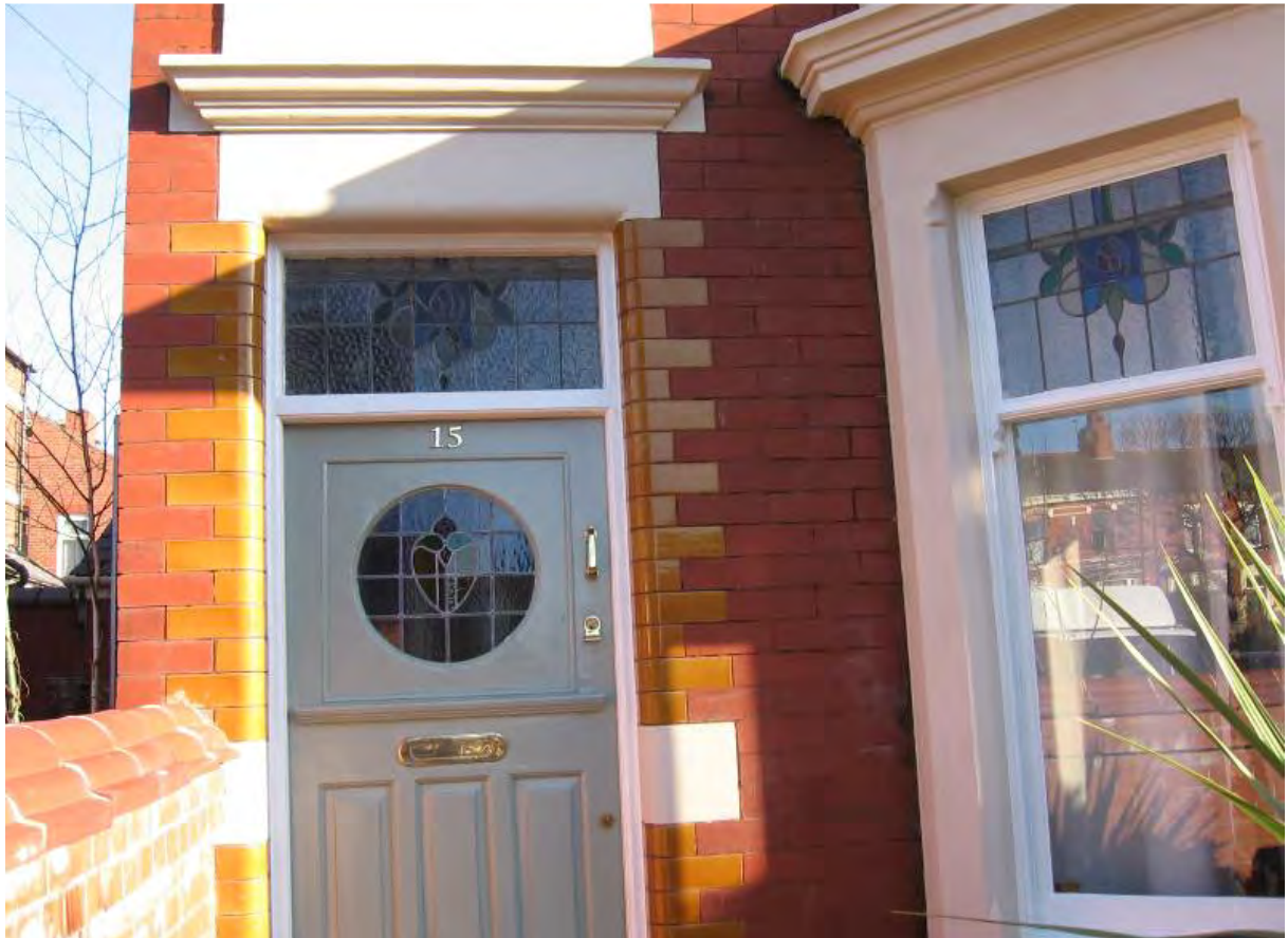
Fig. 34: Modest example of intact joinery with sash, door with overlight at Elm Avenue, early 1900s
