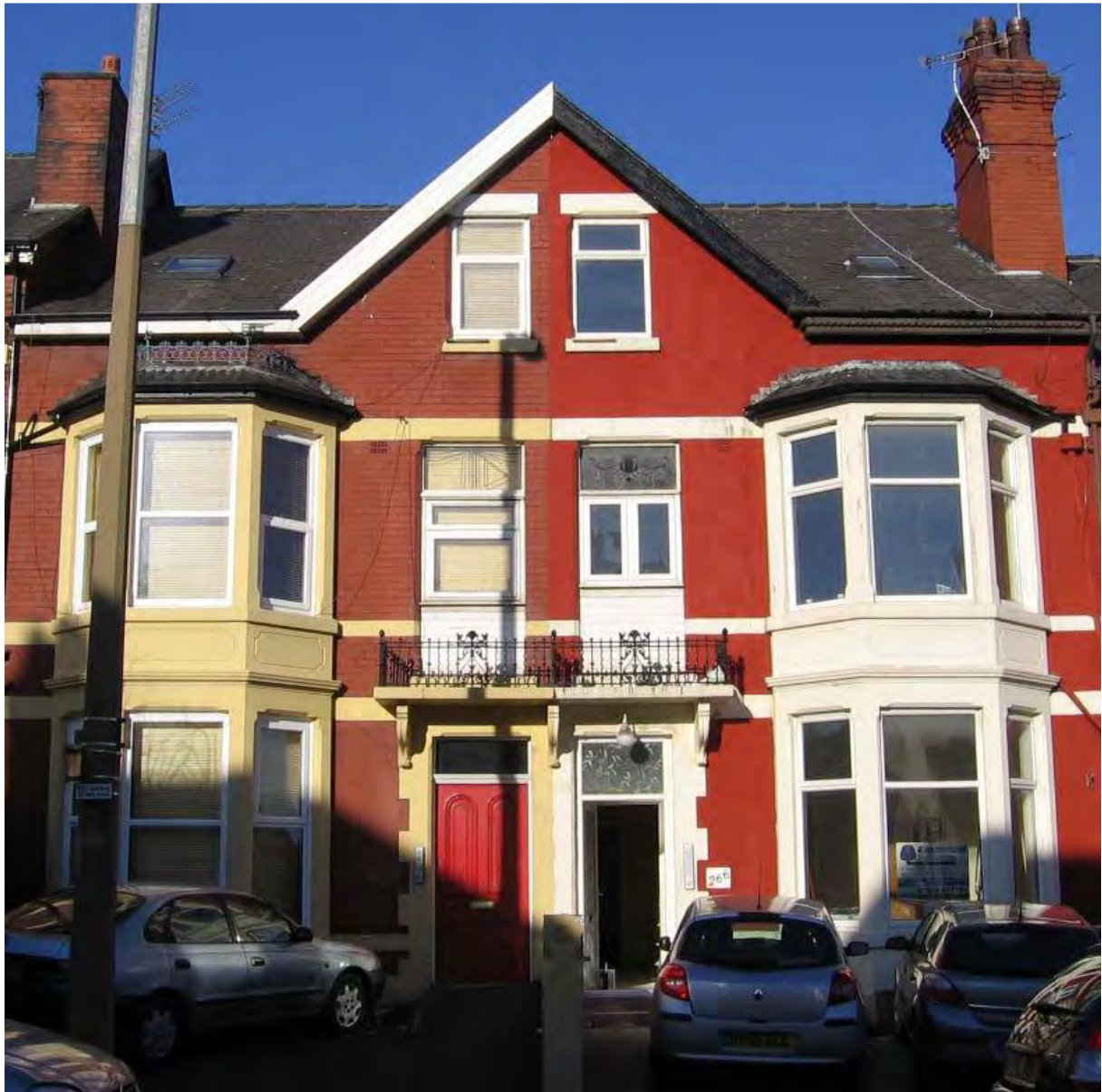
Fig. 43: Ironwork balconies and bay cresting (left) on Hornby Road
