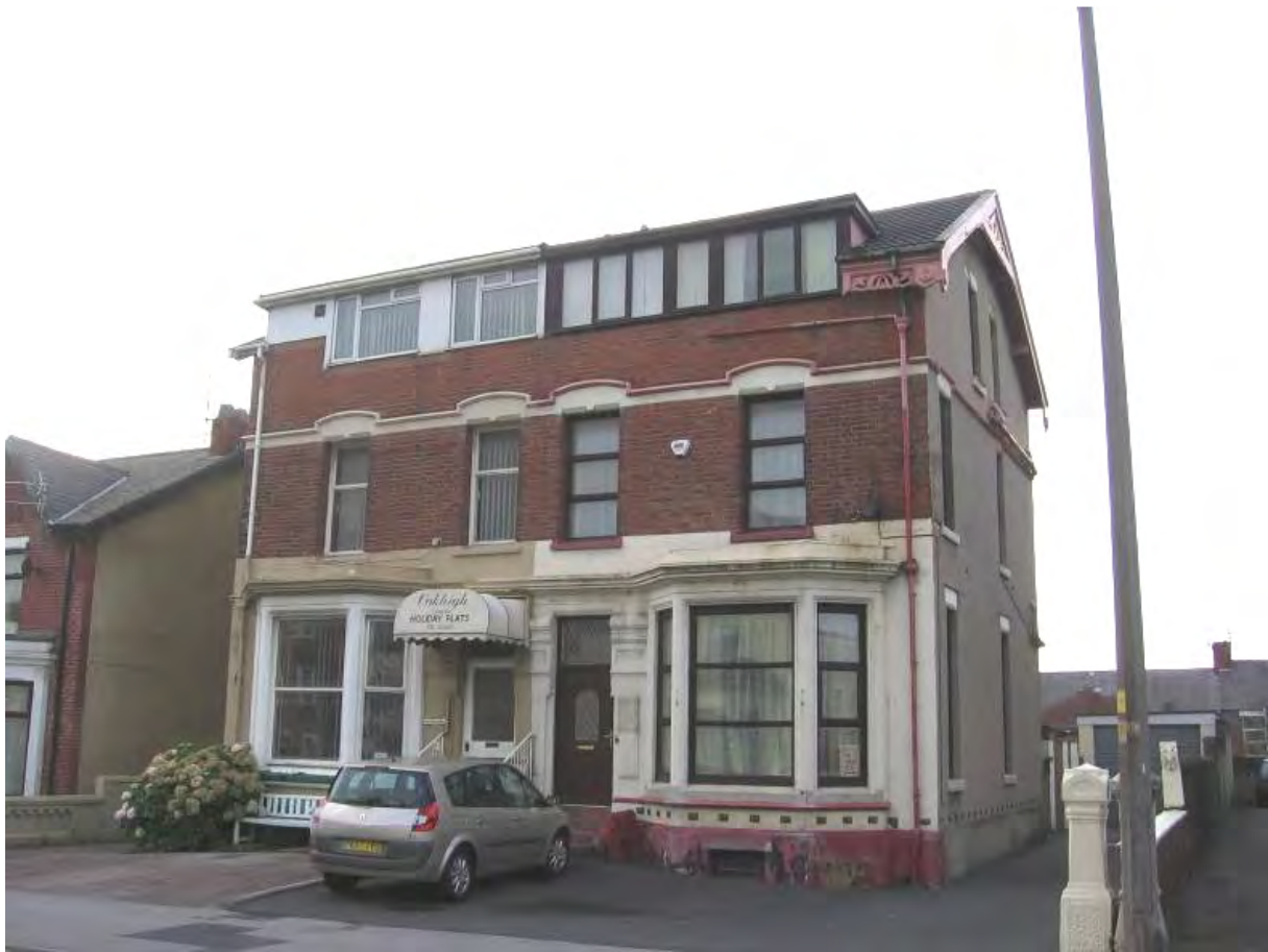
Fig. 66: Unsympathetic alterations and frontage parking: Nos 51-53 Park Road
