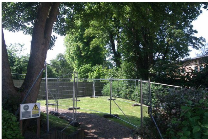
Figure 7: Acceptable tree protection with correctly placed heras fencing and clear signage.
